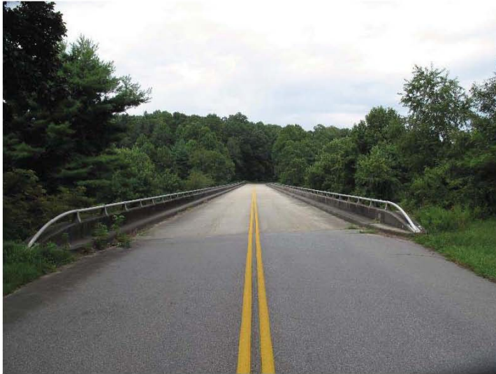
PHOTO #1 - LOOKING SOUTHBOUND TOWARD CHEROKEE
