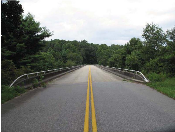
PHOTO #1 - LOOKING SOUTHBOUND TOWARD CHEROKEE
