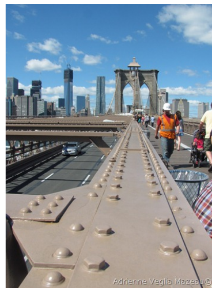
Pedestrian and bicycle bridge above the Brooklyn Bridge, New York City, NY
