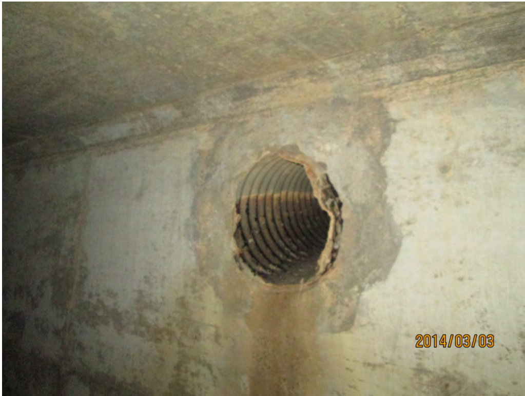
Pipe Outlet in the Middle of the Box
