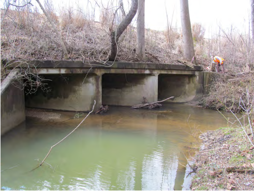
Looking at Upstream Face of 3 @ 7' x 7' RCBC under I-26
