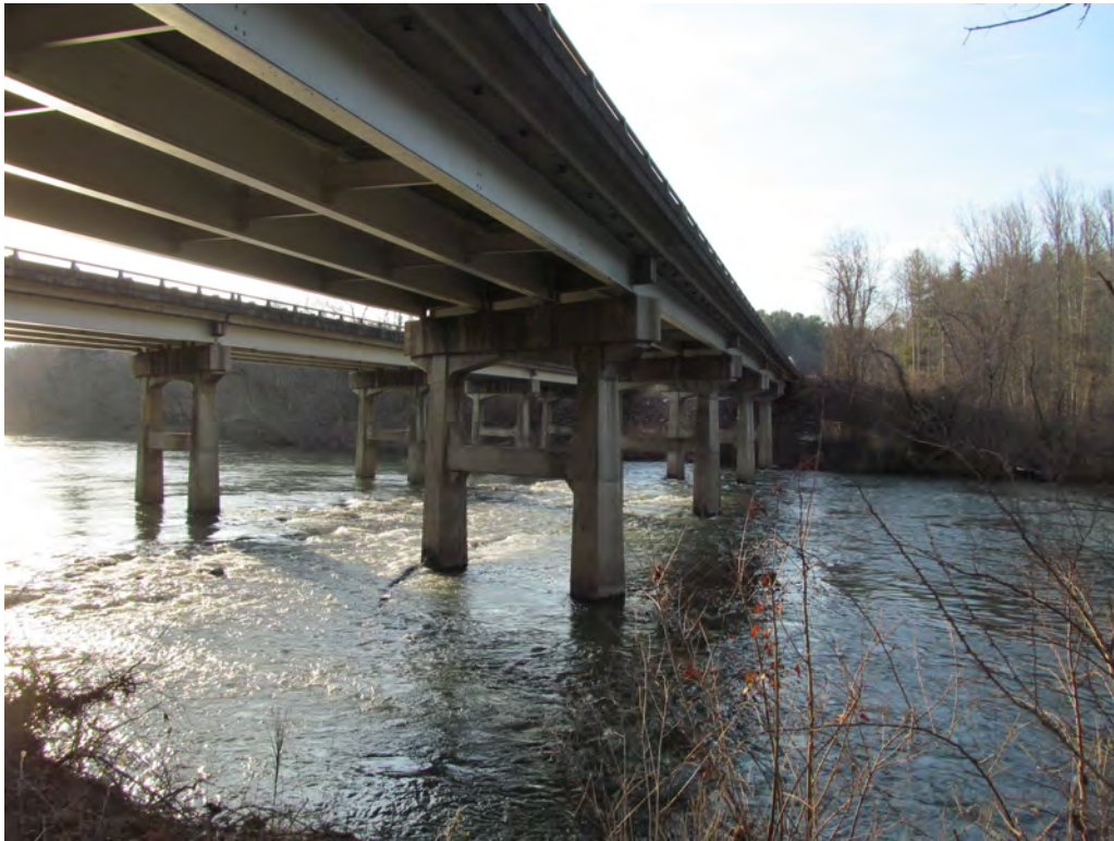
Looking at Downstream Face
