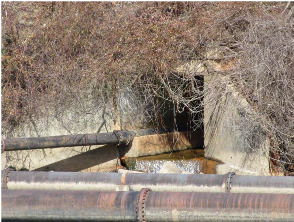
Looking at Downstream Face of 1 @ 8' x 8' RCBC under I-26
