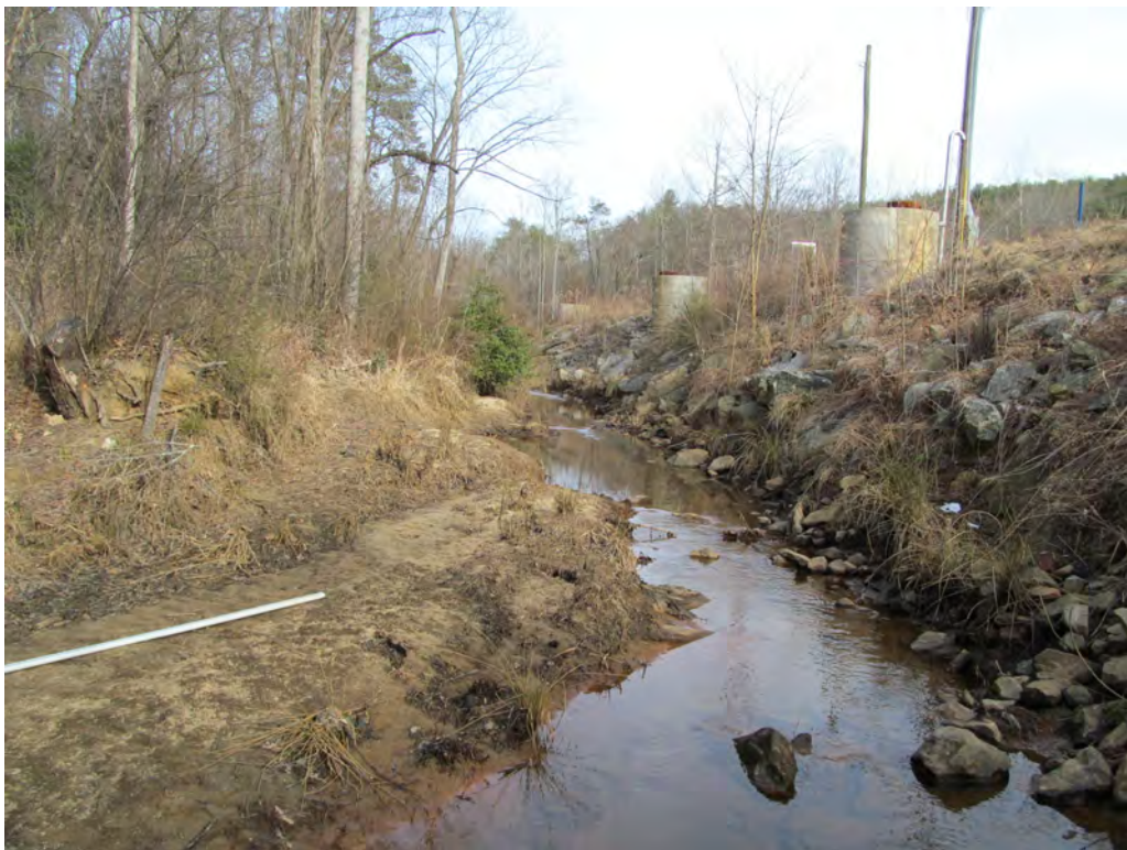
Looking Upstream from 2 @ 10' x 10' RCBC Inlet
