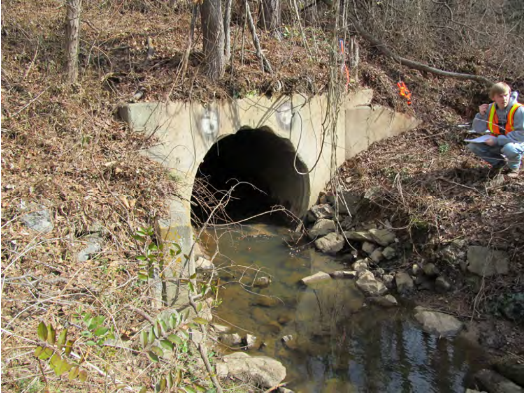
Looking at Upstream Face of 66" SPP with Headwall under I-26
