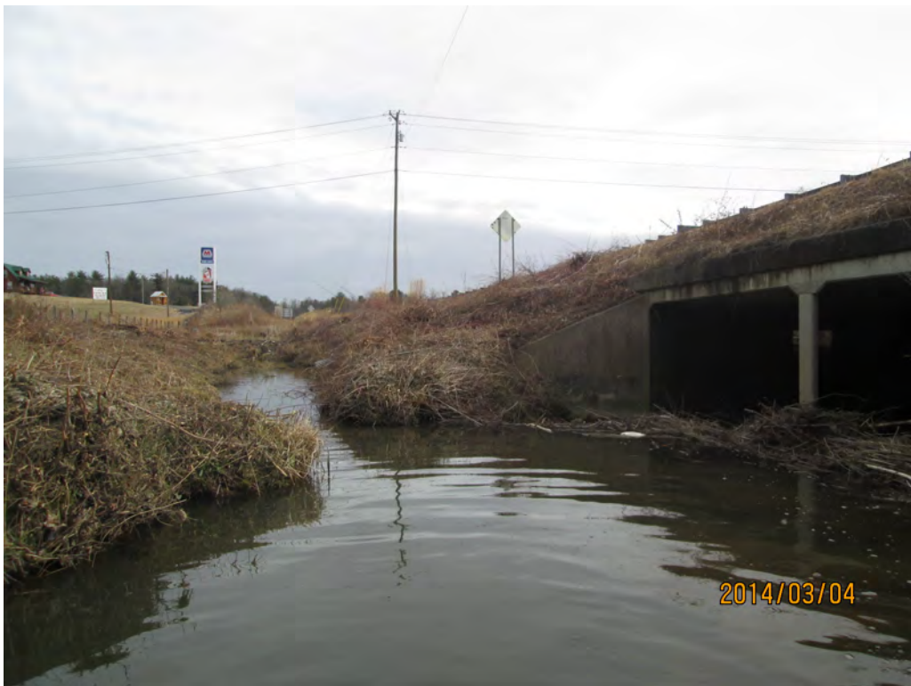
Looking at Upstream Left Ditch
