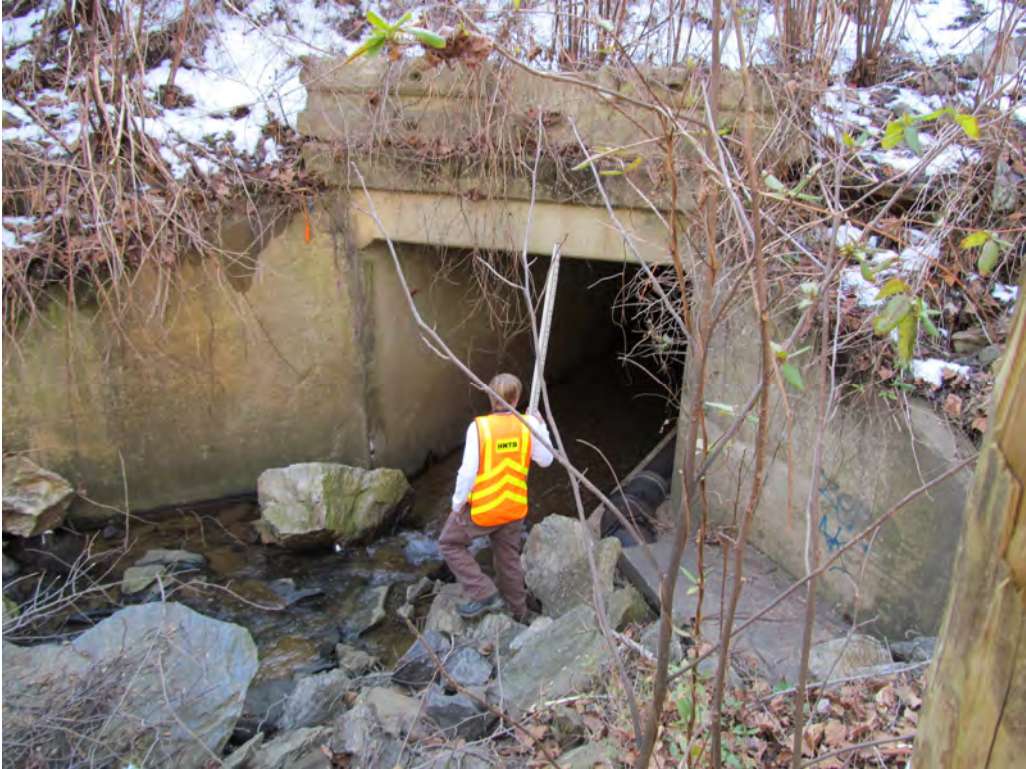
Looking at Upstream Face of 1 @ 8' x 8' RCBC under I-26
