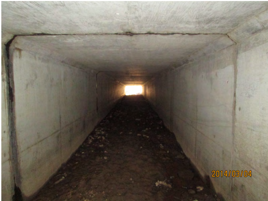
Looking Downstream in Right Barrel
