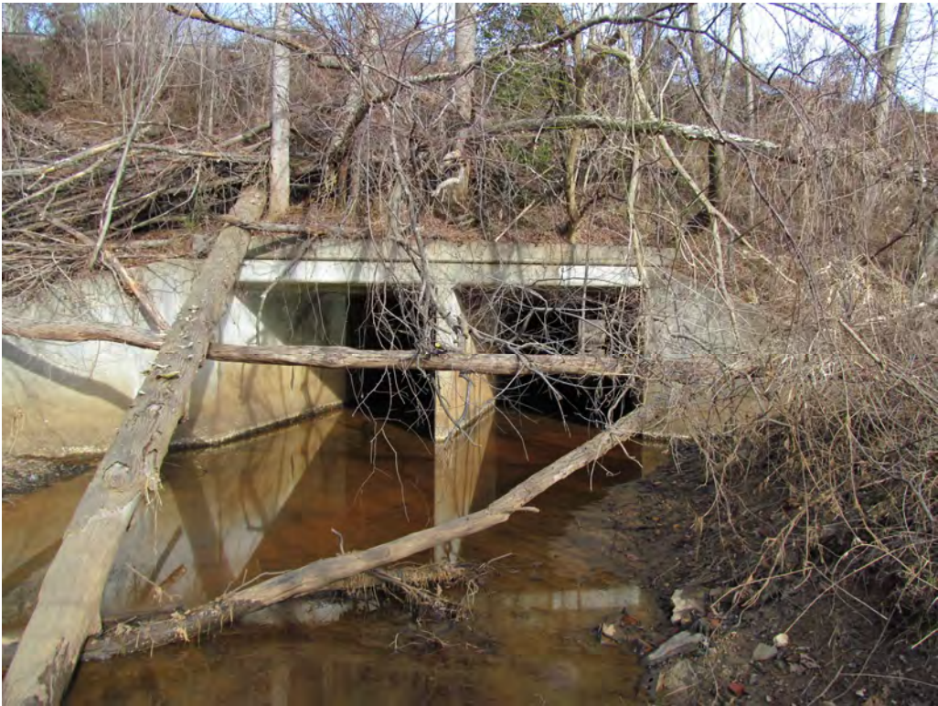
Looking at Downstream Face of 2 @ 10' x 10' RCBC under I-26
