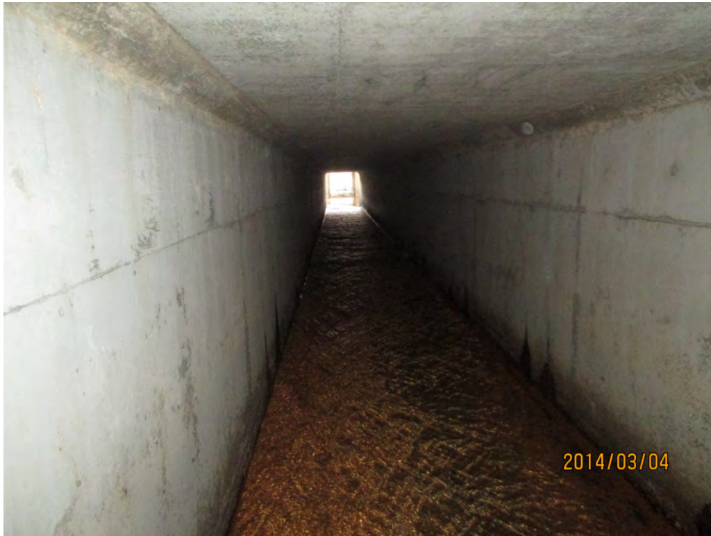
Looking Downstream Inside of 1 @ 6' x 6' RCBC
