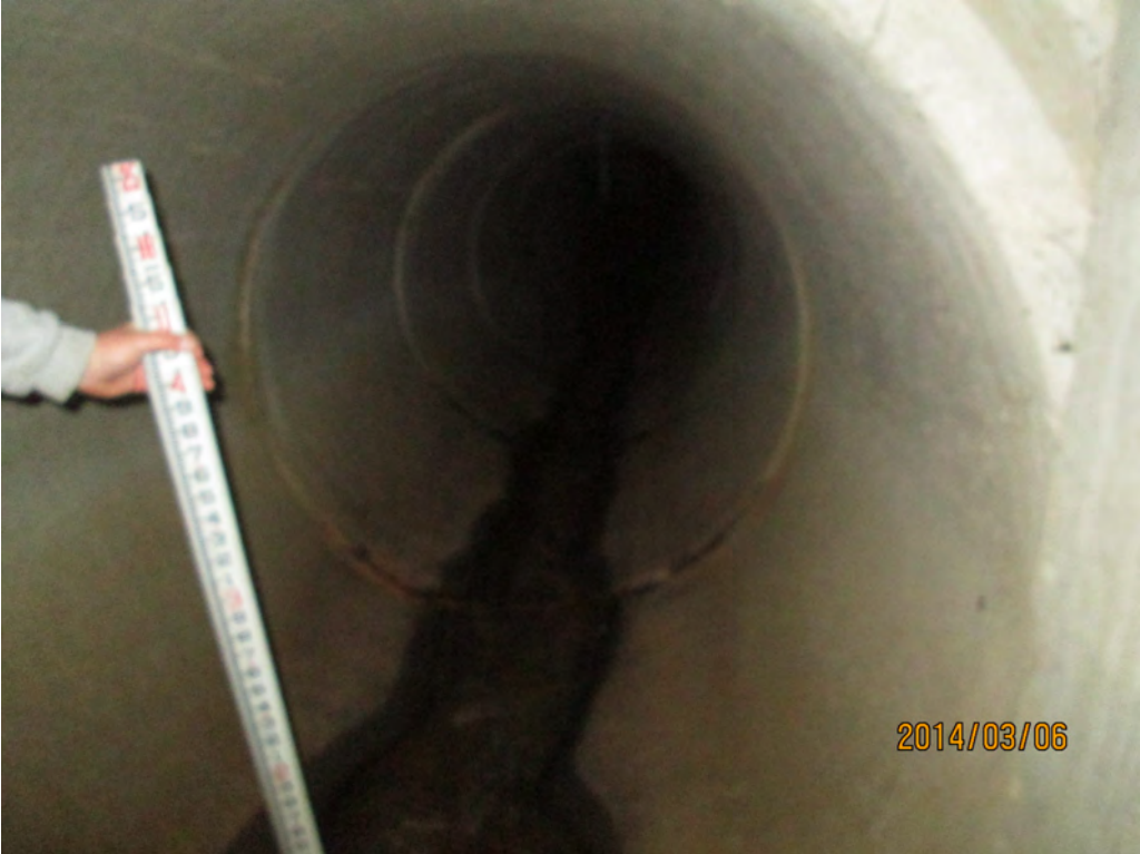
Looking Downstream Inside of 66" RCP
