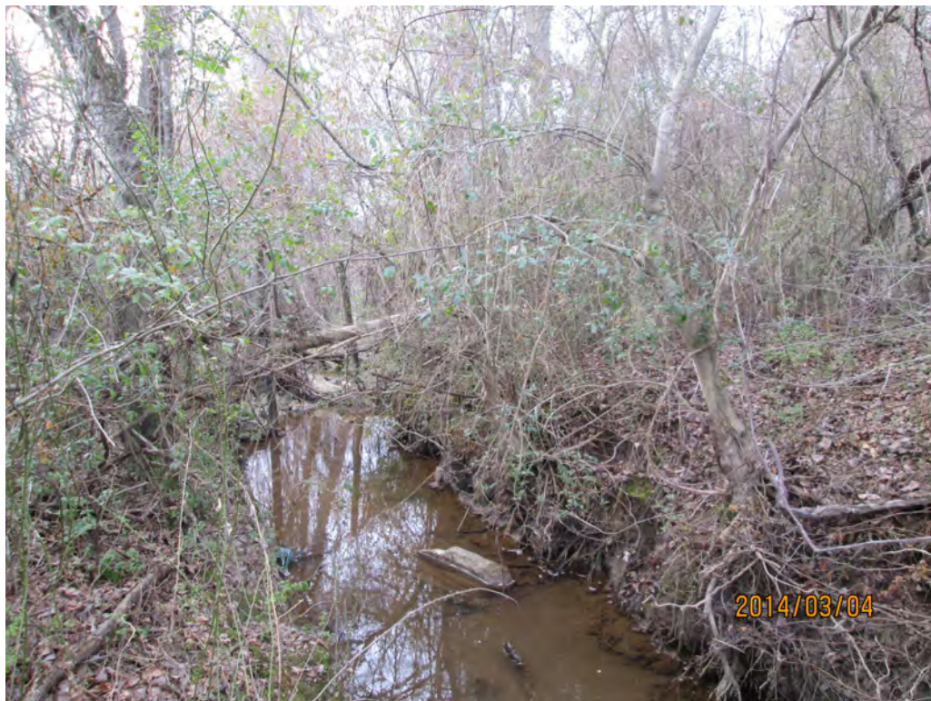
Looking Downstream from 1 @ 6' x 6' RCBC Outlet
