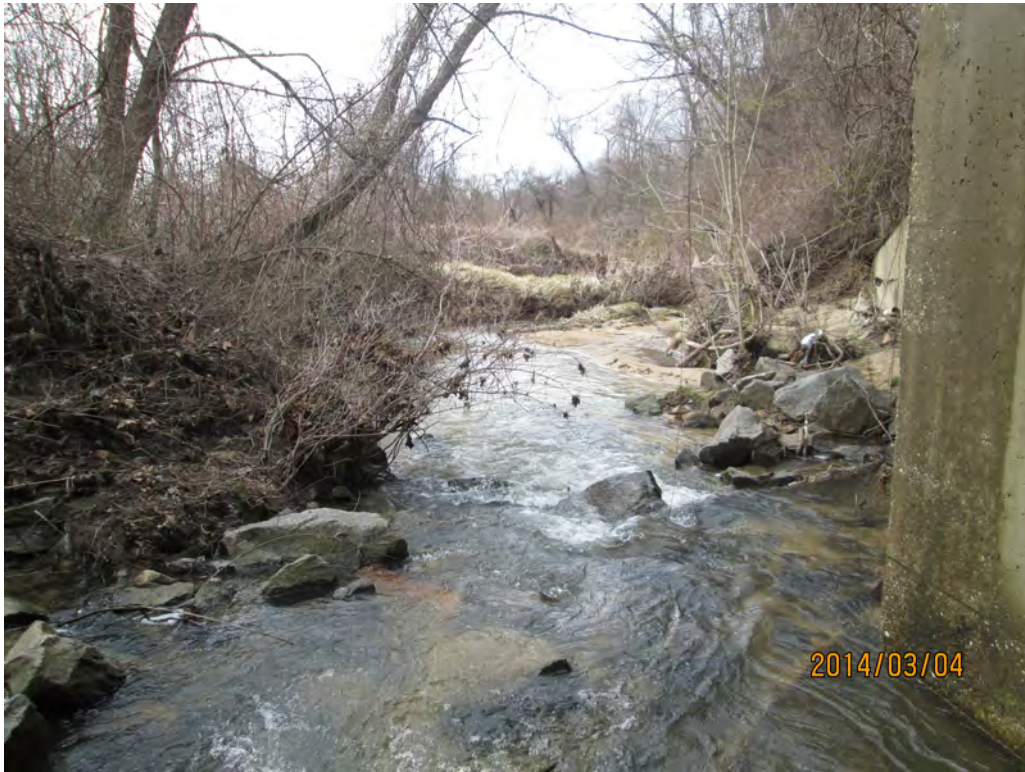
Looking Downstream from 3 @ 9' x 10' RCBC Outlet
