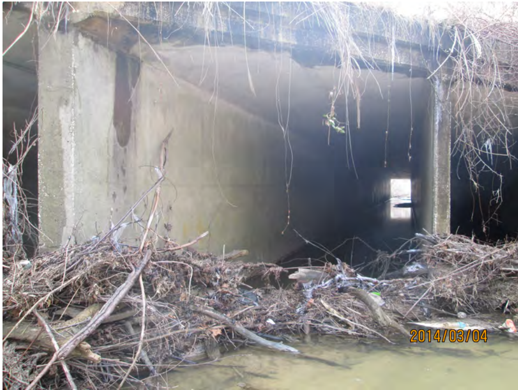
Looking Downstream in Center Barrel
