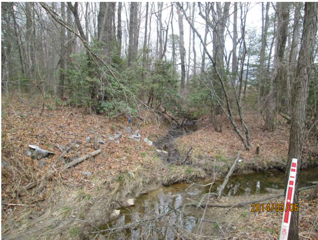
Looking Upstream from 1 @ 6' x 5' RCBC Inlet
