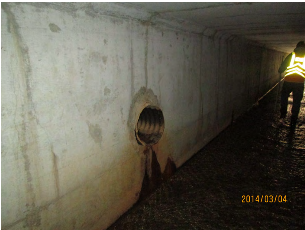
Pipe Outlet on Right Side of the Barrel
