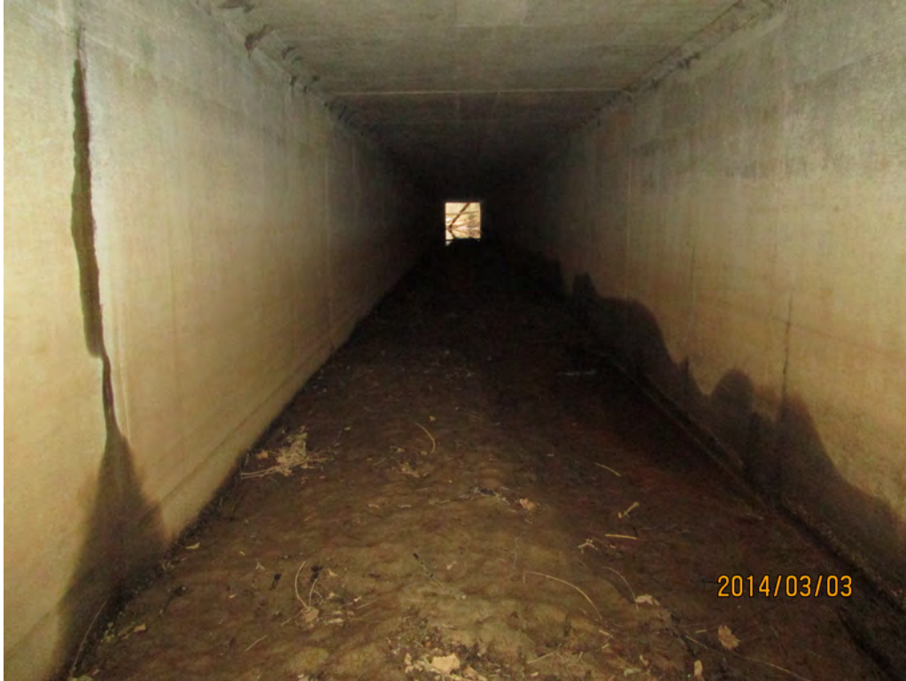
Looking Downstream in Right Box
