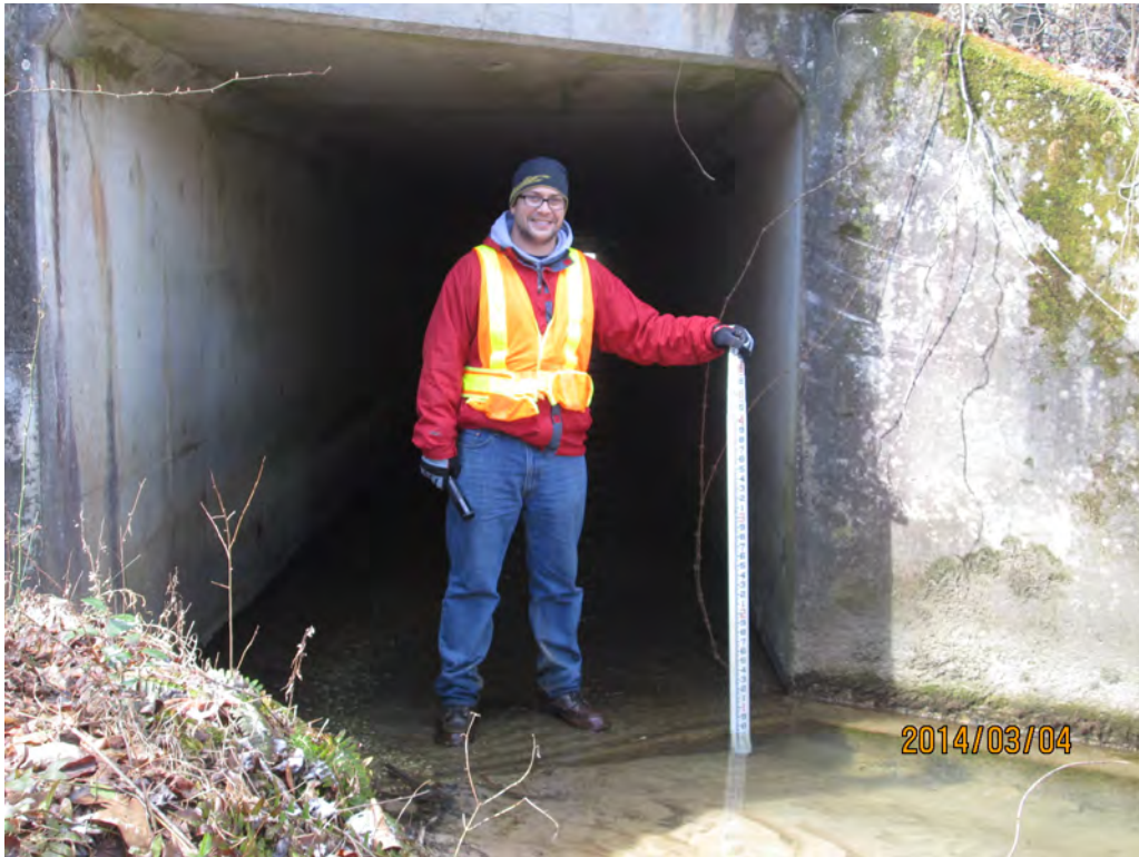
Looking at Upstream Face of 1 @ 7' x 7' RCBC under I-26
