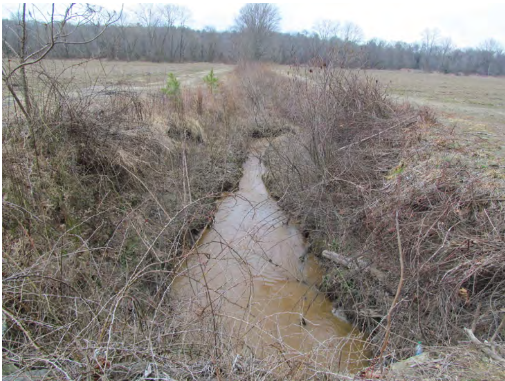
Downstream of 54" CMP with Rock Headwall
