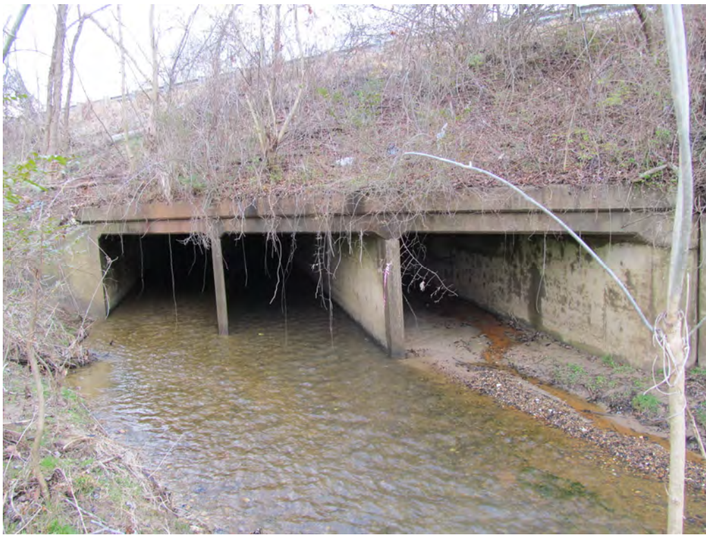
Looking at Downstream Face of 3 @ 7' x 7' RCBC
