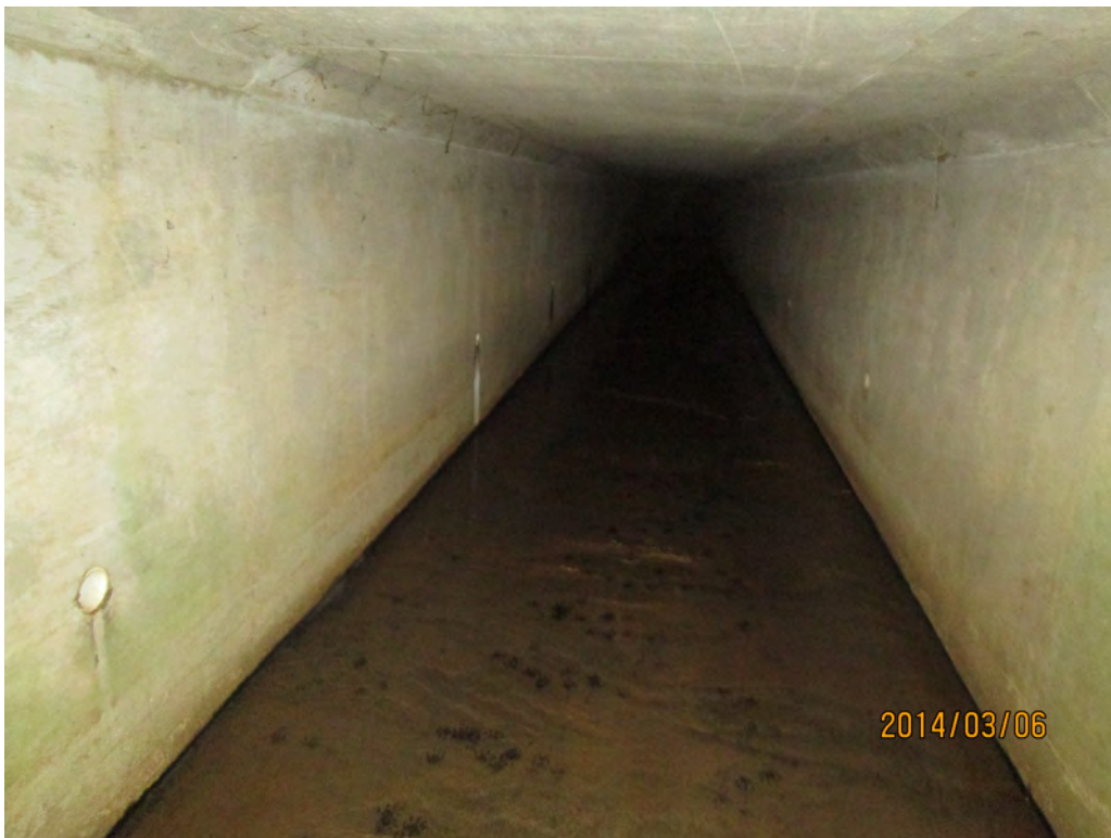
Looking Downstream Inside 1 @ 6' x 5' RCBC
