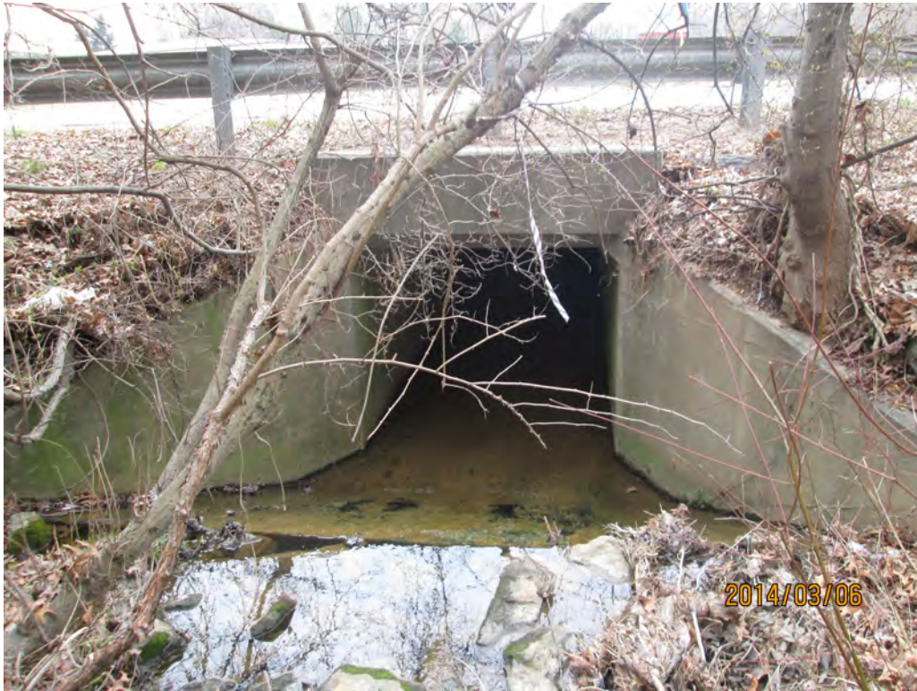
Looking at Upstream Face of 1 @ 6' x 5' RCBC under Airport Rd.
