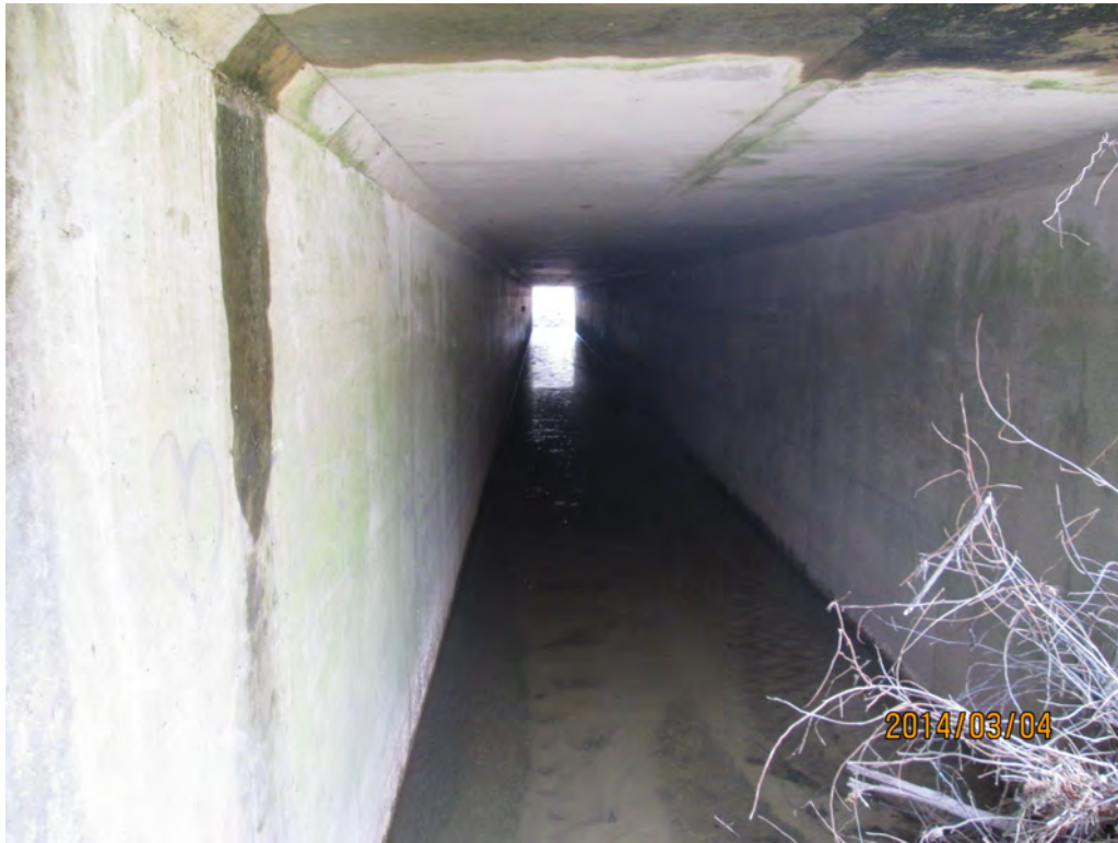
Looking Downstream in Left Barrel
