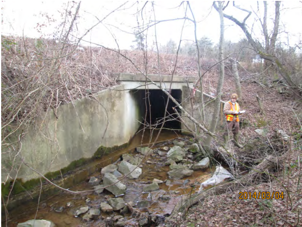
Looking at Downstream Face of 1 @ 6' x 6' RCBC under I-26
