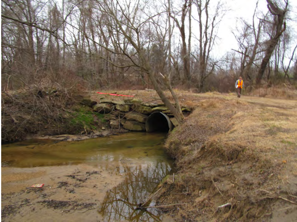
Looking at Downstream Face of 78" CMP
