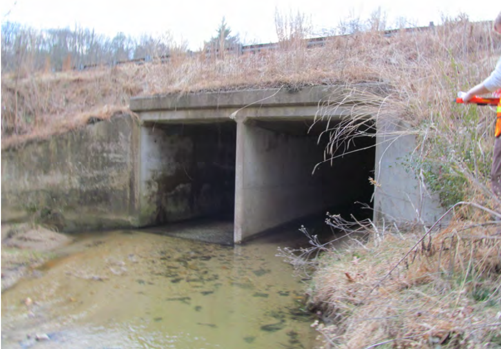
Looking at Upstream Face of 2 @ 8' x 8' RCBC under I-26
