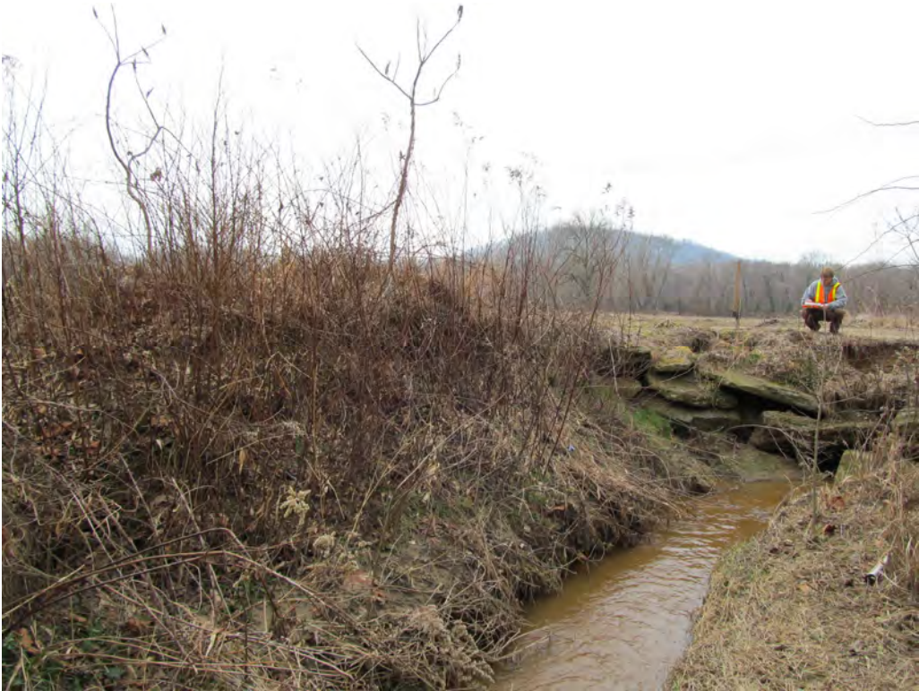
Looking Downstream from 1 @ 7' x 7' RCBC Outlet
