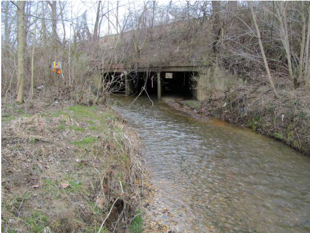
Looking at Downstream Face of 3 @ 7' x 7' RCBC under I-26
