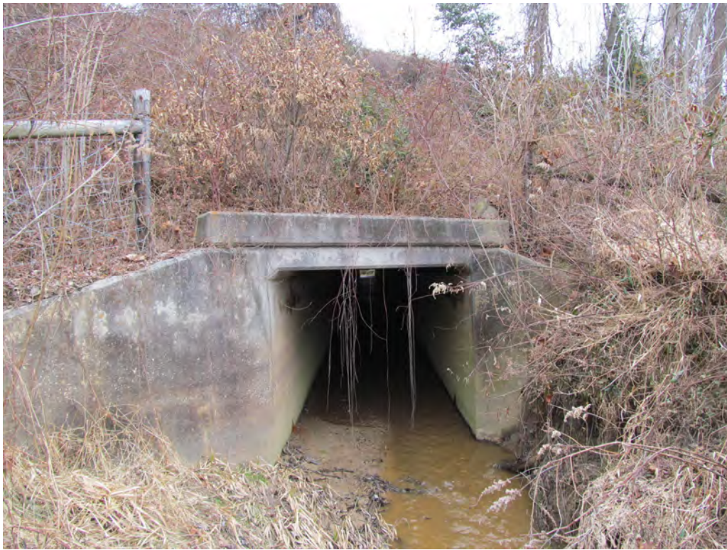
Looking at Downstream Face of 1 @ 7' x 7' RCBC under I-26
