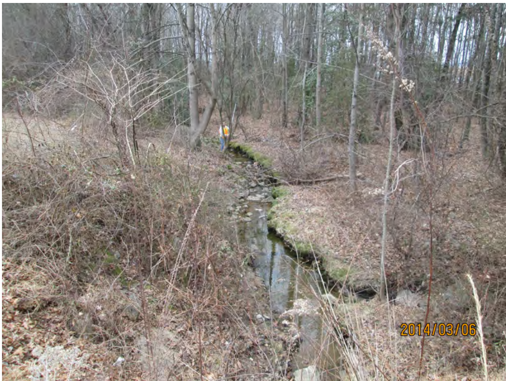
Looking Downstream 66" RCP
