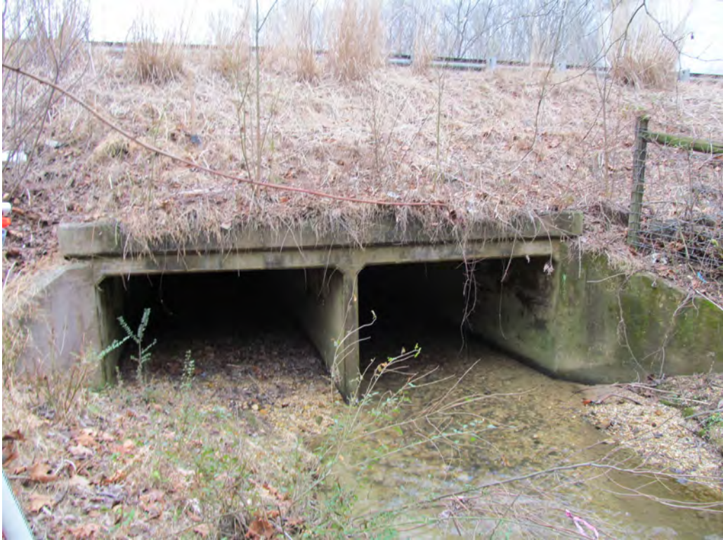
Looking at Downstream Face of 2 @ 8' x 8' RCBC under I-26
