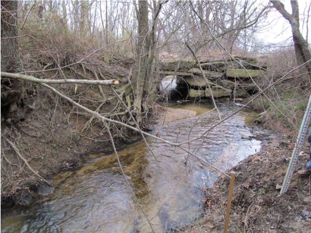
Looking at Upstream Face of 78" CMP
