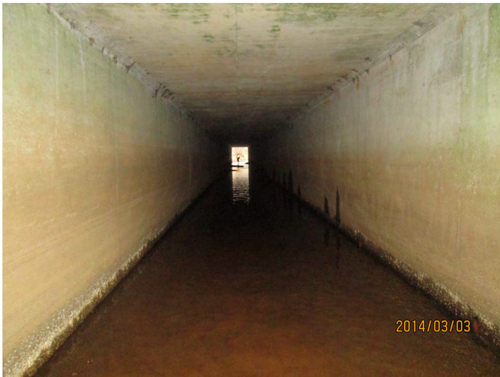
Looking Upstream in Left Box
