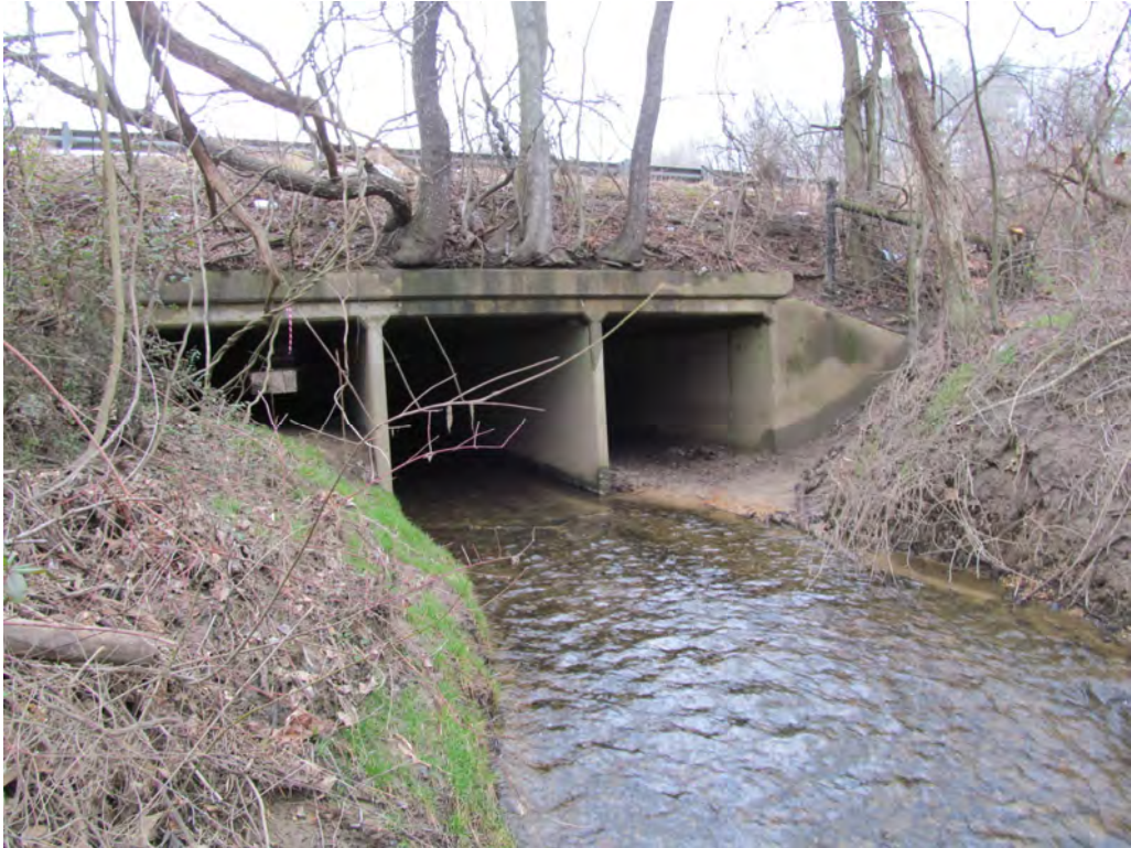
Looking at Downstream Face of 3 @ 8' x 8' RCBC under I-26
