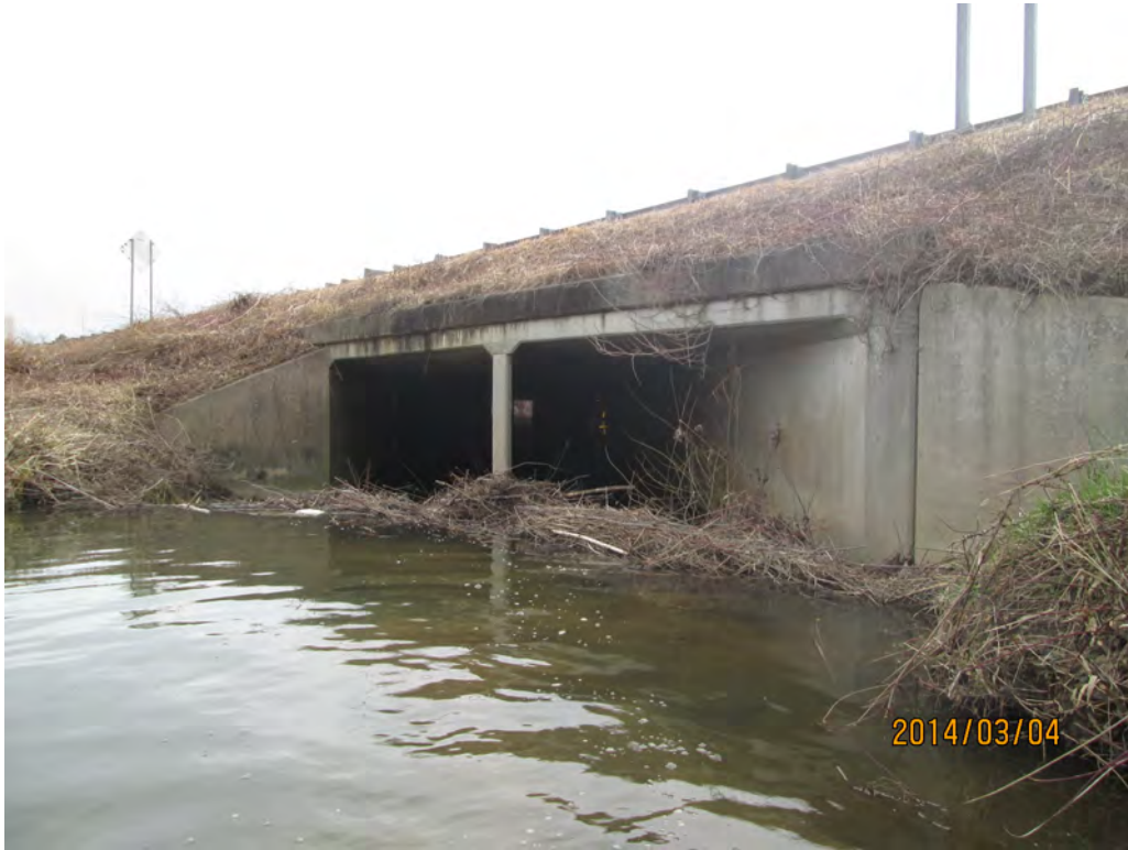
Looking at Upstream Face of 2 @ 8' x 8' RCBC under I-26
