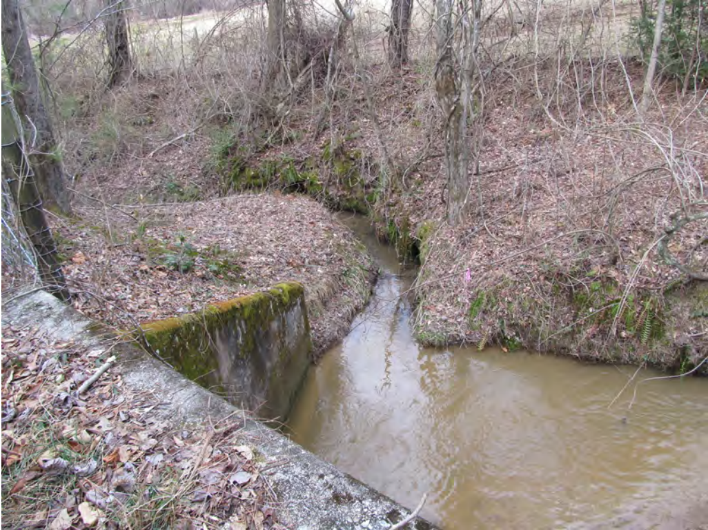
Looking at Upstream Channel coming from the right
