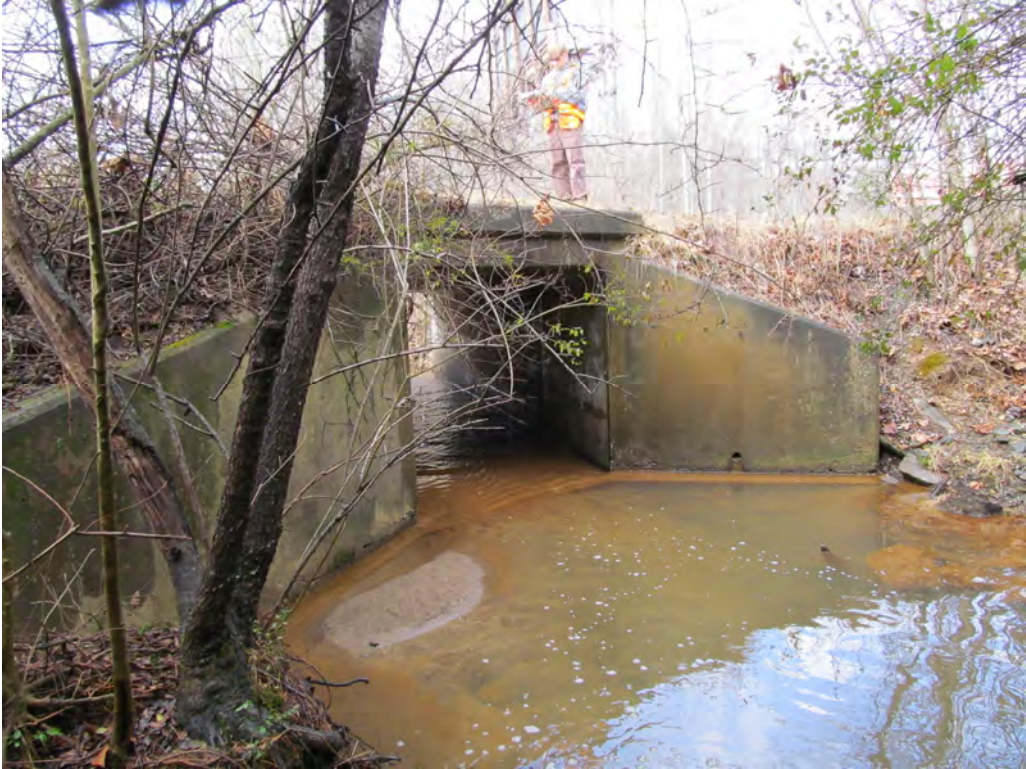
Looking at Upstream Face of 1 @ 6' x 6' RCBC under Hidden Creek Rd
