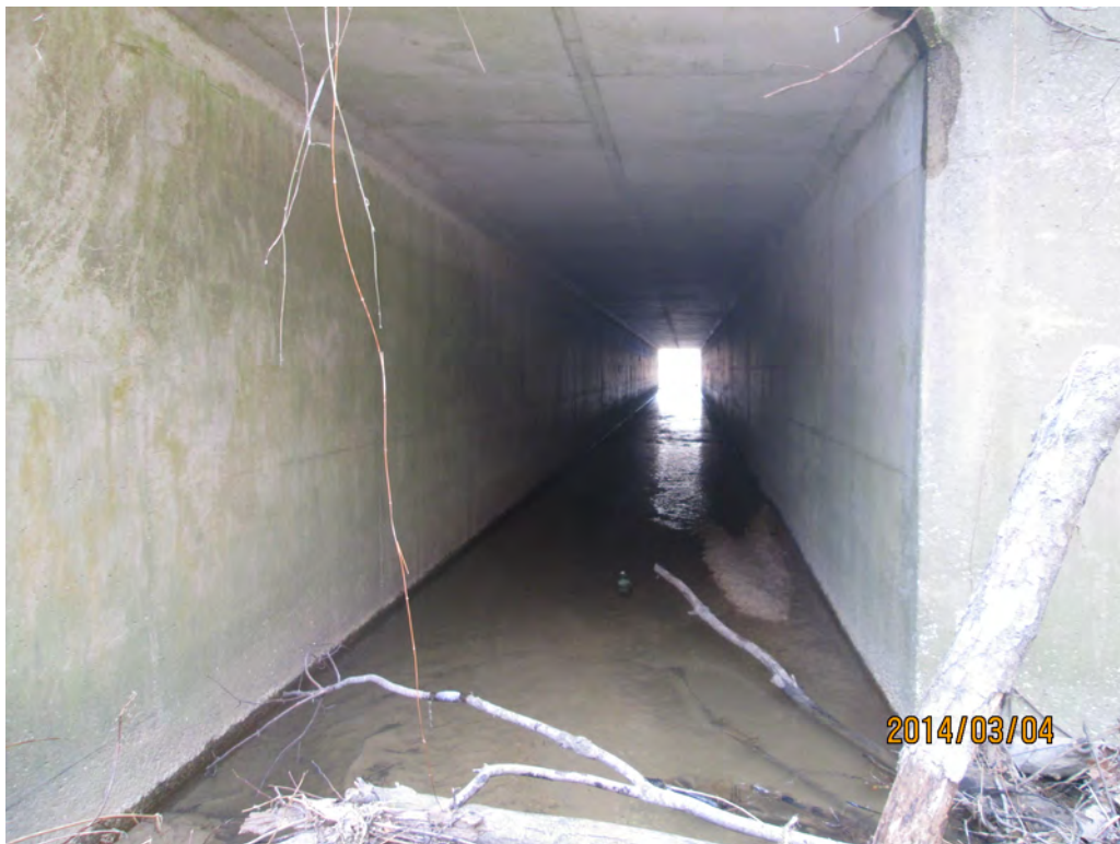
Looking Downstream in Right Barrel
