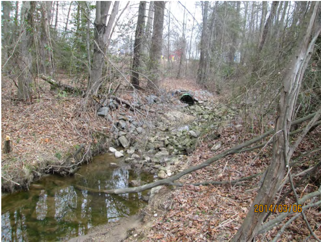
Pipe located Upstream of 1 @ 6' x 5' RCBC
