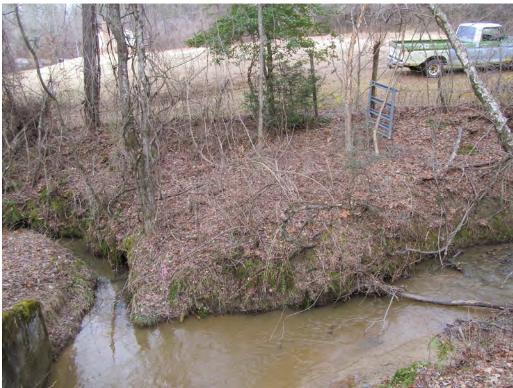
Looking Upstream from 1 @ 7' x 7' RCBC Inlet
