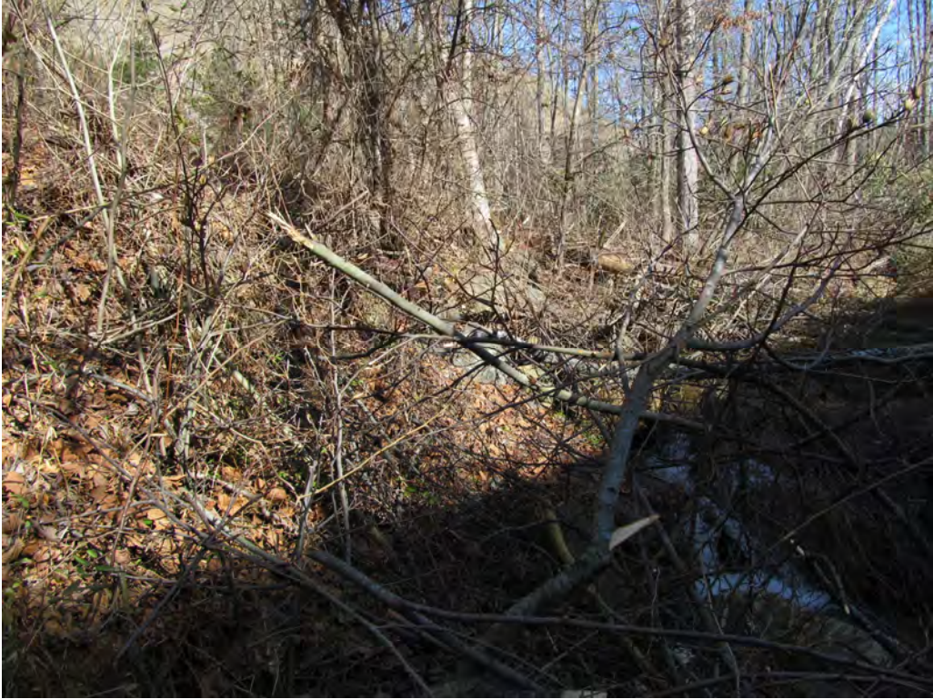
Looking Upstream from 1 @ 8' x 8' RCBC Inlet
