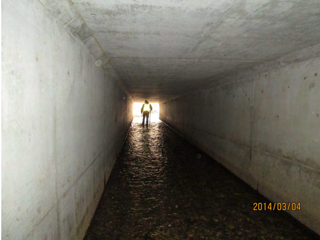
Looking Downstream in Left Barrel
