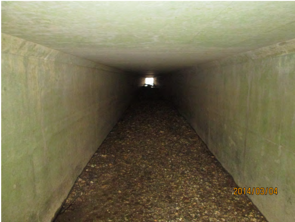
Looking Downstream in Left Barrel
