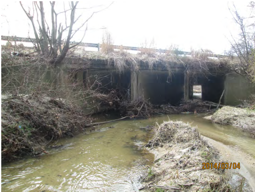
Looking at Upstream Face of 3 @ 9' x 10' RCBC under I-26
