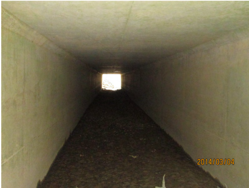
Looking Downstream in Left Barrel
