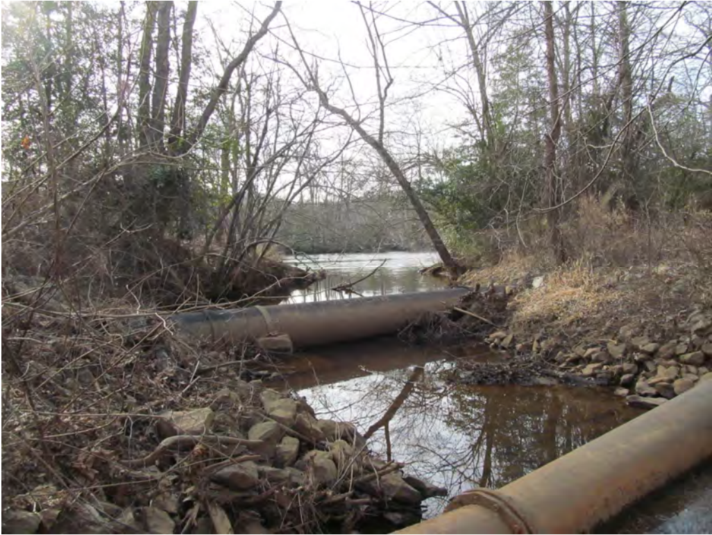
Looking Downstream from 2 @ 10' x 10' RCBC Outlet
