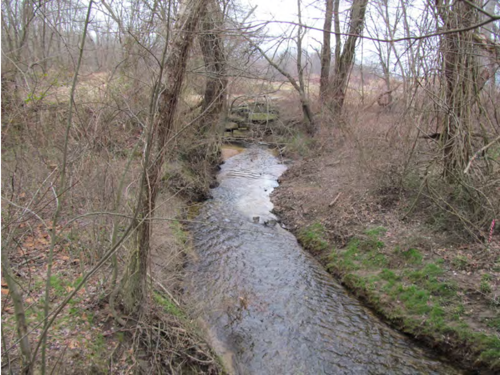
Looking Downstream from 3 @ 8'x 8' RCBC Outlet
