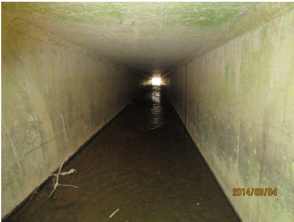
Looking Downstream in Center Barrel
