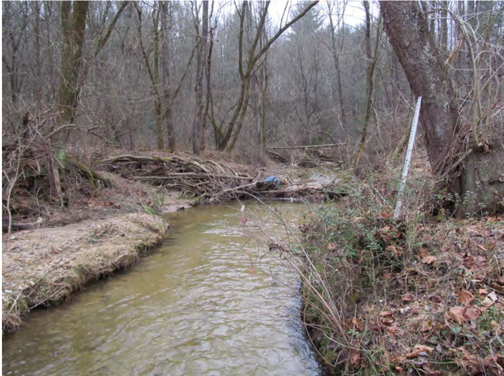
Looking Downstream from 2 @ 8' x 8' RCBC
