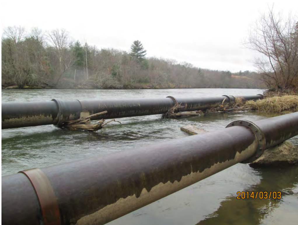
Looking Downstream from 1 @ 8' x 8' RCBC Outlet
