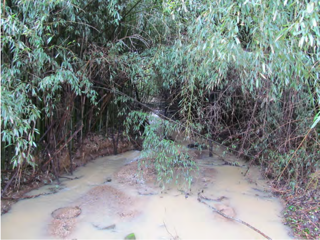
Looking Downstream from 1 @ 6' x 6' RCBC Outlet
