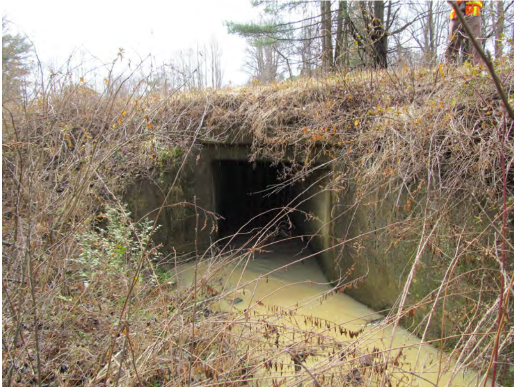
Looking at Upstream Face of 1 @ 6' x 6' RCBC under I-26
