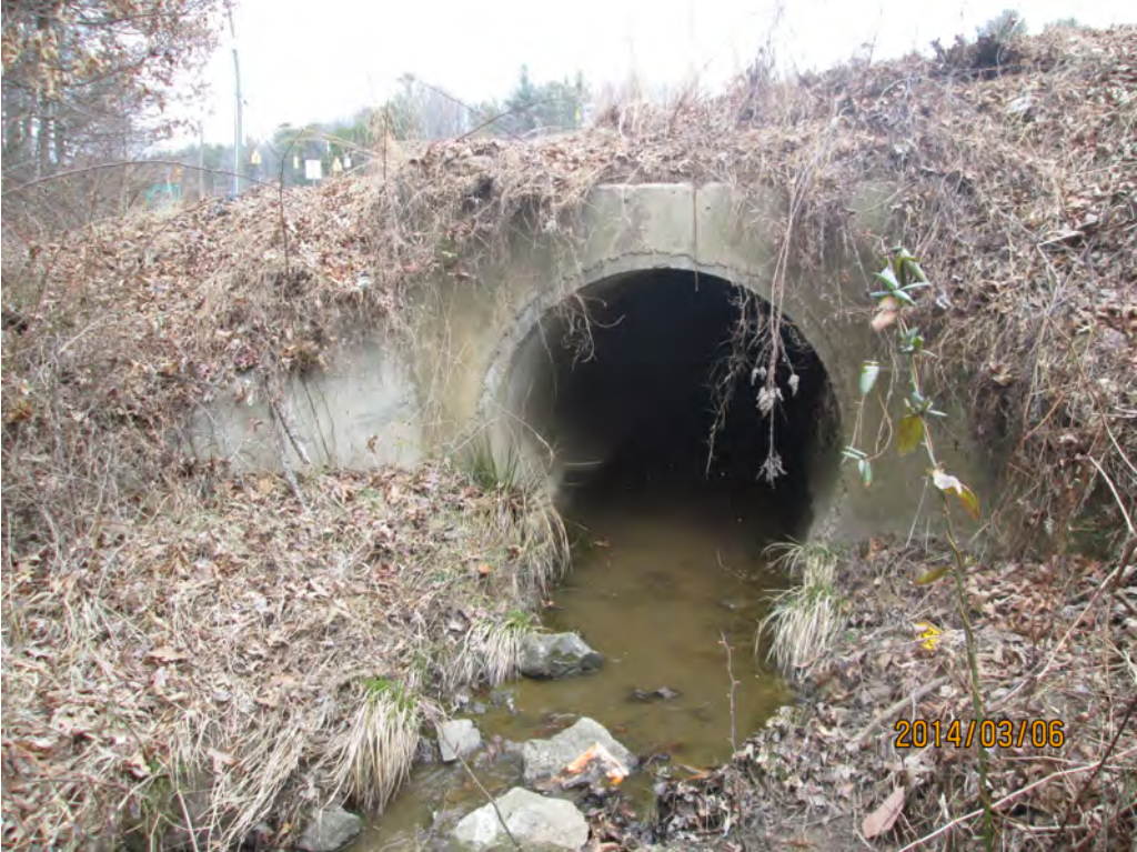
Looking at Downstream Face of 66" RCP with Headwall under Airport Rd.
