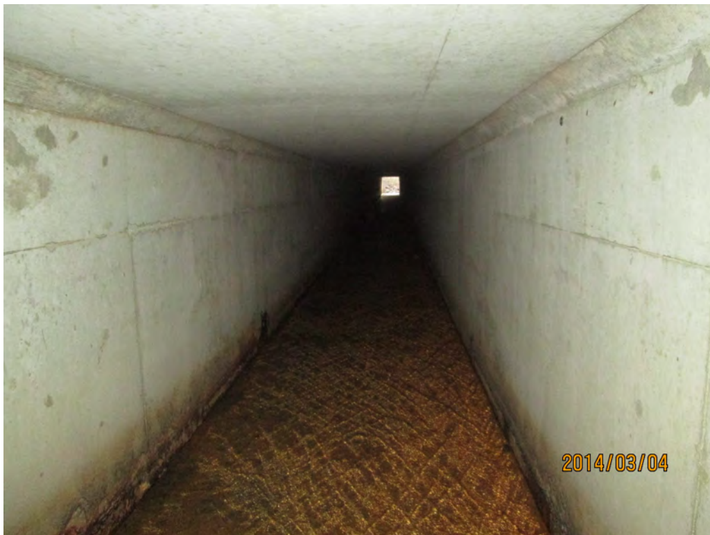
Looking Upstream of 1 @ 6' x 6' RCBC
