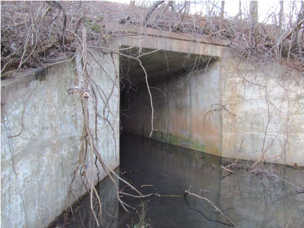
Downstream Side of Vehicular Underpass
