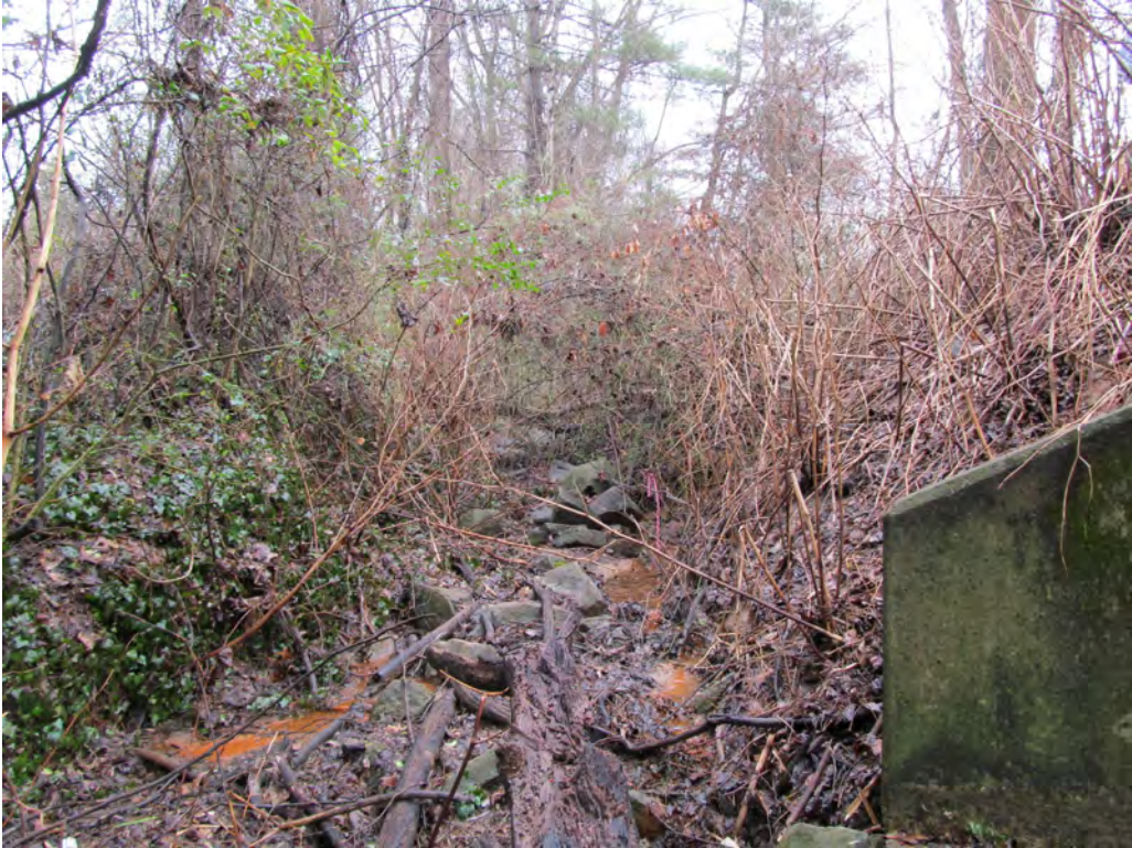
Looking at Downstream Right Ditch
