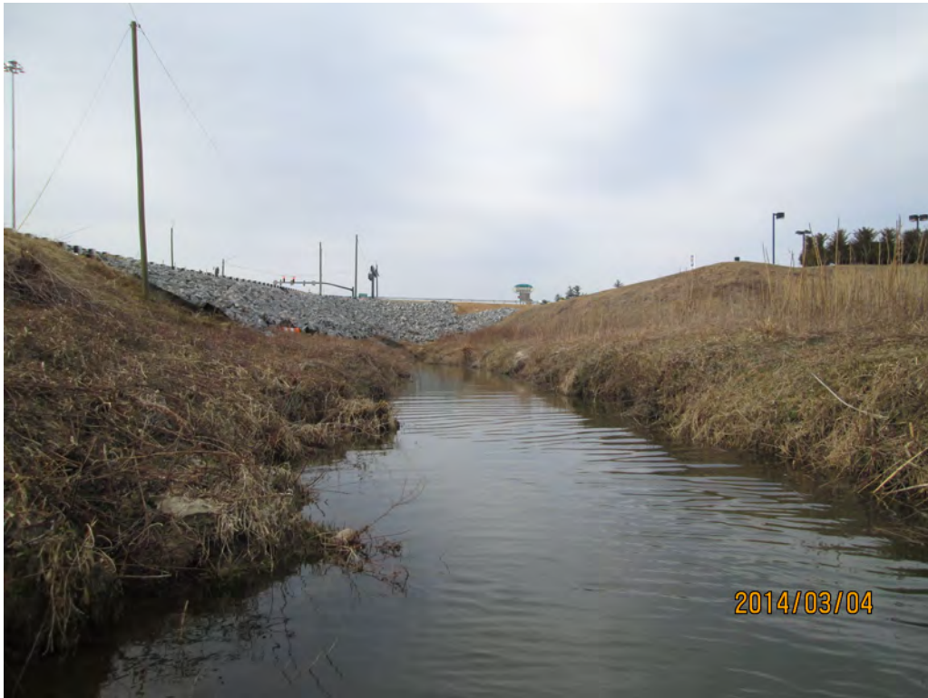
Looking Upstream from 2 @ 8' x 8' RCBC Inlet
