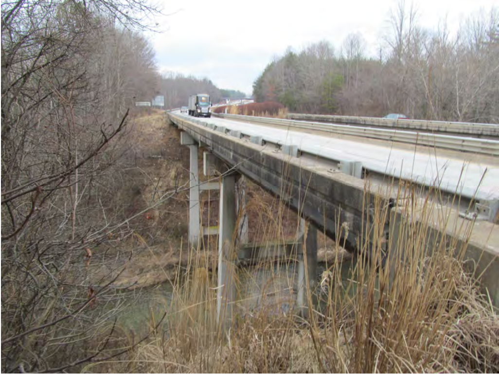
Looking at Downstream Face
