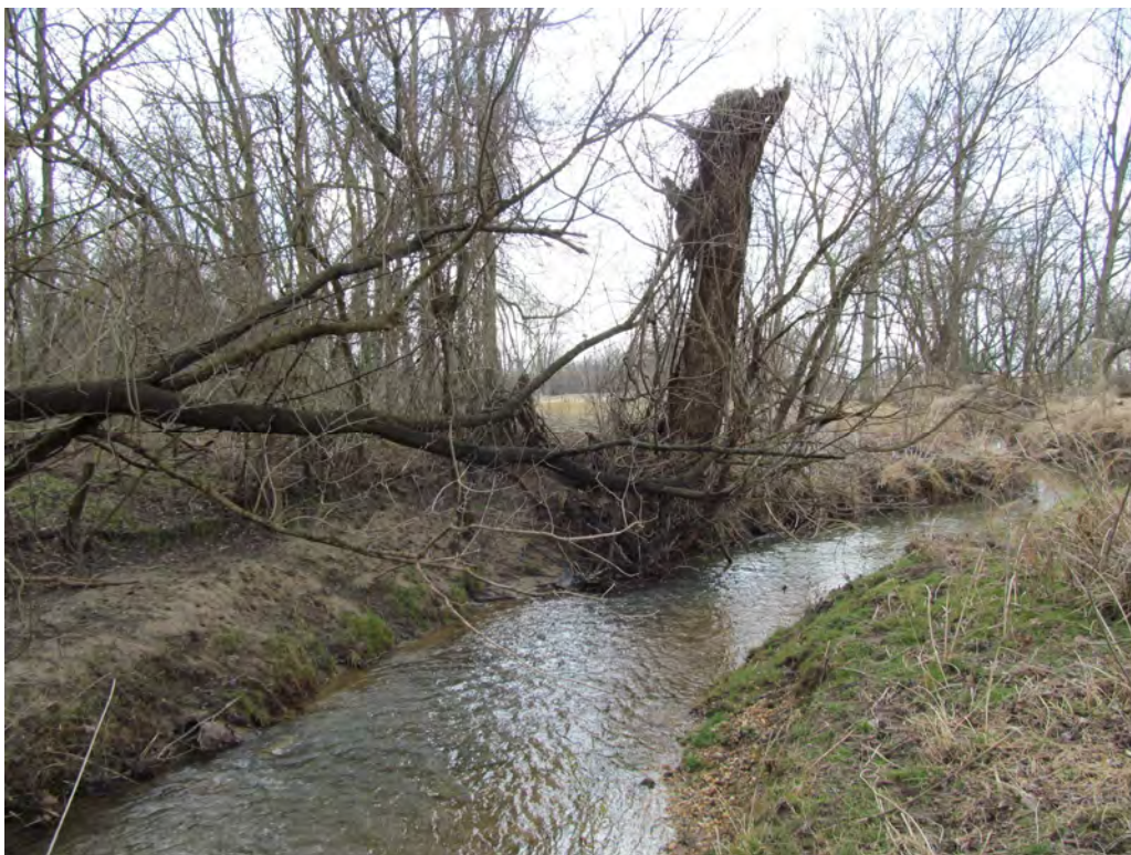
Looking Downstream of 3 @ 7' x 7' RCBC
