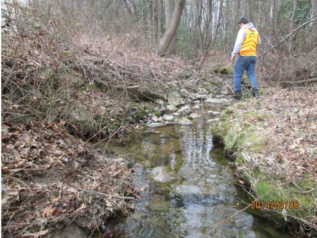
Looking Downstream from 66" RCP
