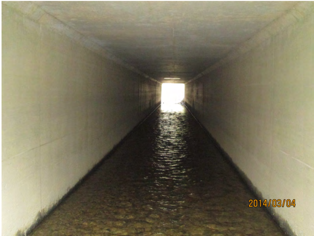
Looking Upstream in Center Barrel
