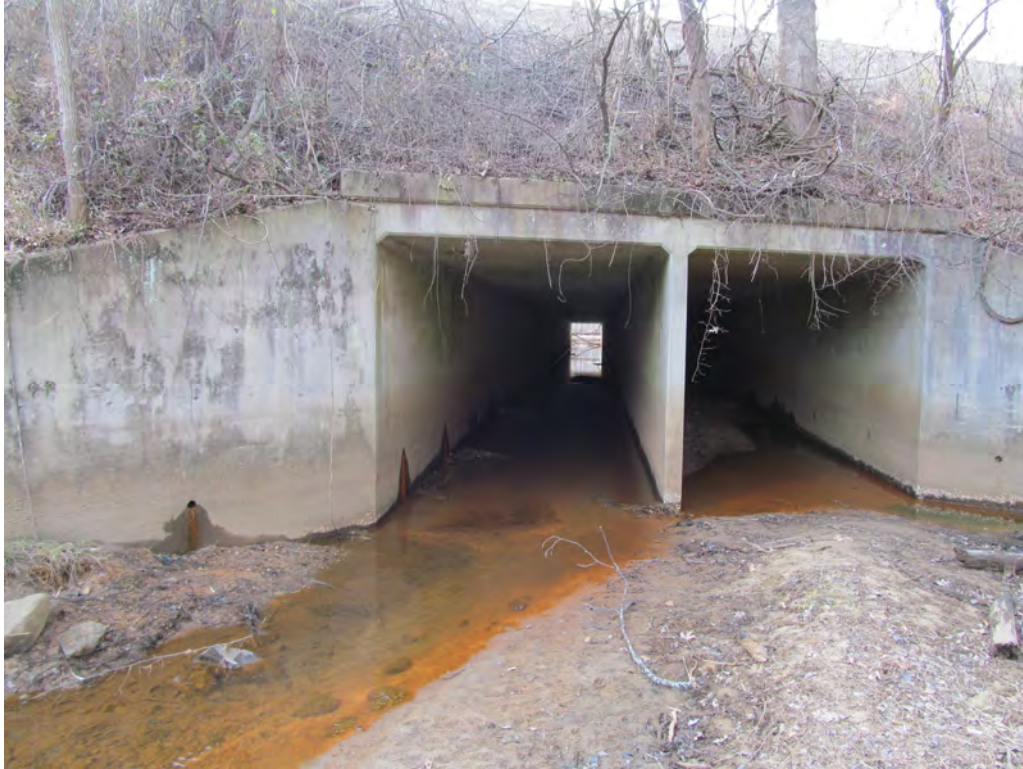
Looking at Upstream Face of 2 @ 10' x 10' RCBC under I-26
