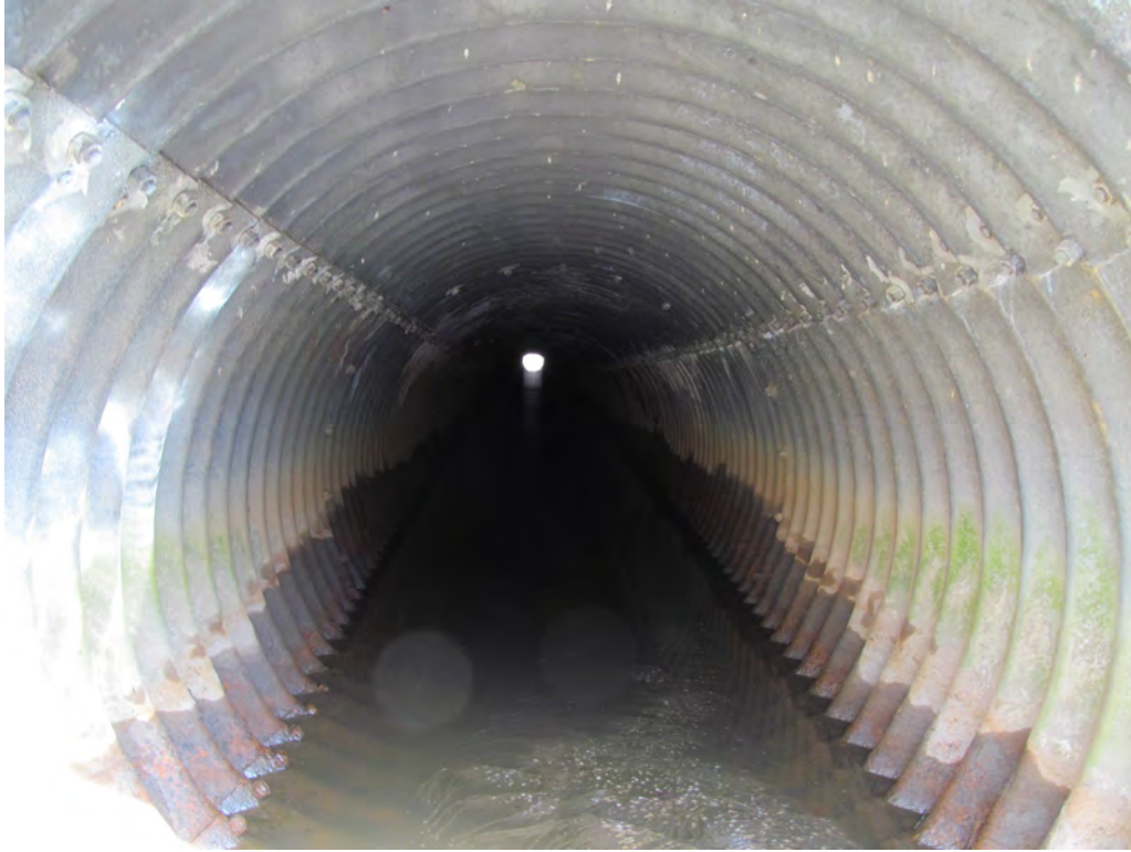
Looking Downstream Inside of 66" SPP
