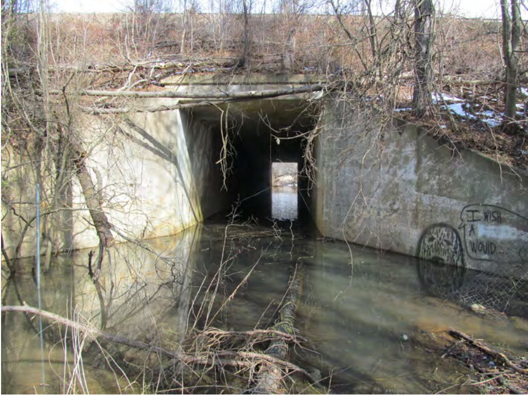
Upstream Side of Vehicular Underpass
