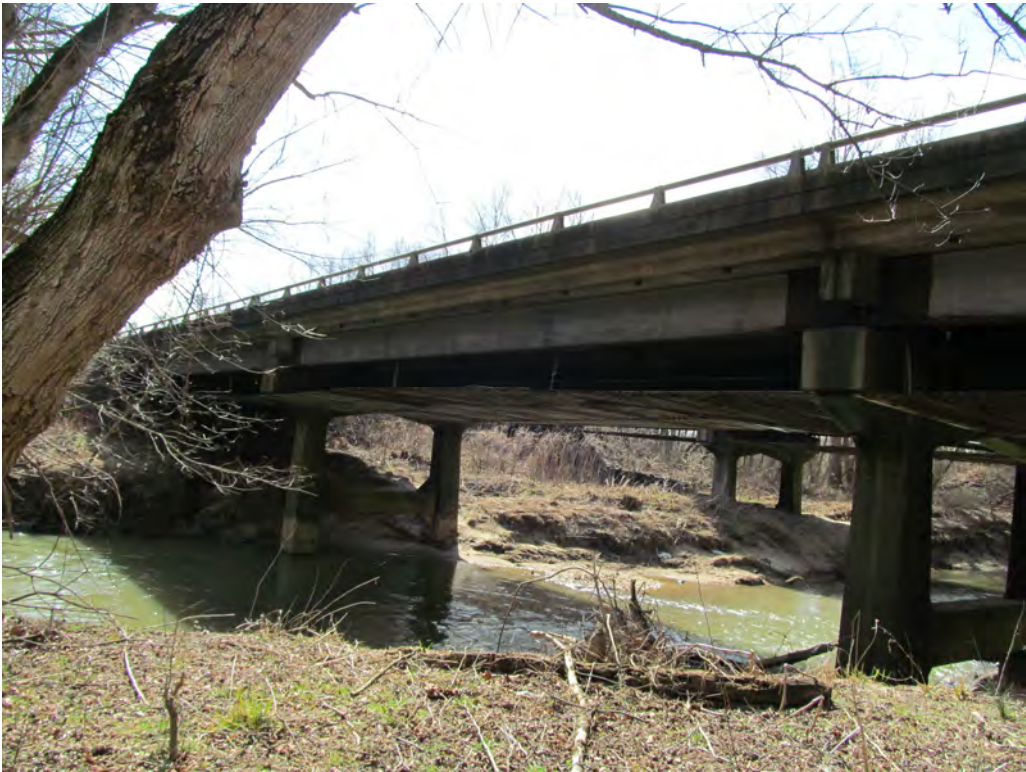
Looking at Downstream Face
