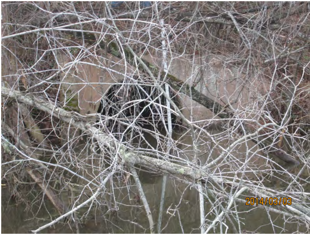
Looking at Downstream Face of 66" SPP with Headwall under I-26
