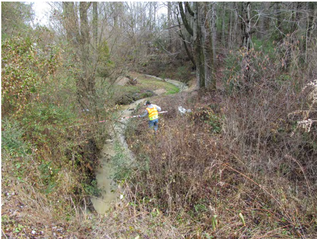
Looking Upstream from 1 @ 6' x 6' RCBC Inlet
