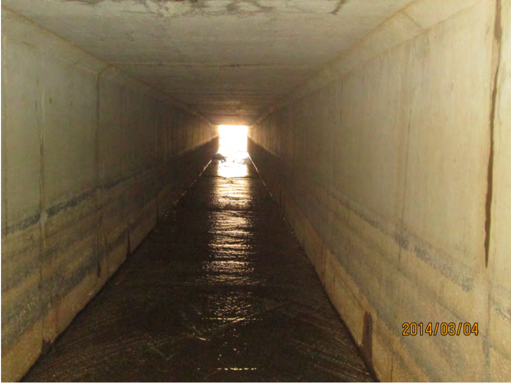
Looking Downstream inside of the Barrel
