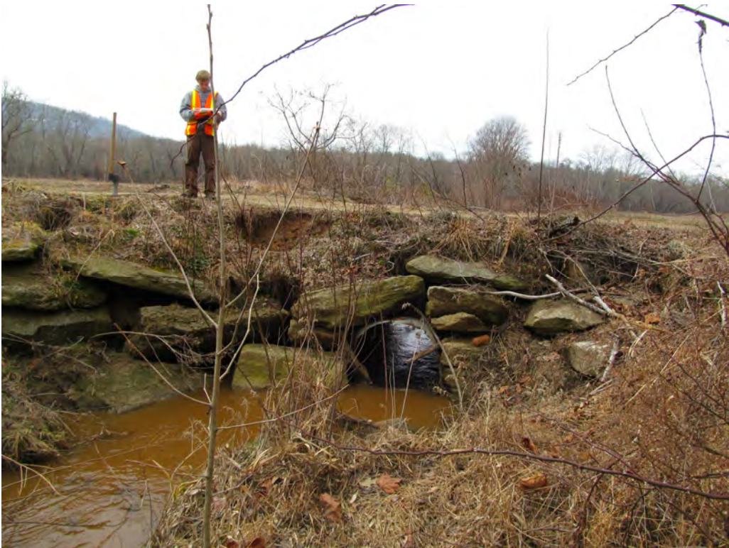
Upstream Face of Downstream 54" CMP with Rock Headwall
