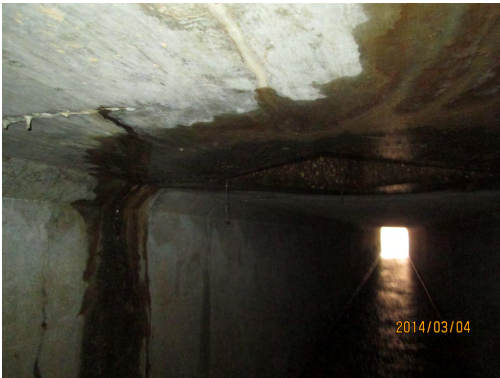
Outlet of Drop Inlet Inside 1 @ 6' x 6' RCBC
