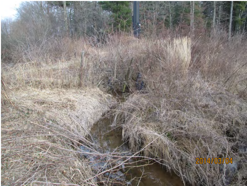
Looking Upstream from 1 @ 6' x 6' RCBC Inlet
