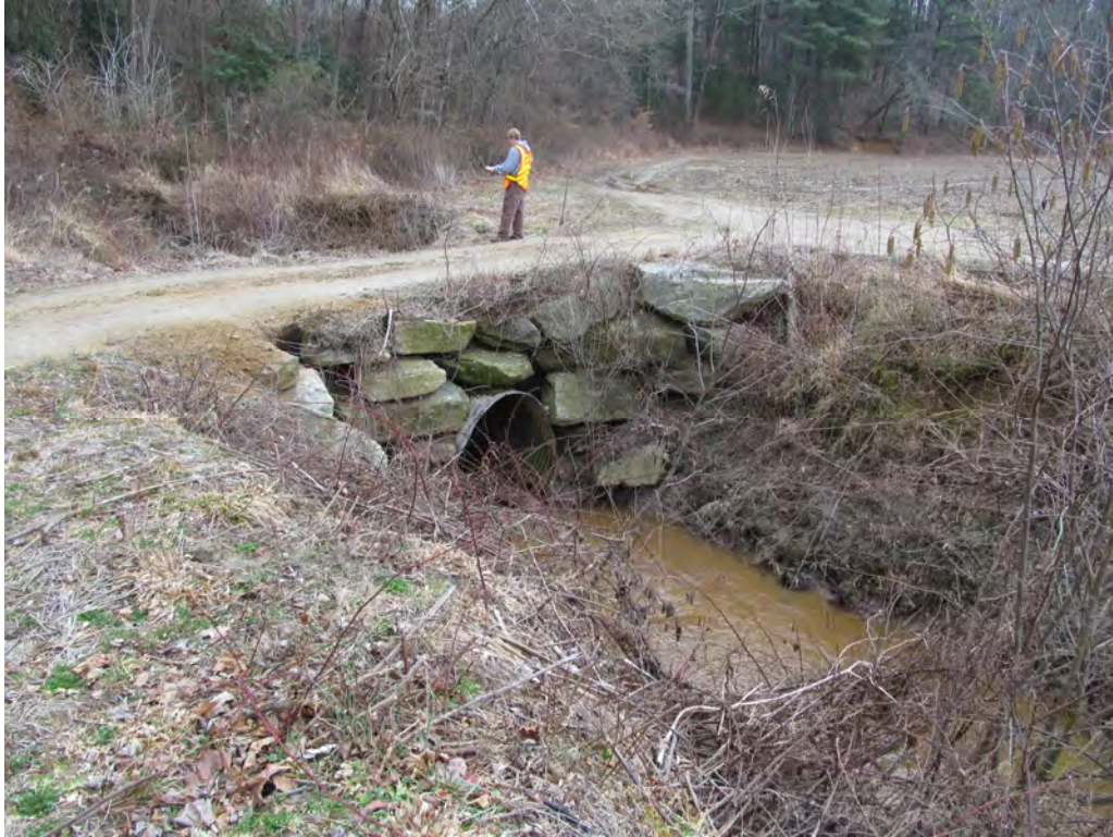
Downstream Face of Downstream 54" CMP with Rock Headwall
