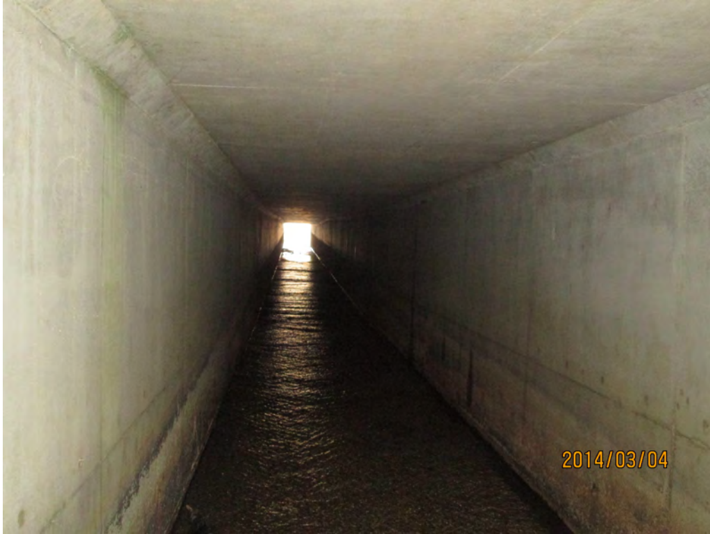
Looking Downstream inside of the Barrel
