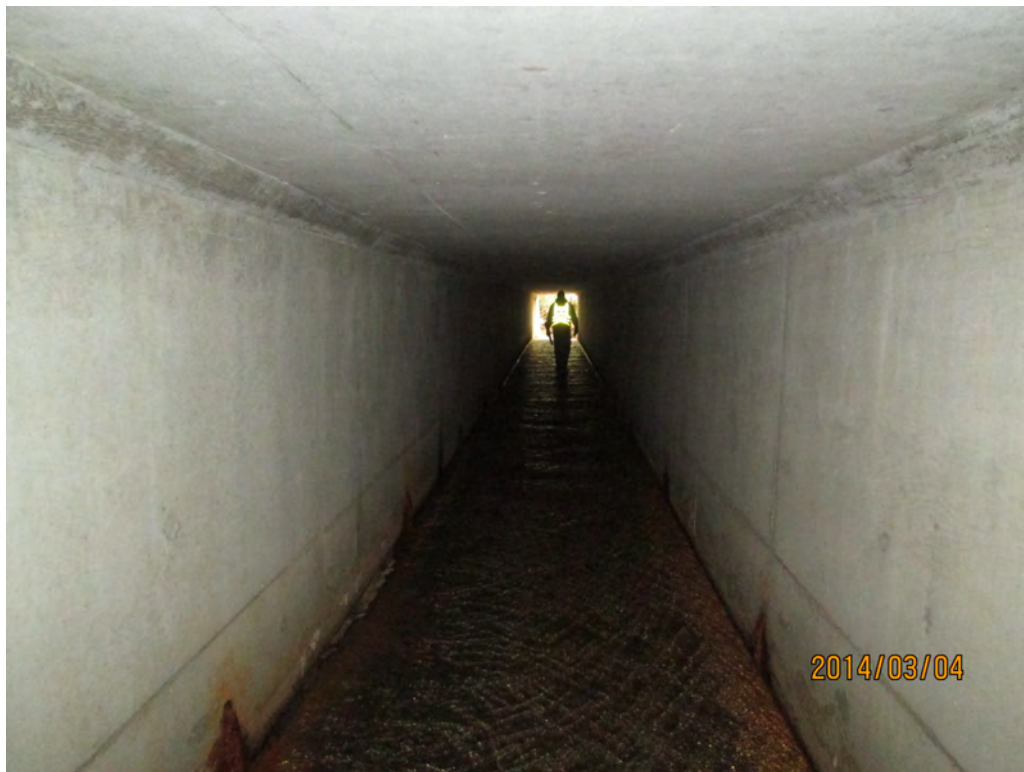
Looking Downstream Inside of the Barrel
