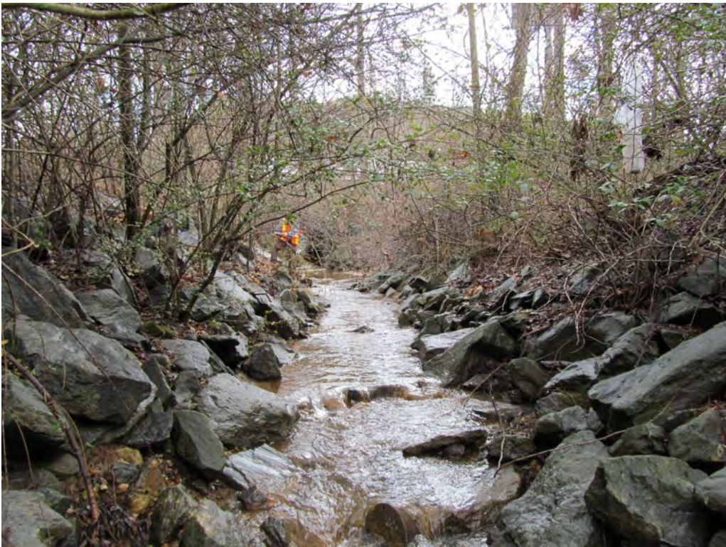
Looking Upstream from 1 @ 6' x 6' RCBC Inlet
