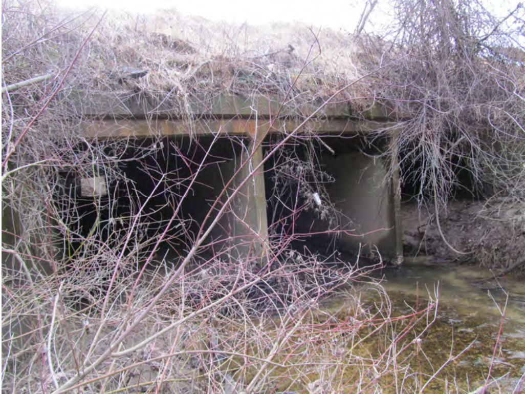
Looking at Upstream Face of 3 @ 8' x 8' RCBC under I-26
