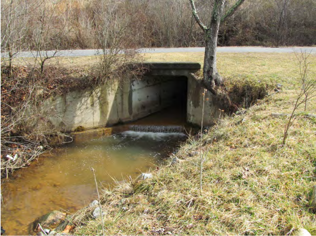
Looking at Downstream Face of 1 @ 6' x 6' RCBC under Hidden Creek Rd
