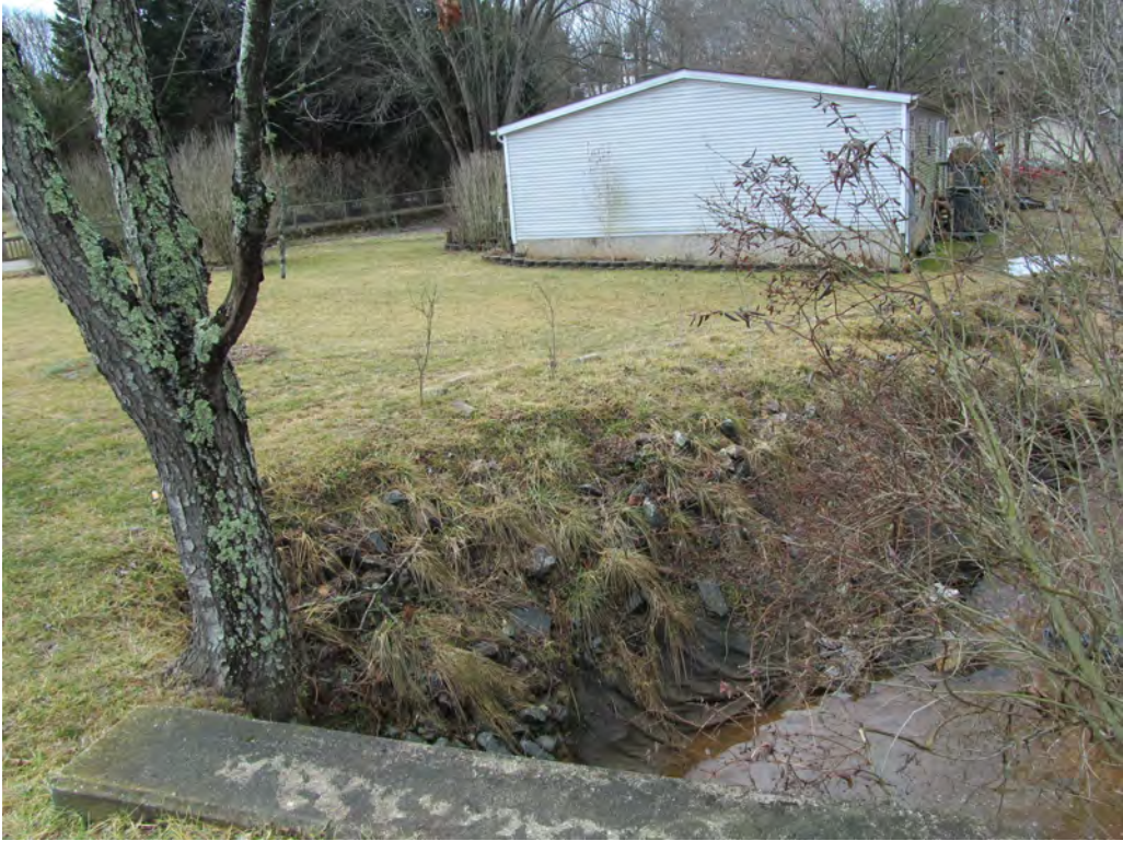
Home Downstream of Hidden Creek Rd
