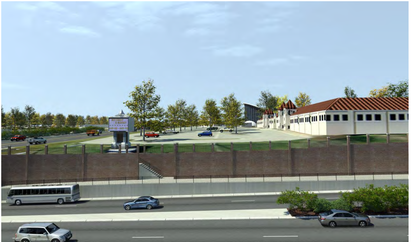
Alternative 12 – view west towards Blue Ridge Road and the retaining wall along the NC State Fairgrounds Source: NCDOT
