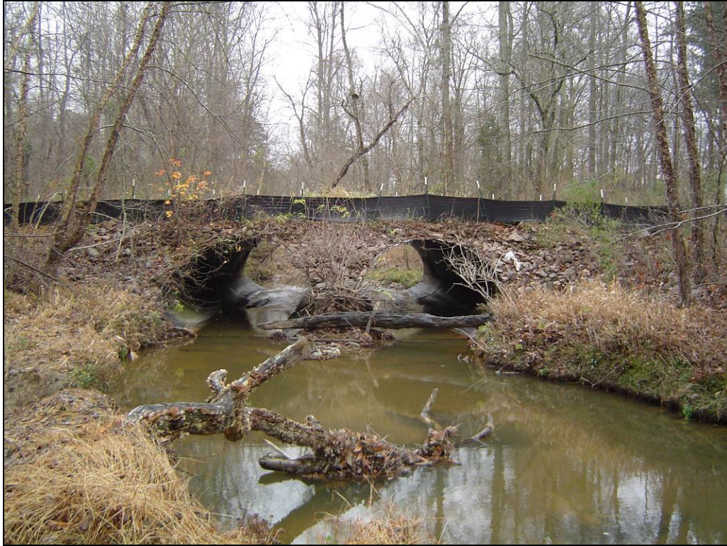
Looking downstream at existing 2@12'x7.5' CSPA w/ 2/3 asphalt paving
