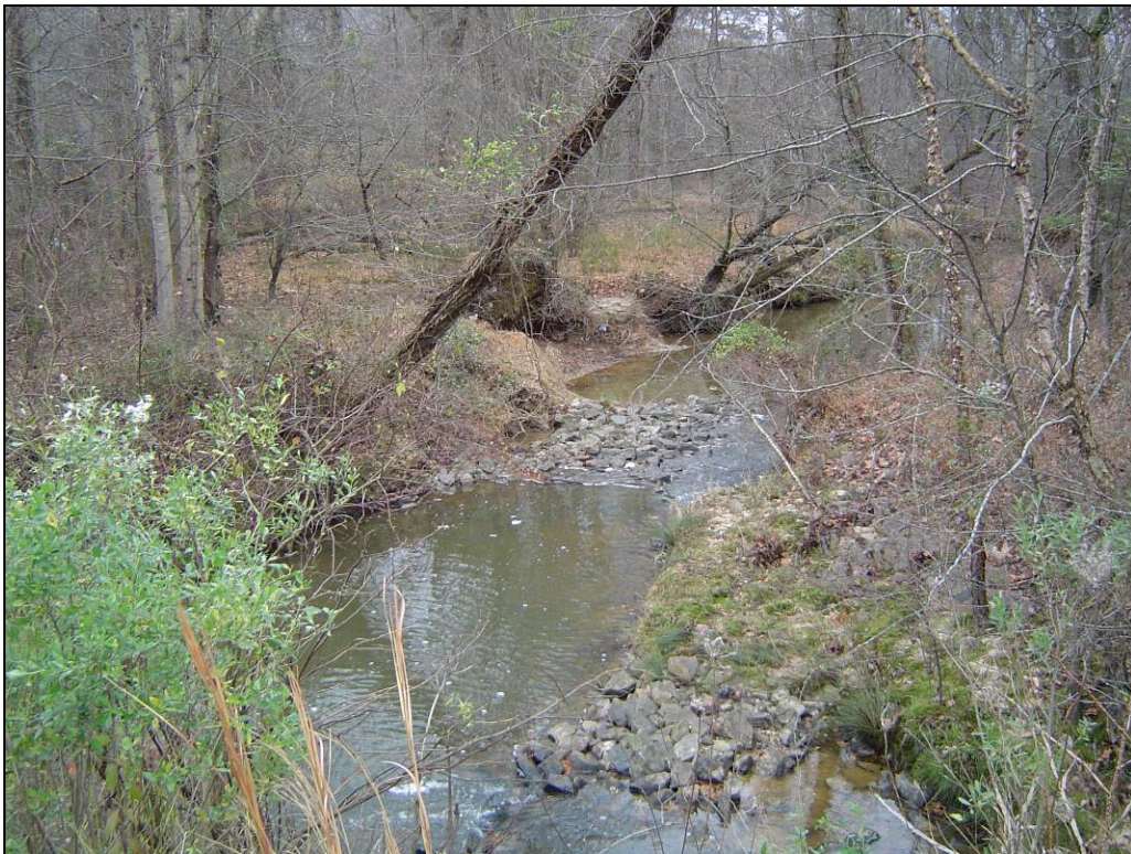
Looking Downstream from Sunset Lake Road (Proposed Site)
