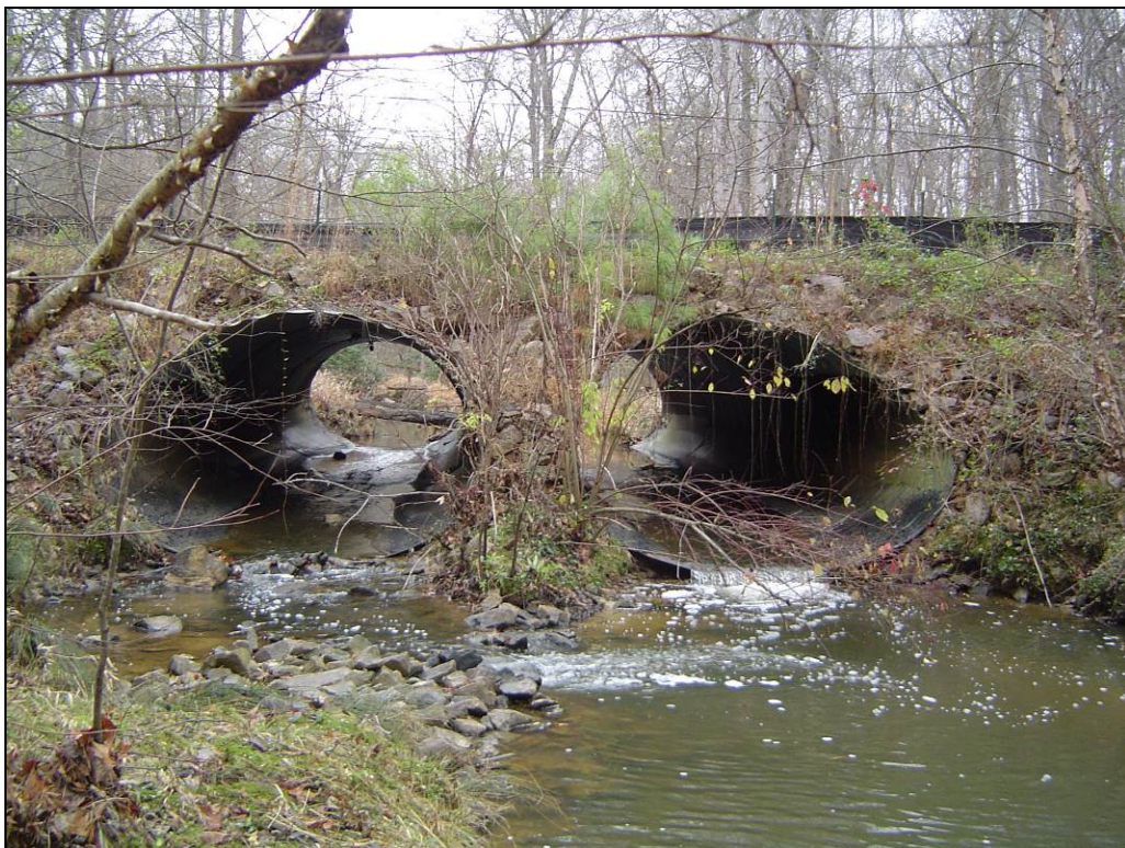
Looking upstream at existing 2@12'x7.5' CSPA
