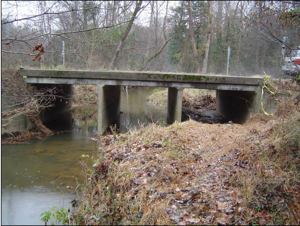
Triple 10'x 9' RCBC Downstream Structure
