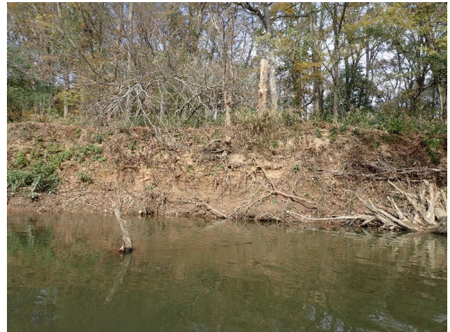
Photo 13. LDB at upstream side of bridge.
