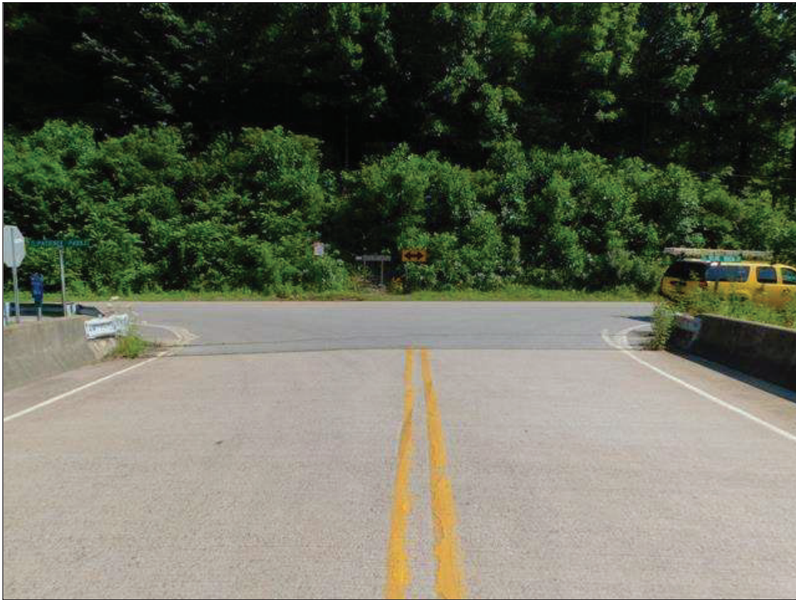
LOOKING NORTH AT APPROACH GUARDRAIL
