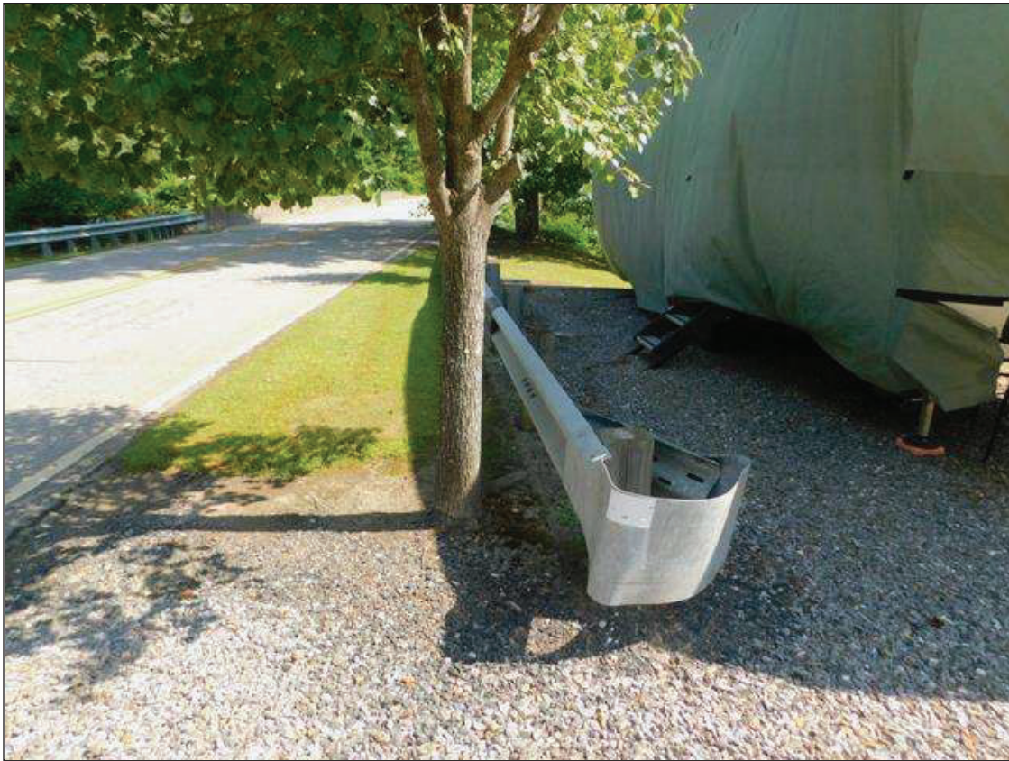
TYPICAL GUARDRAIL END TREATMENT AND POST SPACING
