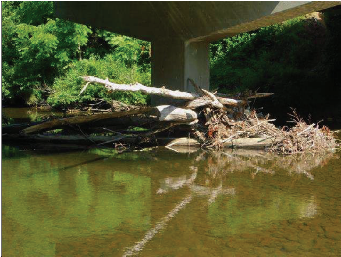
DRIFT 25' WIDE X 5' HIGH X 10' DEEP LODGED AGAINST BENT 2.
