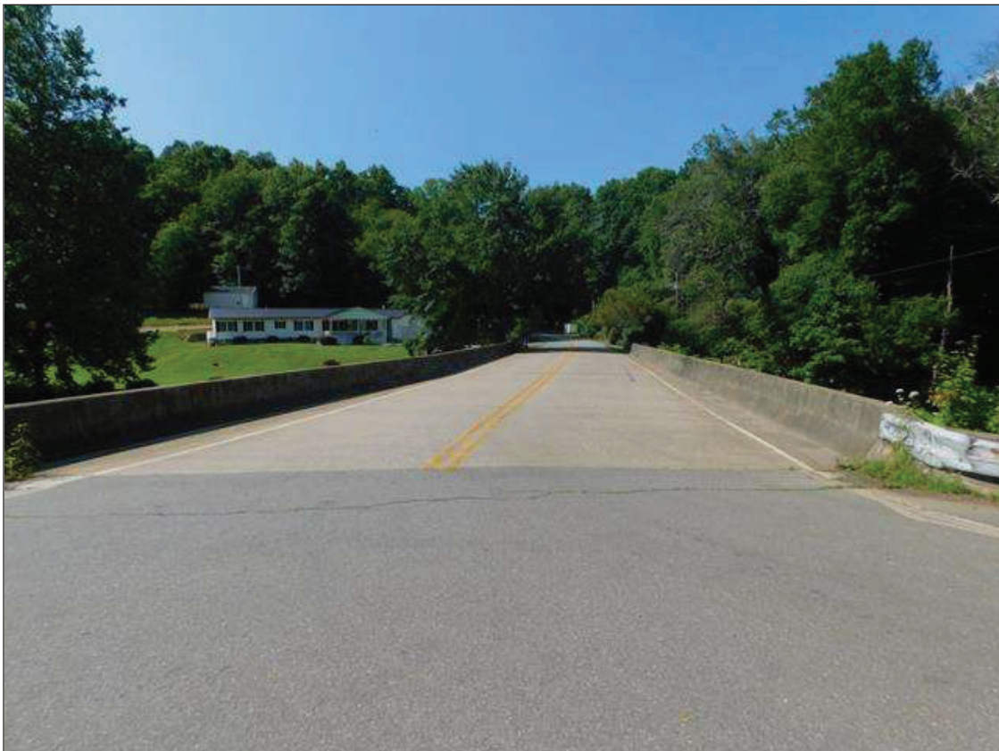
NORTH APPROACH LOOKING SOUTH
