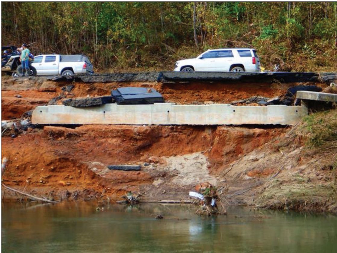
BRIDGE CLOSED. END BENT 2. COULD NOT ACCESS. (PAR)
