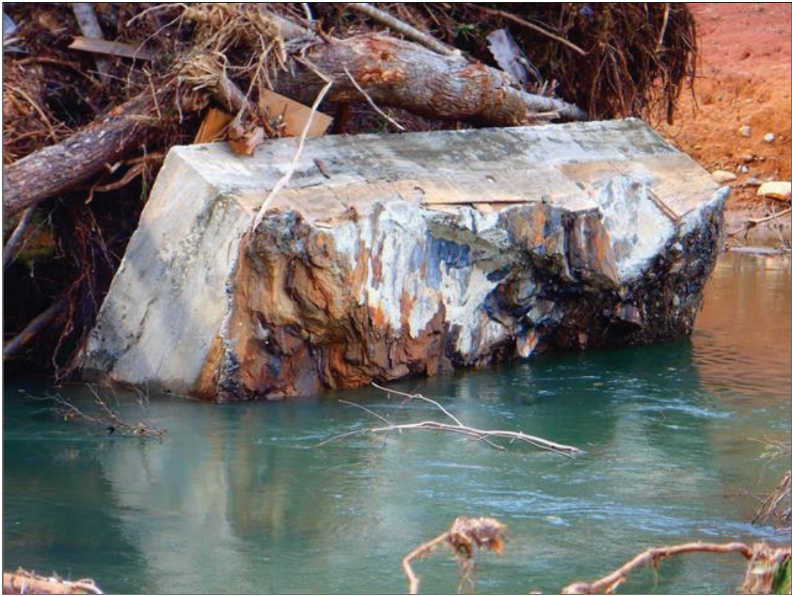
INTERIOR BENT 2 FAILED. (PAR)
