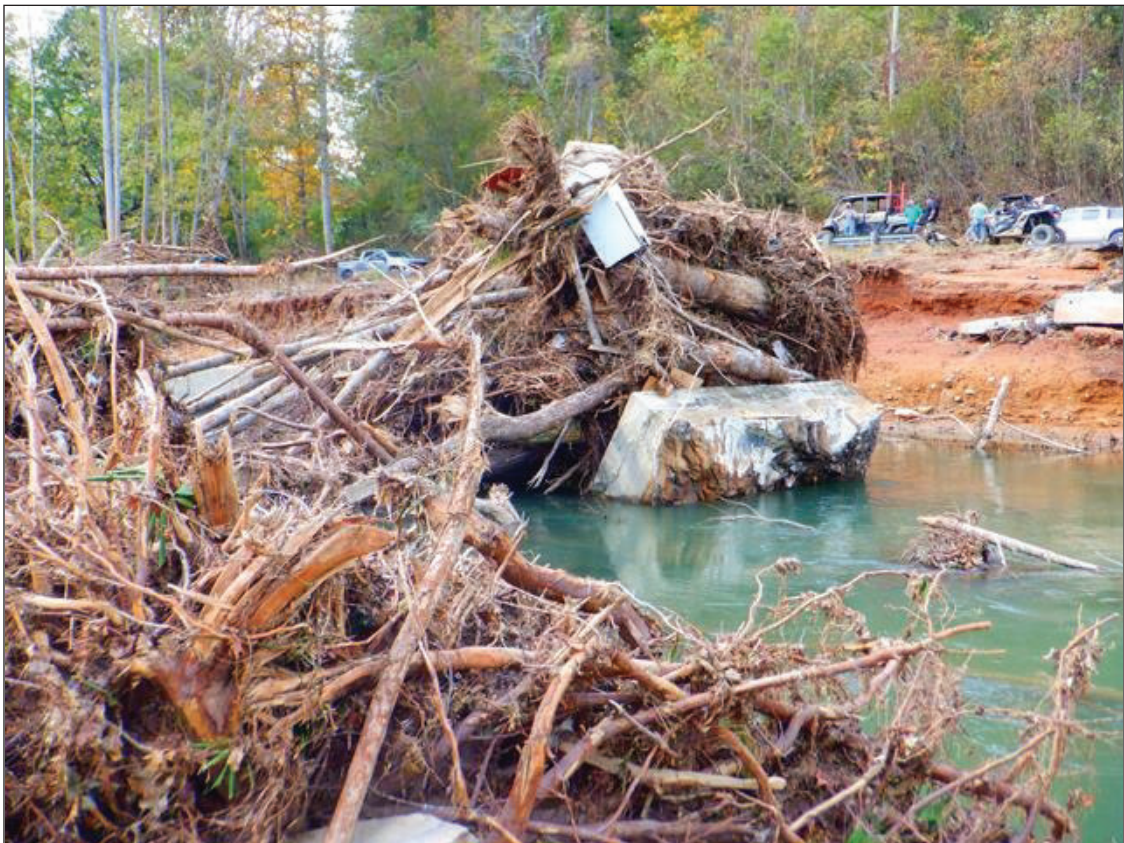
INTERIOR BENT 2 FAILED. (PAR)
