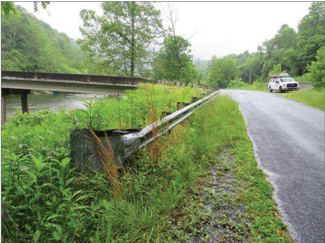
NORTHEAST GUARDRAIL END TERMINAL
