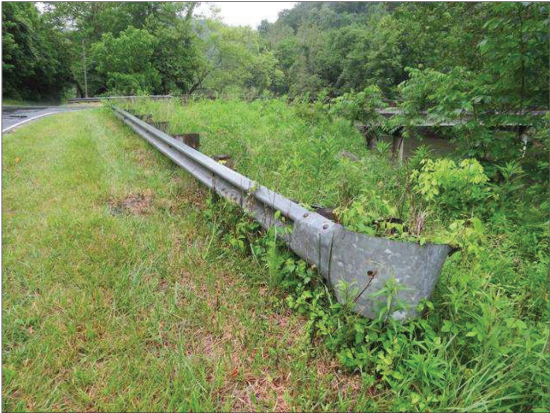
NORTHWEST GUARDRAIL END TERMINAL
