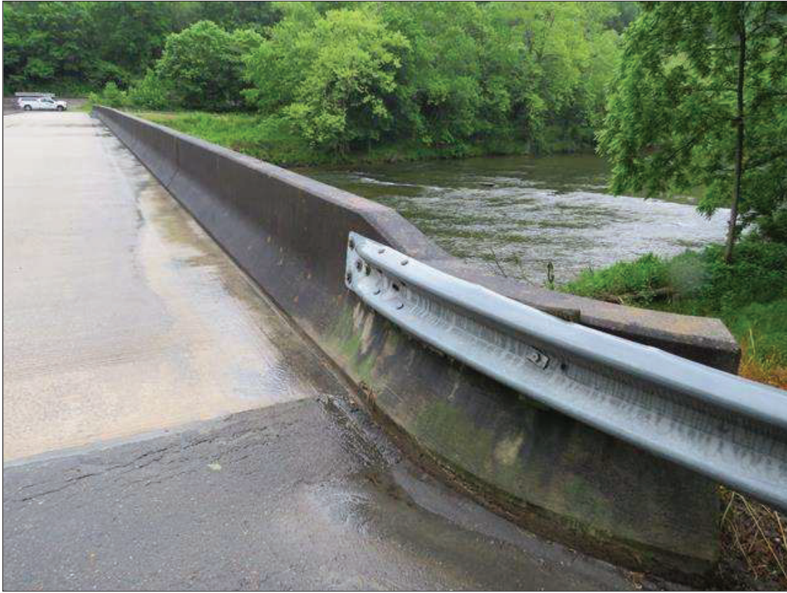
SPAN 1 RIGHT RAIL
