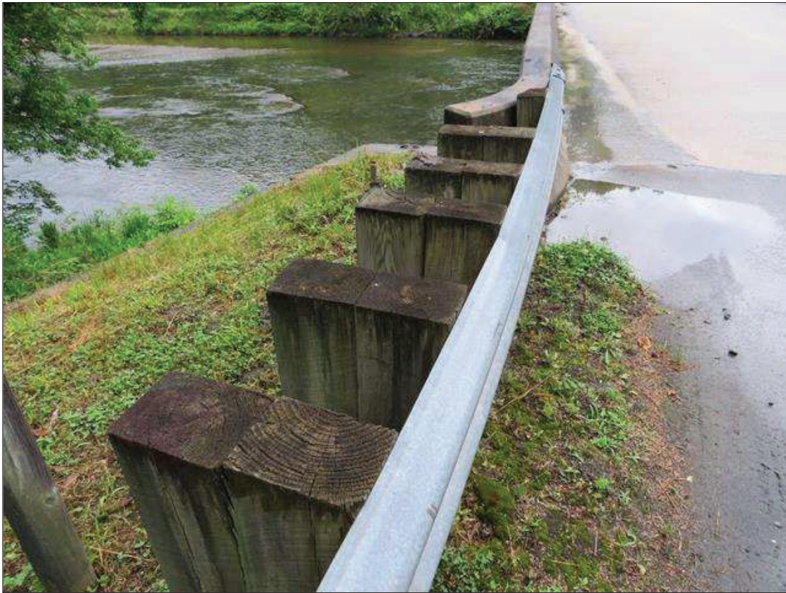
SOUTHWEST CORNER AT BRIDGE 5 POSTS AT 18 INCH CENTERS
