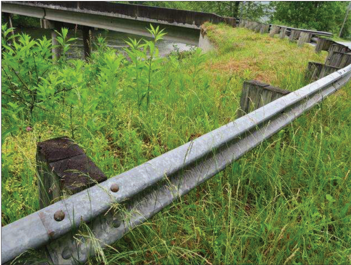
APPROACH GUARDRAIL POST SPACES 75 INCHES AT NORTHEAST CORNER
