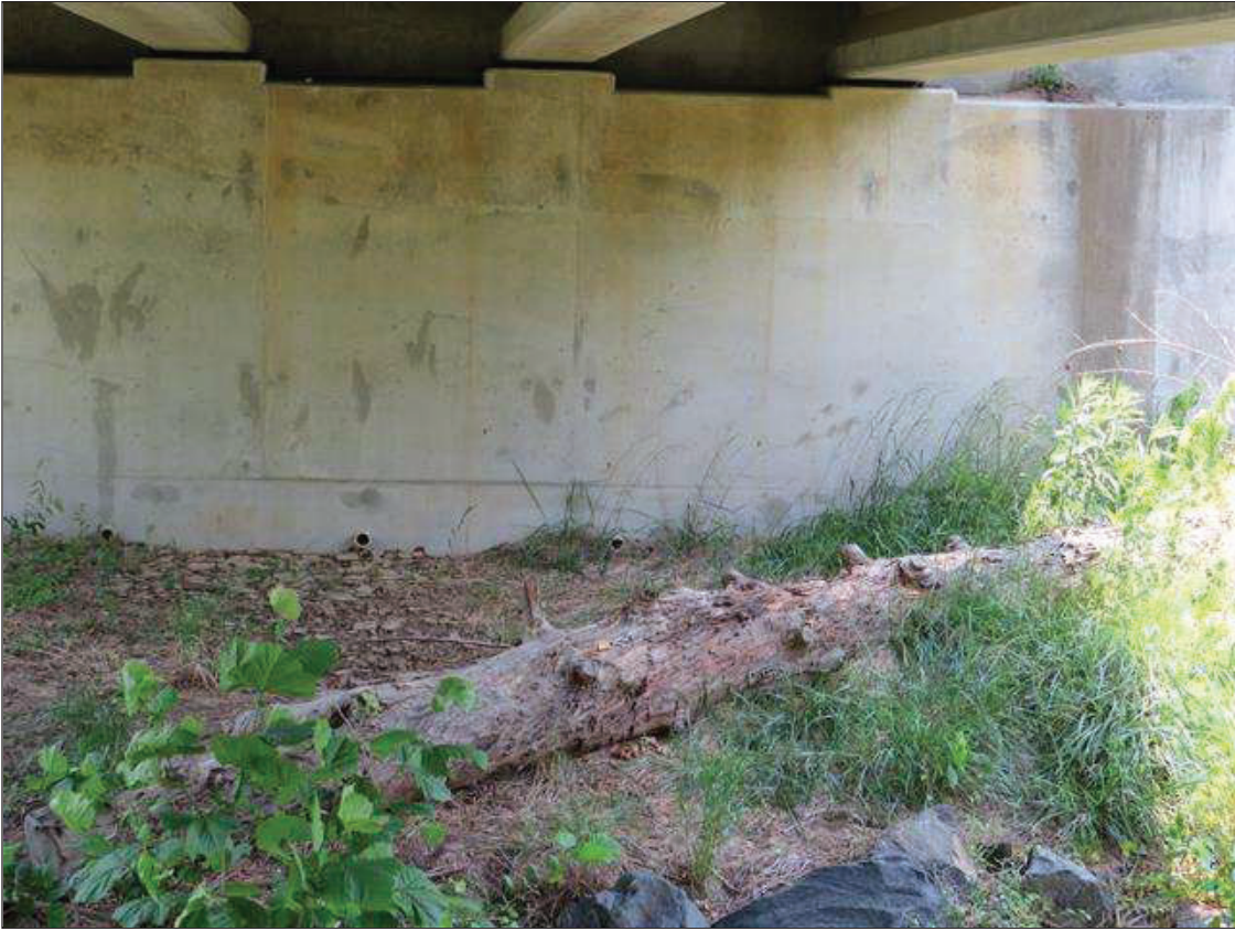
DRIFT (2 FEET DIAMETER) AT END BENT 2 ABUTMENT
