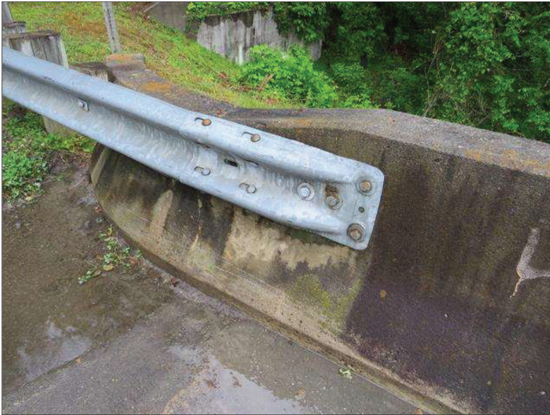
END BENT 1 LEFT SIDE APPROACH GUARDRAIL ATTACHMENT
