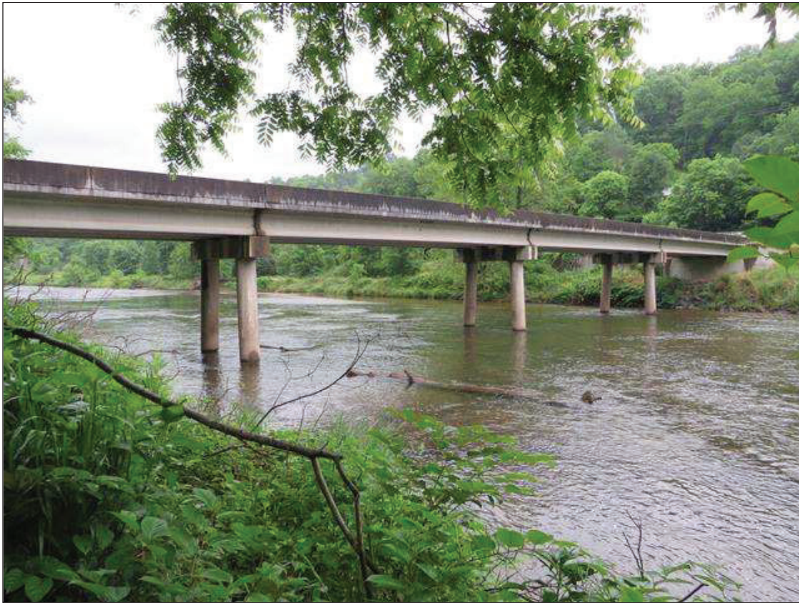
RIGHT SIDE OF BRIDGE LOOKING WEST
