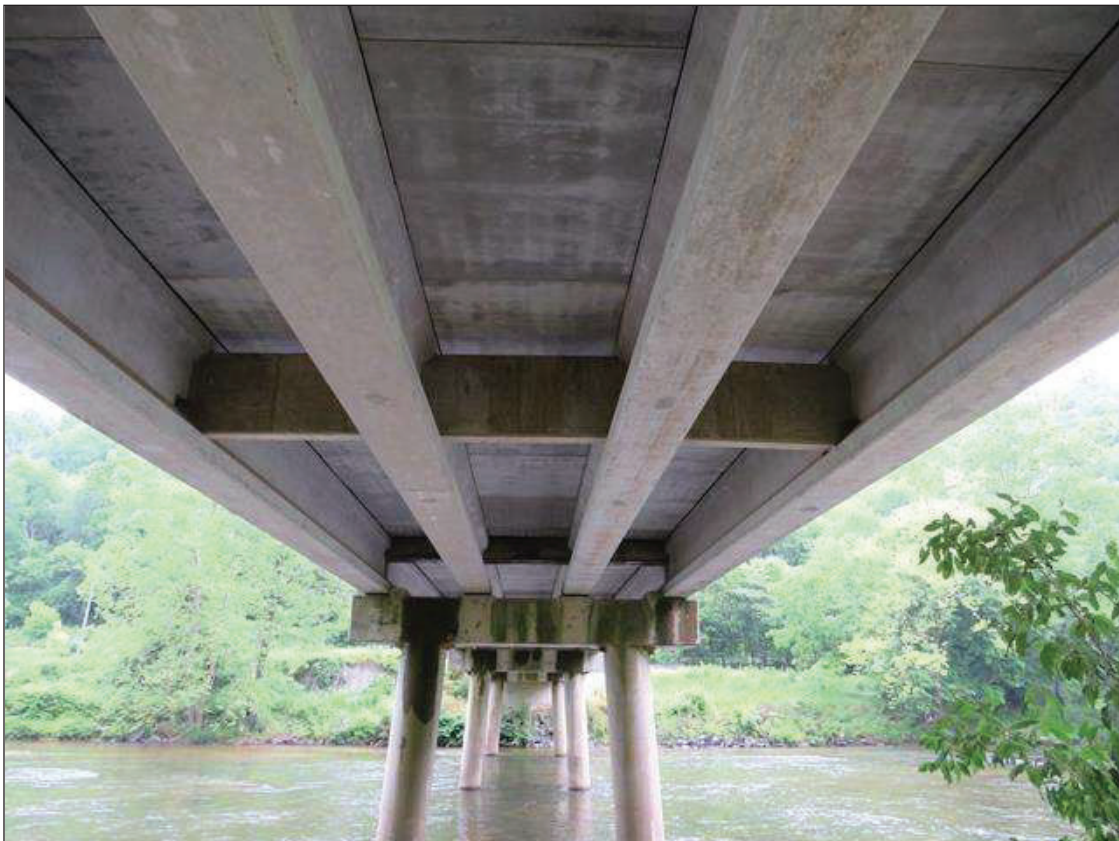
SPAN 1 SUPERSTRUCTURE LOOKING NORTH
