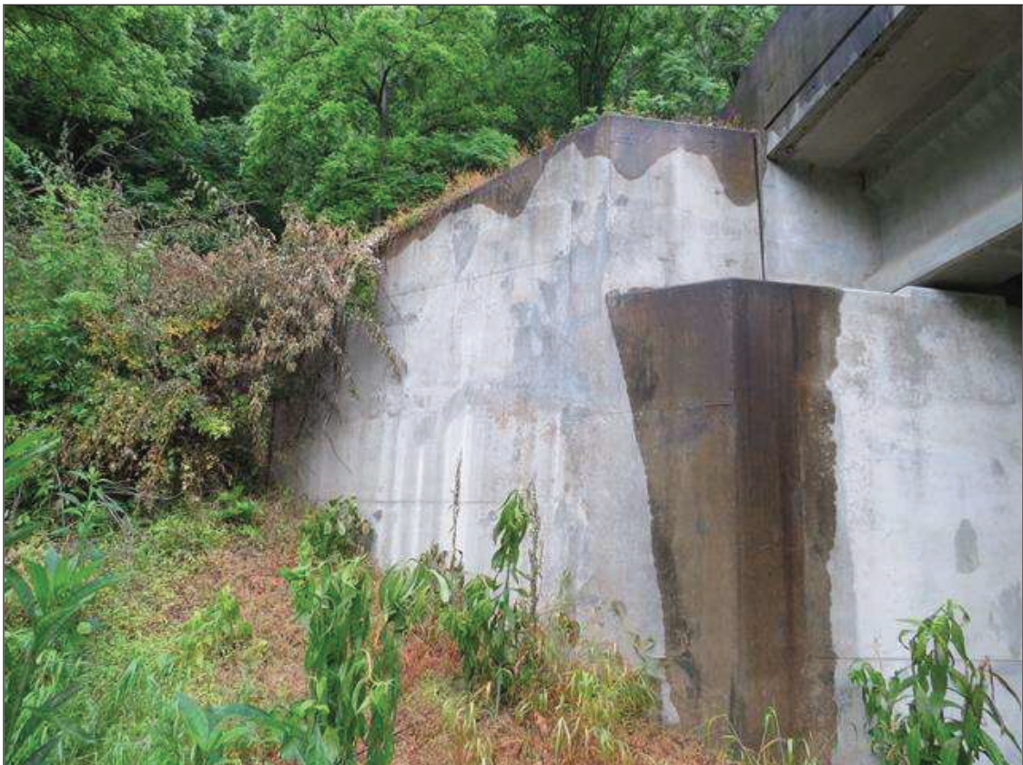
ABUTMENT 1 RIGHT SIDE
