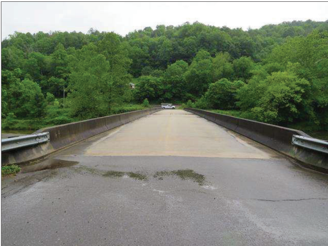
SOUTH APPROACH LOOKING NORTH
