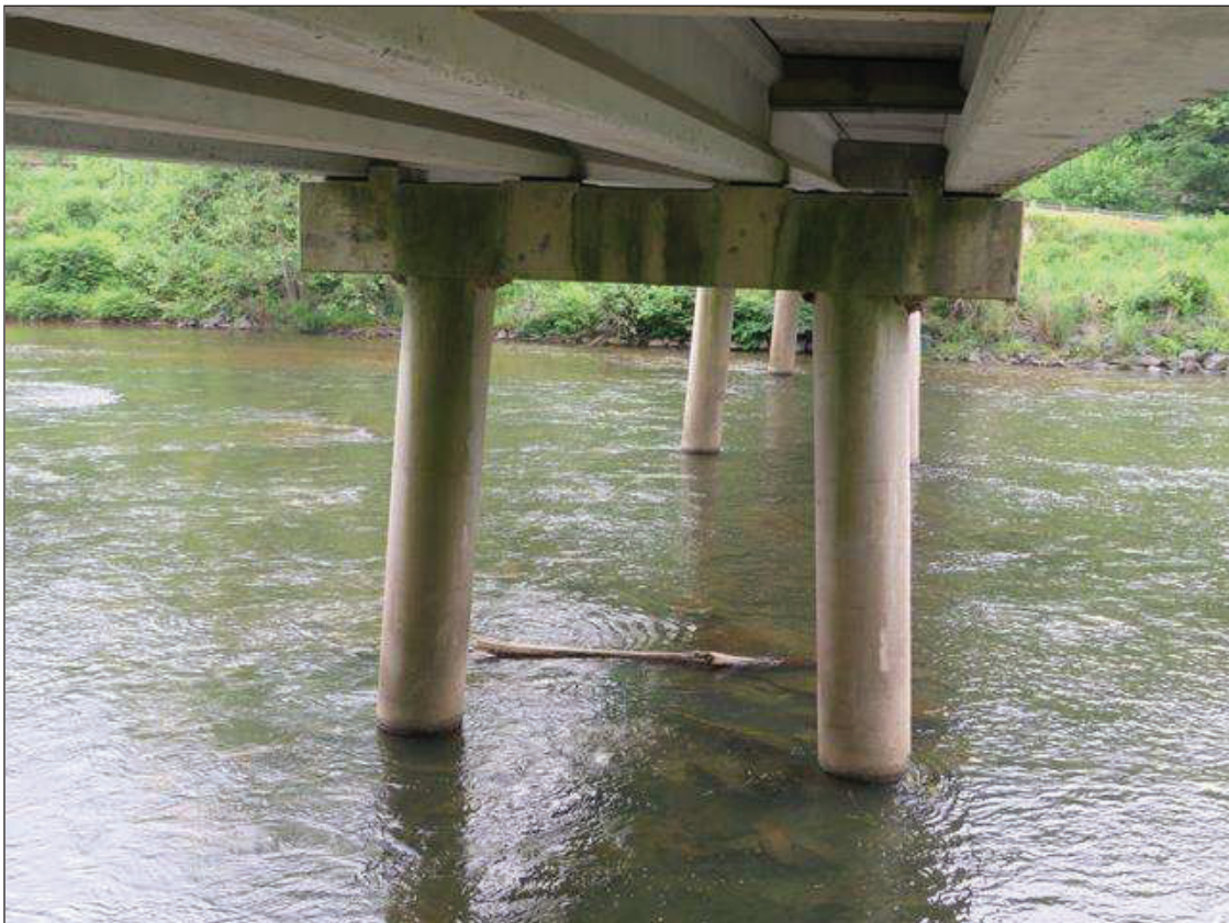
BENT 1 SPAN 1 SIDE
