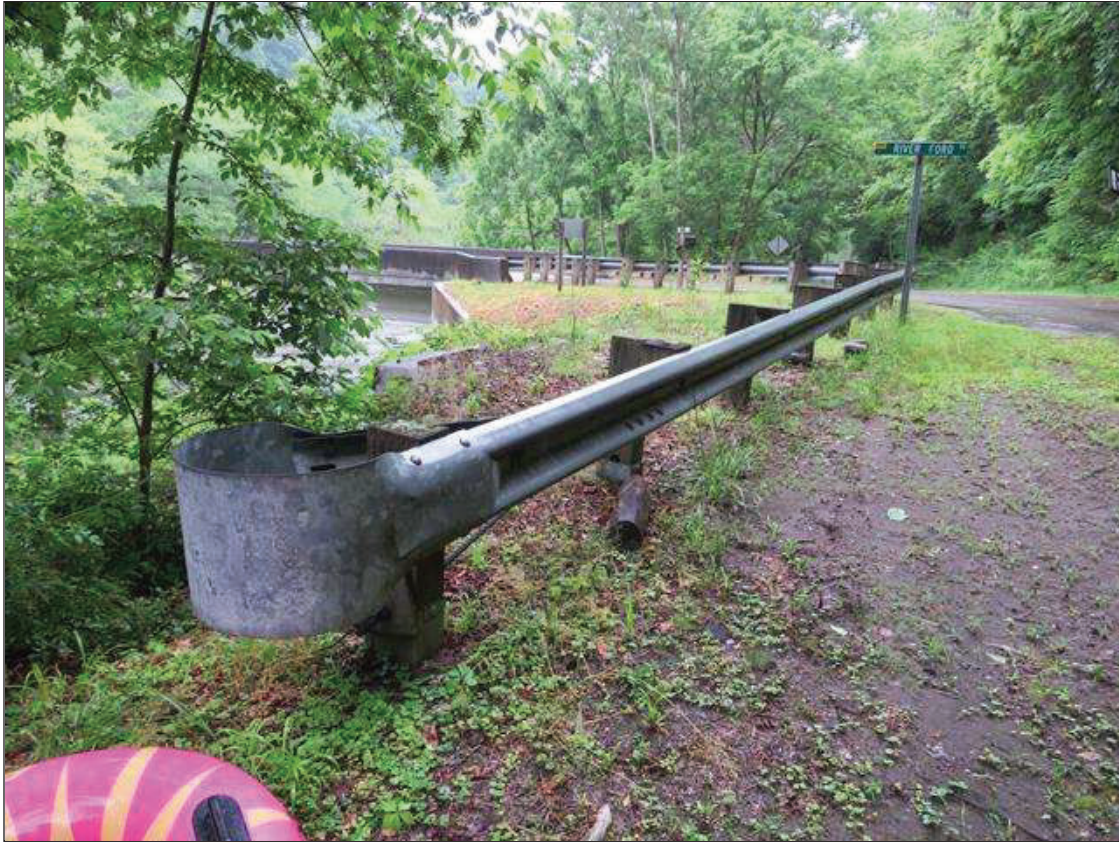
SOUTHWEST GUARDRAIL END TERMINAL
