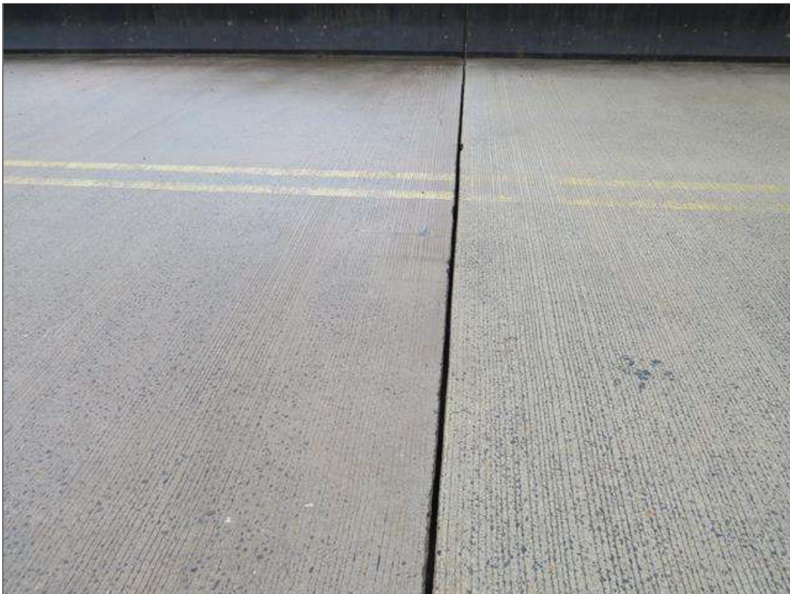
BENT 1 OPEN JOINT
