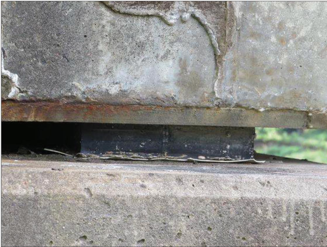
SPAN 2 BEAM 4 NEAR BEARING
