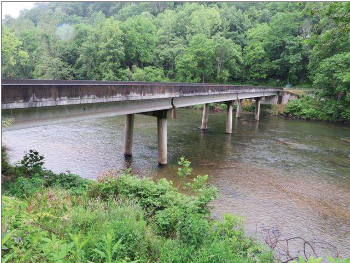
LEFT SIDE OF BRIDGE LOOKING EAST UPSTREAM
