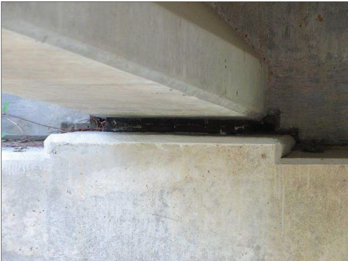
SPAN 1 BEAM 4 FAR BEARING
