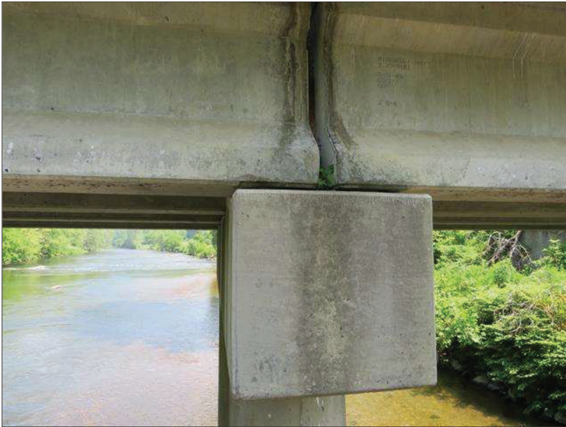
BENT 3 RIGHT SIDE SUPERSTRUCTURE
