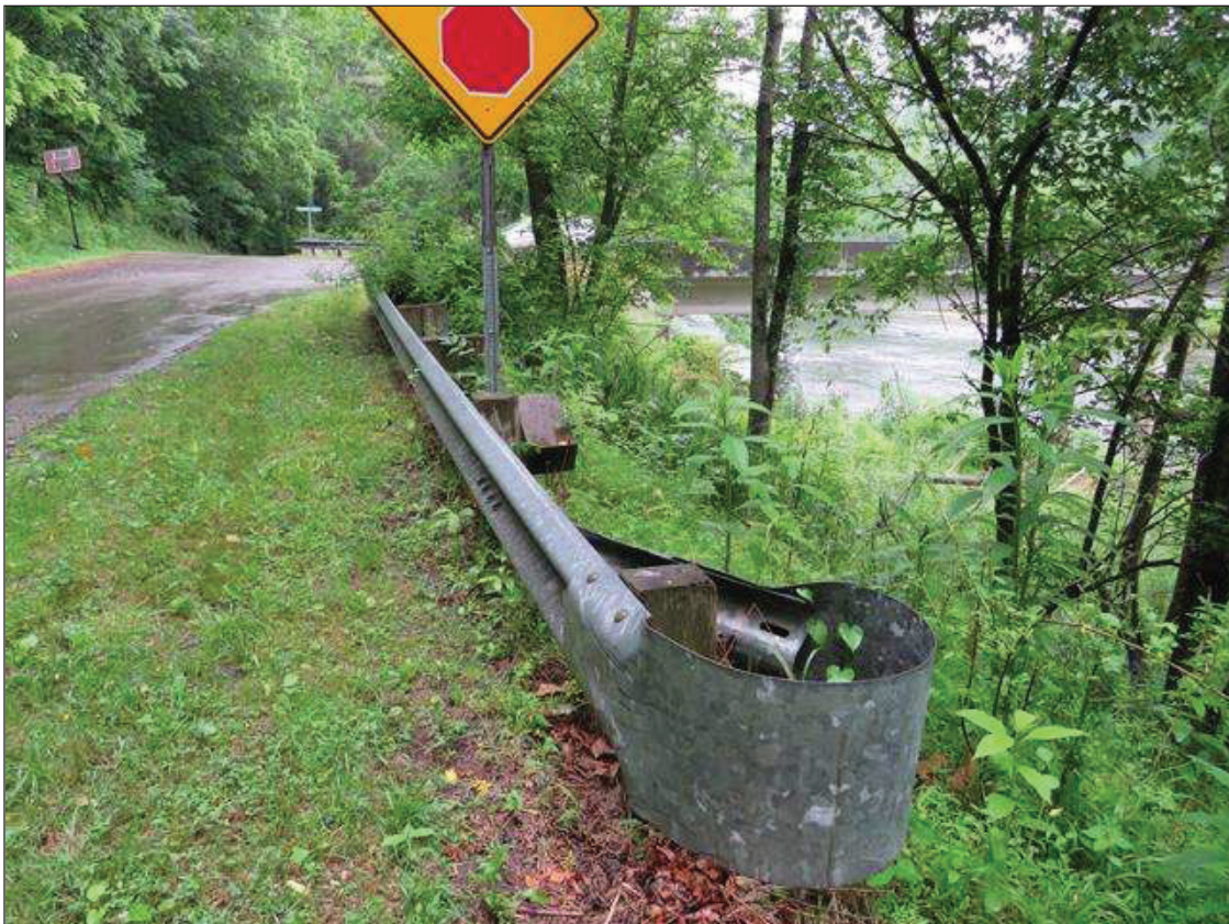
SOUTHEAST GUARDRAIL END TERMINAL
