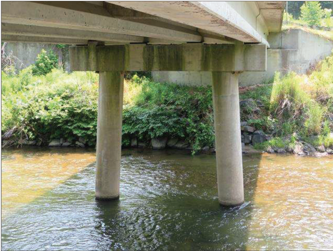
BENT 3 SPAN 3 SIDE
