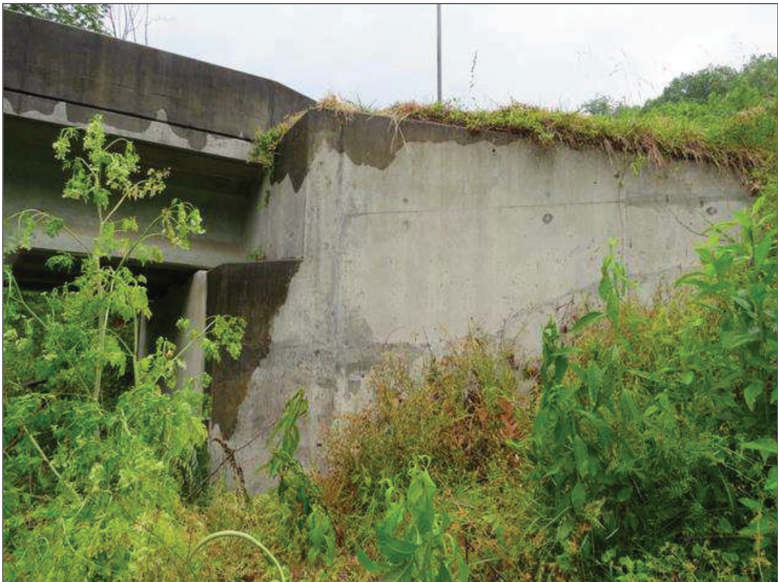
ABUTMENT 2 RIGHT SIDE
