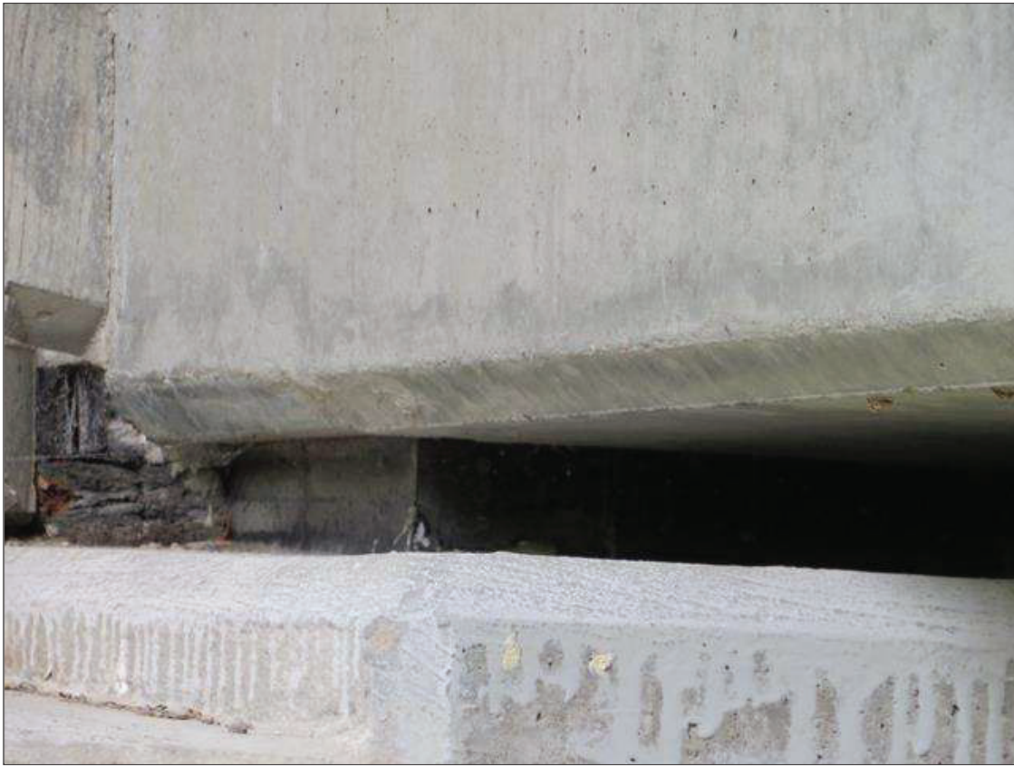
SPAN 1 BEAM 4 NEAR BEARING
