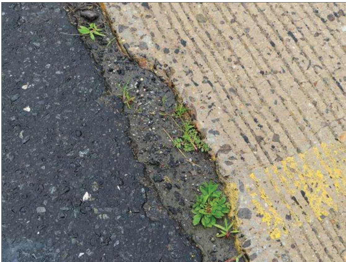
Span 4 Deck: (3) UP TO 12 INCHES WIDE X 1.5 INCHES LONG X 1.5 INCHES DEEP SPALLS ALONG END BENT 2
