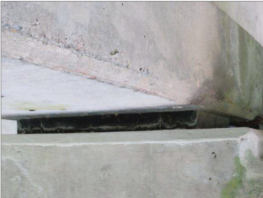
SPAN 3 BEAM 3 FAR BEARING
