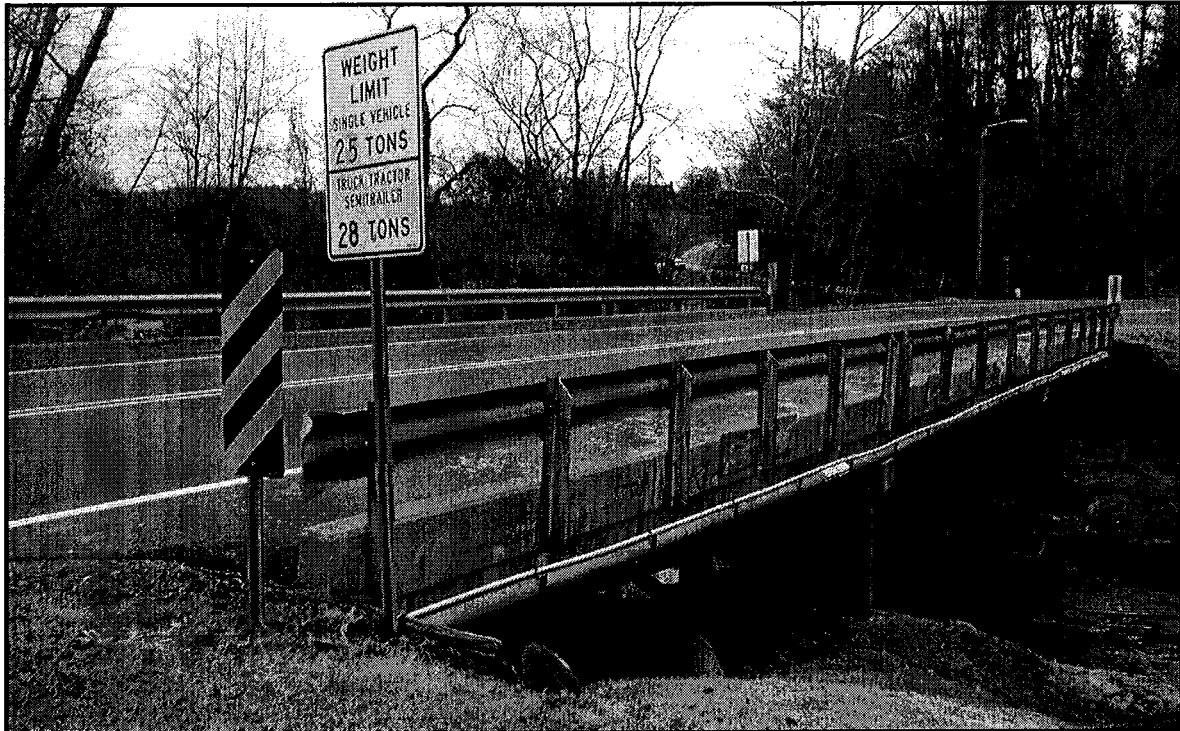
Figure 3. Bridge No 29 over Cub Creek, facing southeast.
