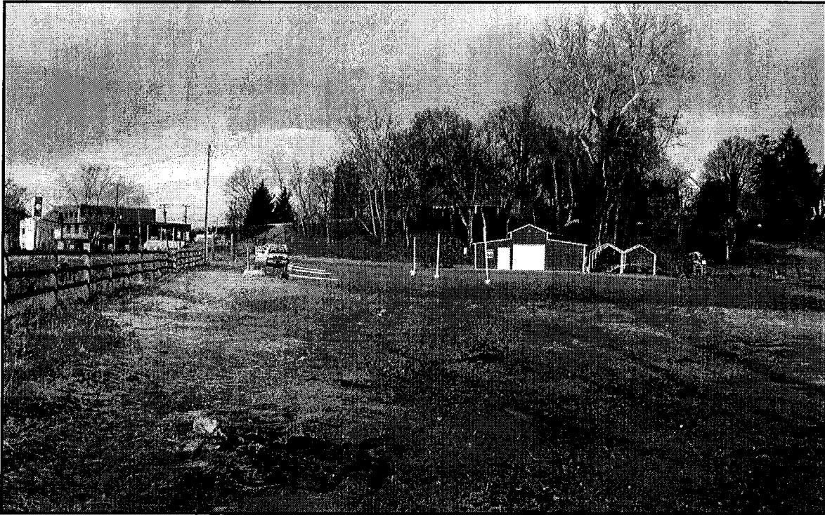
Figure 9. General View of Project Area north of Cub Creek and east of SR 1001 showing nursery parking lot and graded hillslope, facing northwest.
