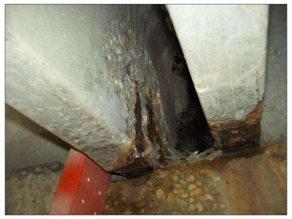
SPAN 1 BENT 1 BEAM 3 LEG 2, SPALL (10IN X 9IN X 1/2IN) WITH EXPOSED RUSTED REBAR
