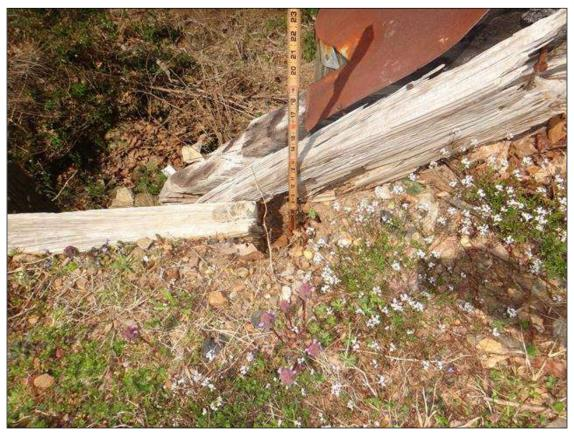
SOUTH APPROACH LEFT SHOULDER, LOSS OF BACKFILL (6IN DIAMETER X 8IN DEEP) WITH SLOPE EROSION (18IN X 18IN X 24IN DEEP)
