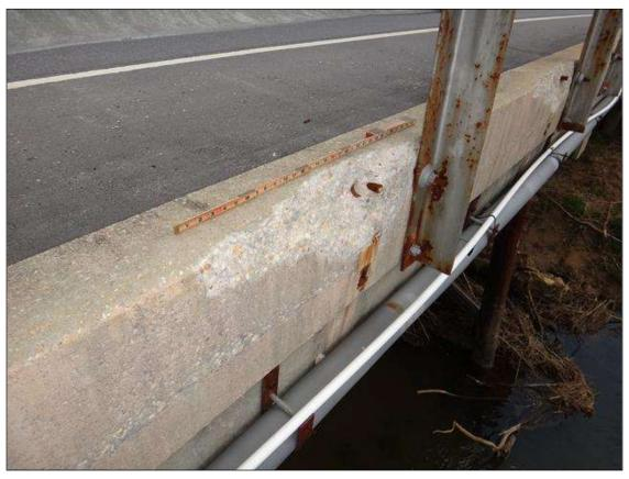
SPAN 2 LEFT PARAPET, SPALL (30IN X 9IN X 2-1/2IN DEEP) WITH EXPOSED RUSTED REBAR AT RAIL POST 3
