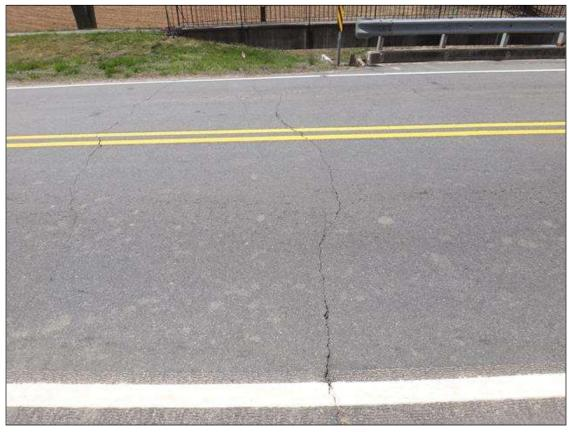
SOUTH APPROACH ASPHALT WEARING SURFACE, MULTIPLE PARTIAL TO FULL WIDTH TRANSVERSE CRACKS (UP TO 1/8IN WIDE)
