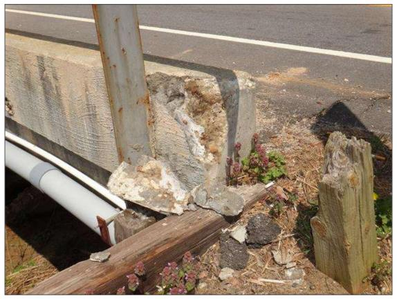
LEFT BARRIER RAIL AT END BENT 1, SPALL (10IN X 12IN X 4IN DEEP)
