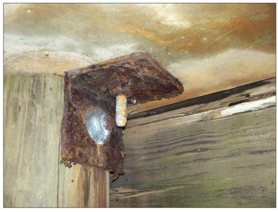
END BENT 1 PILE 6 CONNECTION PLATES, FLAKING STEEL
