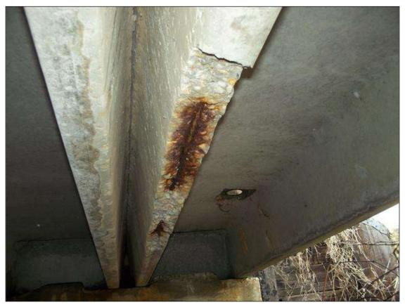
(PM) SPAN 3 BEAM 12 LEG 1 6FT FROM END BENT 2, SPALL (4FT X 2-1/2IN X 1IN) WITH EXPOSED STRAND
