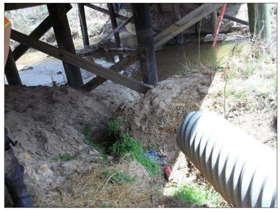
END BENT 2 BANK AT CORRUGATED METAL PIPE OUTLET, EROSION (5FT X 20FT X 4FT DEEP)
