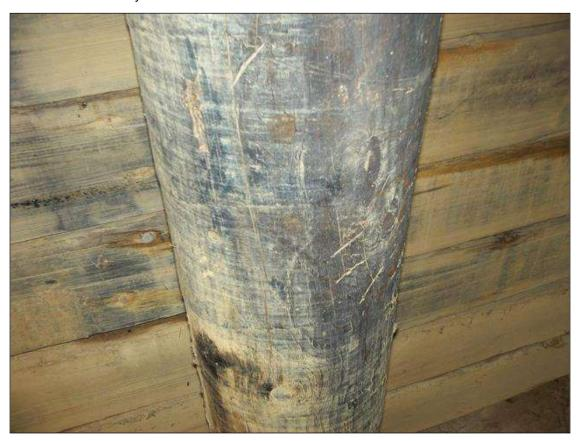
END BENT 1 PILES, CHECKS THROUGHOUT
