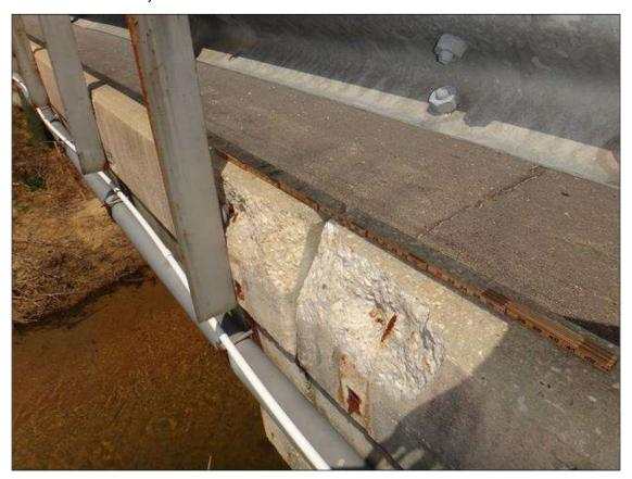
BENT 1 LEFT PARAPET, SPALL (36IN X 10IN X 4IN DEEP) WITH EXPOSED RUSTED REBAR
