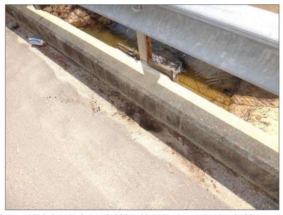
SPAN 2 LEFT SHOULDER, ONE (1) CLOGGED SCUPPER DRAIN WITH DEBRIS ACCUMULATION
