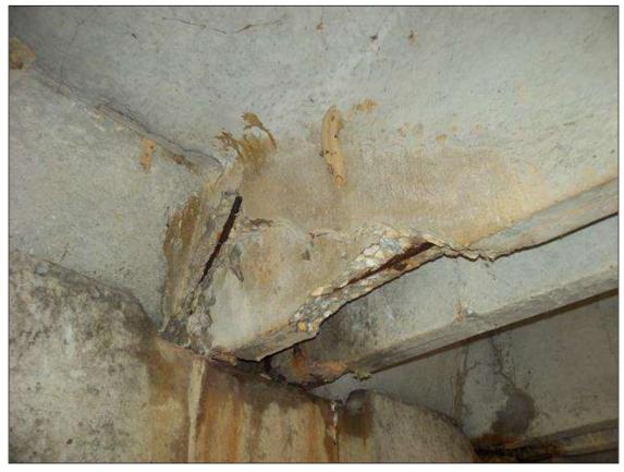
(PM) BENT 1 BEAM 1 LEG 2, SPALL/DELAMINATION (18IN X 8IN) WITH EXPOSED STRAND
