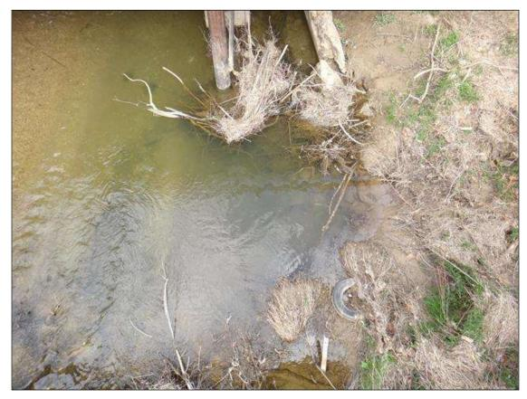
STREAMBED AT BENT 1, SCOUR HOLE (10FT X 15FT X 3FT DEEP)
