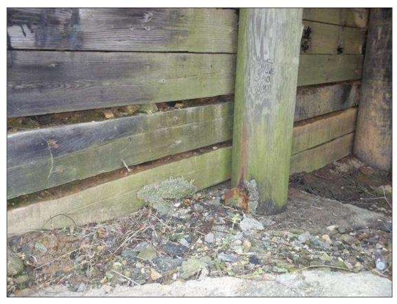
(PM) END BENT 1 BULKHEAD, GAPS IN BOARDS WITH BACKFILL LOSS (20LF)
