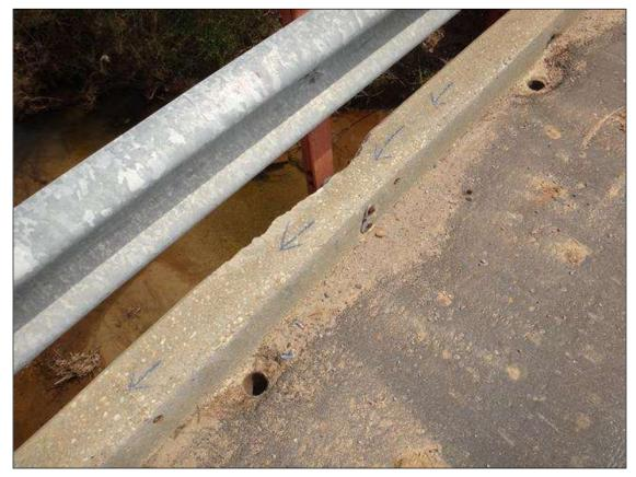
SPAN 1 RIGHT PARAPET, FOUR (4) FULL WIDTH HAIRLINE CRACKS IN PARAPET AT RAIL POST 5
