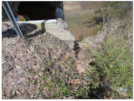
SOUTH APPROACH RIGHT SHOULDER, SLOPE EROSION BEHIND WINGWALL (2FT X 6FT X 1FT DEEP)
