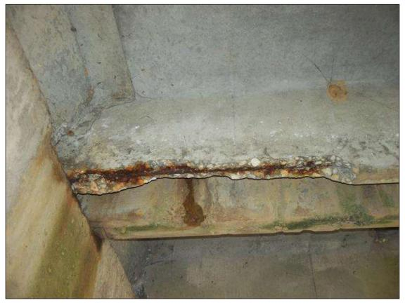
(PM) BENT 2 SPAN 2 BEAM 11 LEG 2 BEARING, SPALL (2FT X 2-1/2IN X 2IN) WITH EXPOSED STRAND
