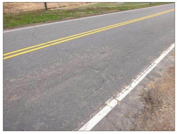
NORTH APPROACH NORTHBOUND LANE, BROKEN AND DEPRESSED ASPHALT (50FT X 4FT WIDE) WITH FULL WIDTH TRANSVERSE CRACK
