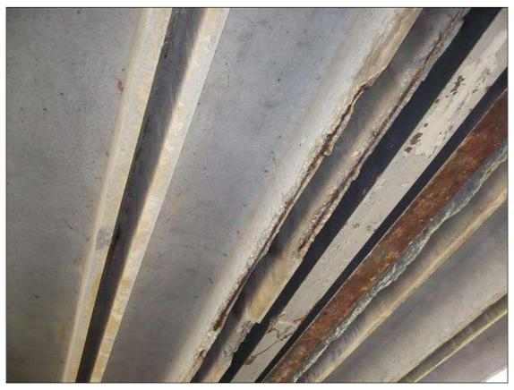
(PM) SPAN 2 BEAM 9 LEG 2 MID SPAN, SPALL (9-1/2FT) WITH EXPOSED STRAND
