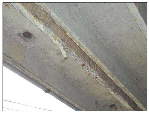
(PM) SPAN 2 BEAM 1 LEG 2 10FT FROM BENT 2, SPALL (10FT X 2-1/2IN X 1IN) WITH FAILED REPAIR
