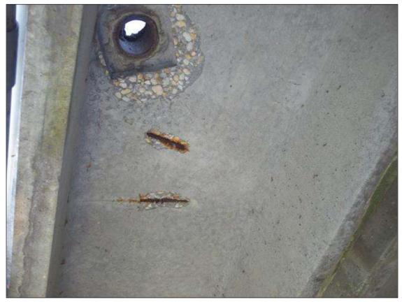
SPAN 1 BEAM 1 NEAR END BENT 1, TWO (2) EXPOSED RUSTED REBAR (8IN)
