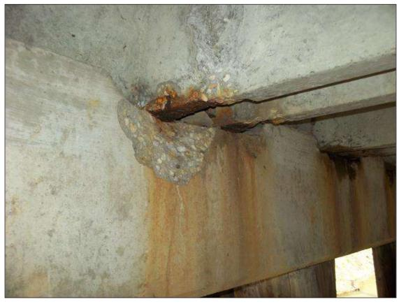
SPAN 1 BENT 1 CAP UNDER BEAM 4 BEARING, SPALL (10IN X 5IN X 1IN)
