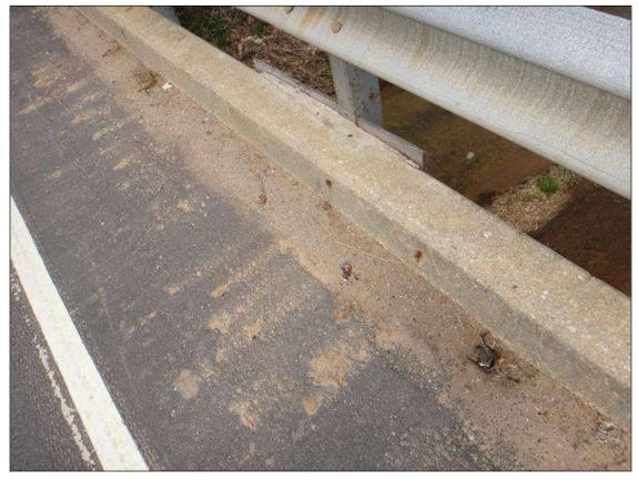
SPAN 2 RIGHT SHOULDER, THREE (3) CLOGGED SCUPPER DRAINS AND DEBRIS ACCUMULATION
