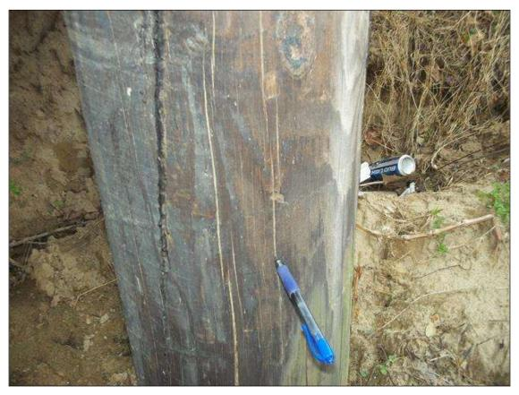
BENT 2 PILES AND BRACING, CHECKS THROUGHOUT
