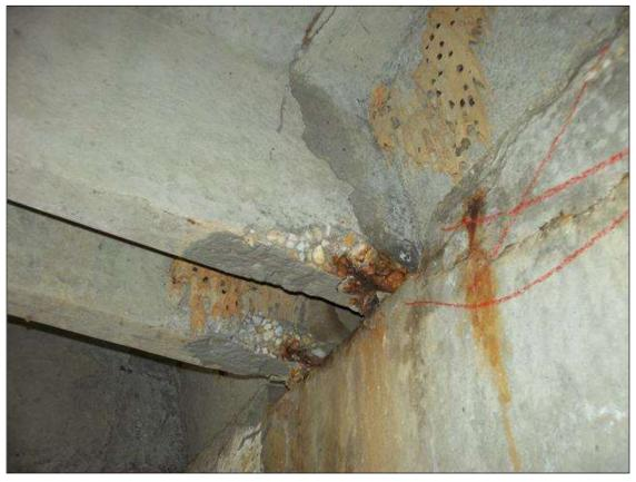
SPAN 2 BENT 2 BEAM 5 LEG 1, FAILED SPALL REPAIR AT BEARING (5IN X 2IN X 1/2IN) (SIMILAR BEAM 6,7)
