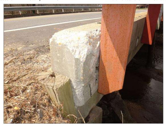
END BENT 1 RIGHT PARAPET, SPALL AT RAIL CONNECTION AND END
