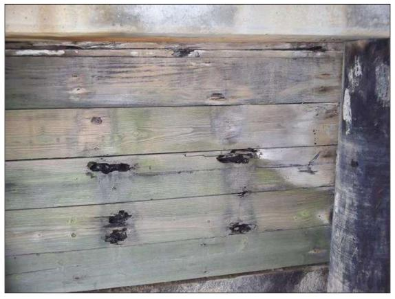
END BENT 1 BULKHEAD BAY 5, SIX (6) DECAYED AREAS (8IN DIAMETER)
