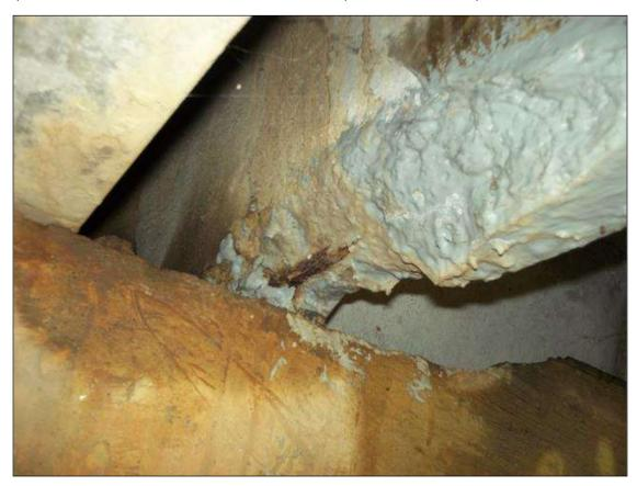
(PM) END BENT 2 BEAM 11 LEG 1 BEARING, SPALL (9IN X 2-1/2IN X 2IN) WITH EXPOSED STRAND
