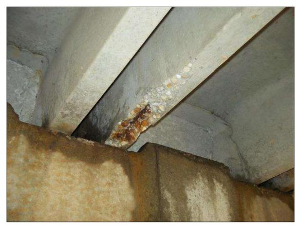
(PM) END BENT 1 BEAM 1 LEG 2 BEARING, SPALL (12IN X 2-1/2IN X 2IN) WITH EXPOSED STRAND
