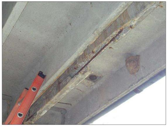
(PM) BENT 1 SPAN 2 BEAM 1 LEG 2, SPALL (9FT X 2-1/2IN X 5IN) WITH EXPOSED STRAND
