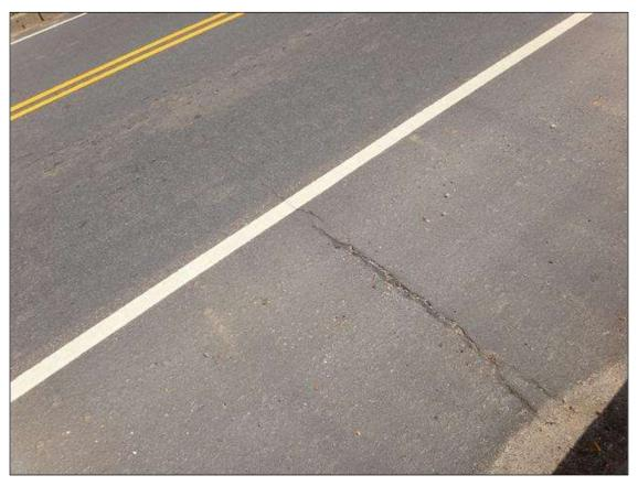
SOUTHBOUND LANE ASPHALT WEARING SURFACE AT BENT 2, TRANSVERSE CRACK (12FT X UP TO 1/8IN WIDE)
