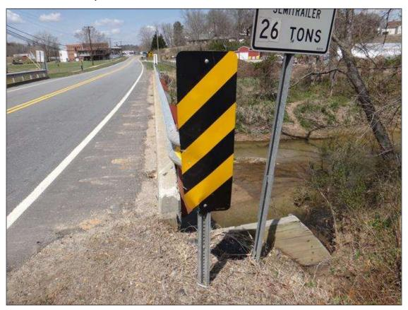
SOUTH APPROACH RIGHT SHOULDER, IMPACT DAMAGE TO DELINEATOR
