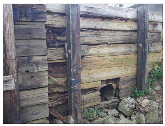
(PM) SOUTHWEST WINGWALL, DECAY (80%) WITH BACKFILL LOSS (36SF)
