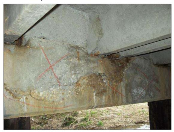
BENT 2 CAP NORTH FACE AT BEAM 5, SPALL/DELAMINATION (7FT X 16IN)
