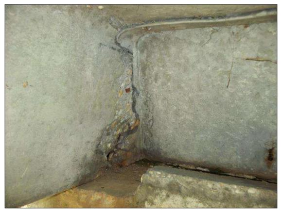
(PM) END BENT 2 BEAM 1 LEG 1 BEARING, SPALL (7IN X 6IN X 2-1/2IN) 1IN BEARING REMAINING
