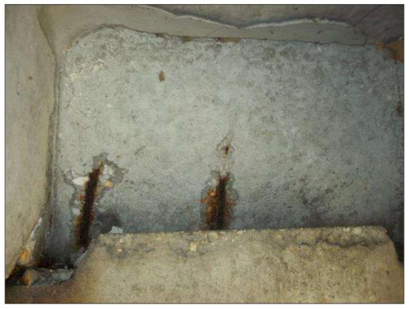
SPAN 2 BENT 1 BAY 5 END DIAPHRAGM, EXPOSED RUSTED REBAR
