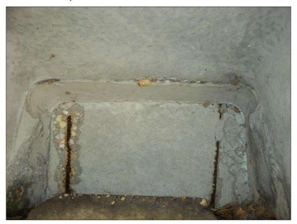
END BENT 1 END DIAPHRAGM BAY 2, SPALL WITH EXPOSED RUSTED REBAR (1SF)
