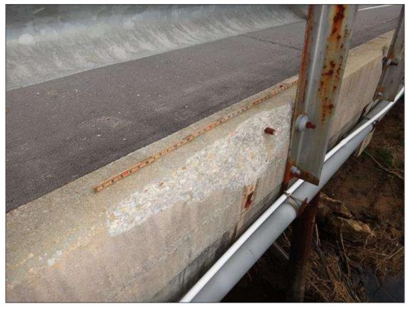
SPAN 2 LEFT PARAPET, SPALL (38IN X 9IN X 2-3/4IN DEEP) WITH EXPOSED RUSTED REBAR
