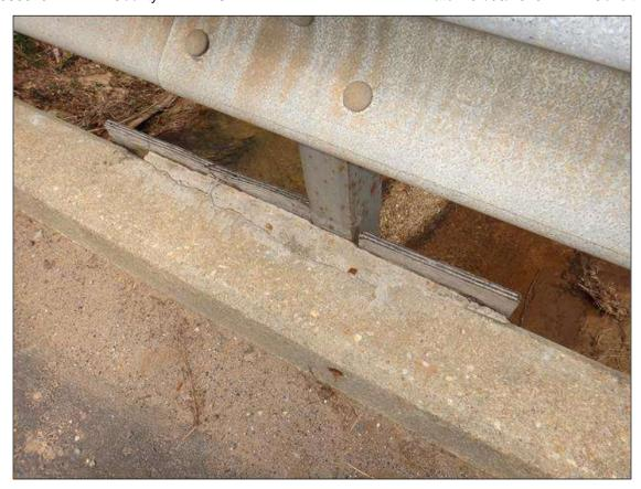
SPAN 2 RIGHT PARAPET, FAILED REPAIR AT RAIL POST 2 CONNECTION
