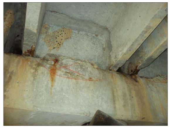
BENT 2 CAP SOUTH FACE UNDER BEAM 5, DELAMINATION (18IN X 7IN) (SIMILAR BEAM 6)
