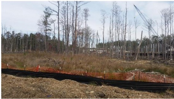
1. Swamp Forest looking east. Silt fencing has been placed around the wetland boundary
