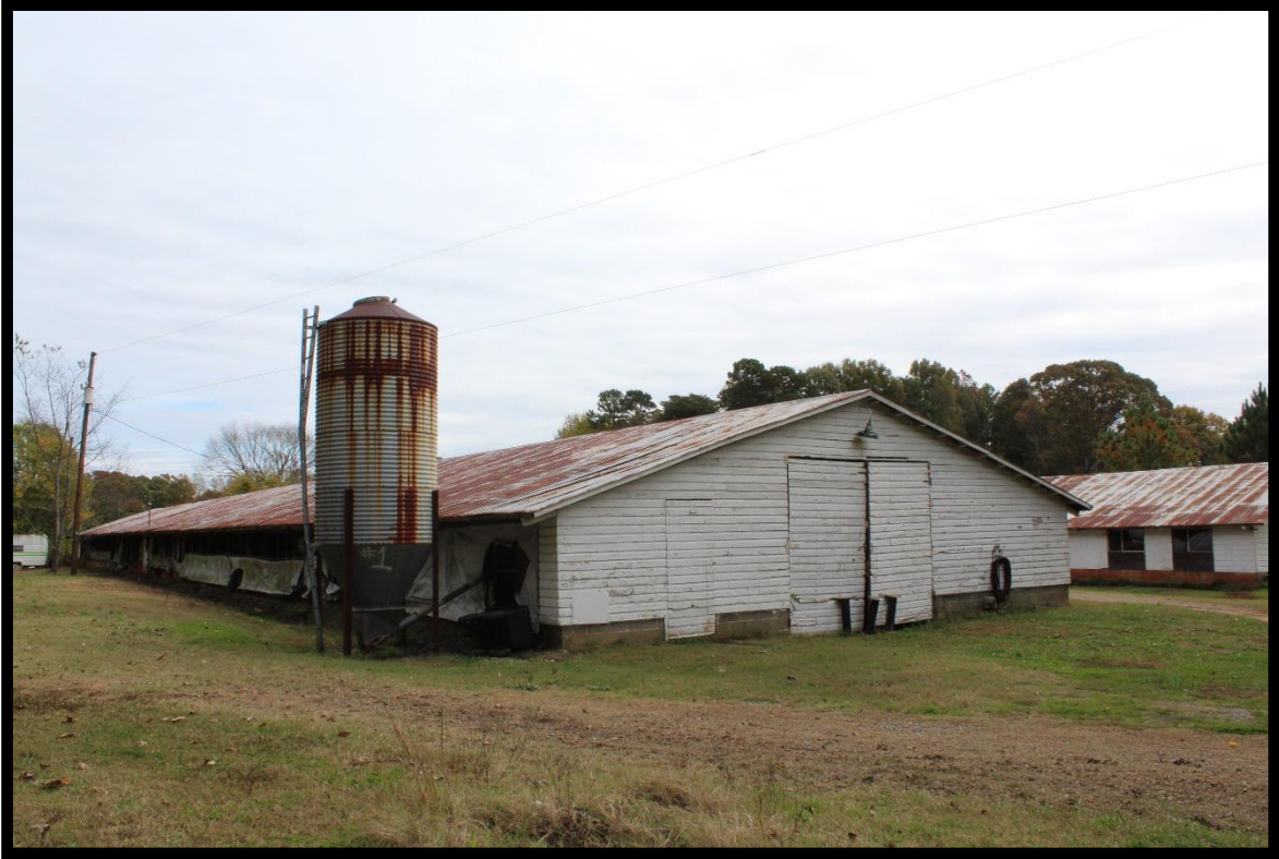
Figure 19: Chester Farmstead, Poultry Shed, Looking Southeast.
