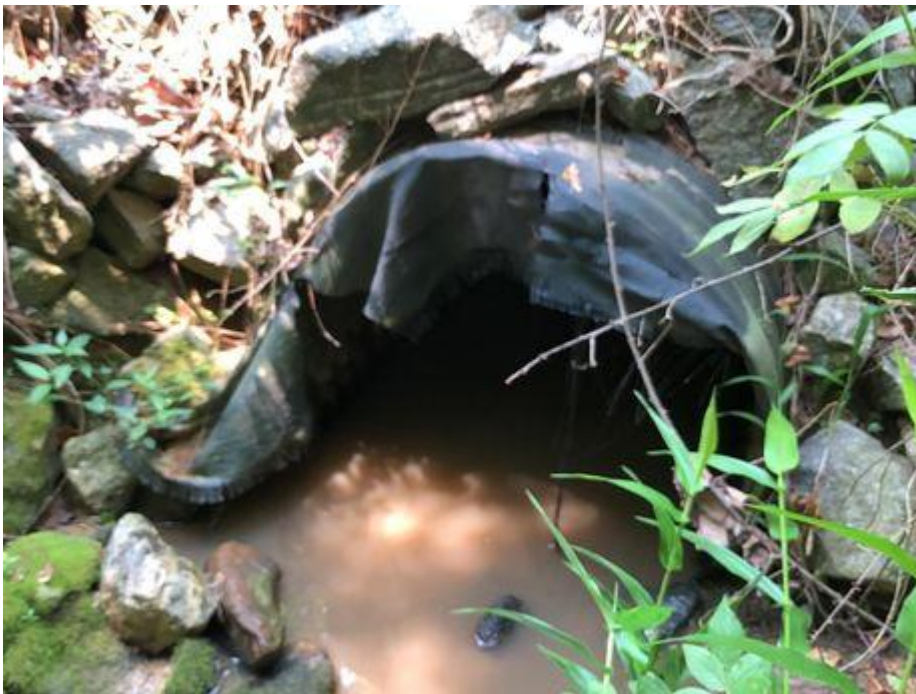
Culvert Photo: Photo Caption: Outlet
