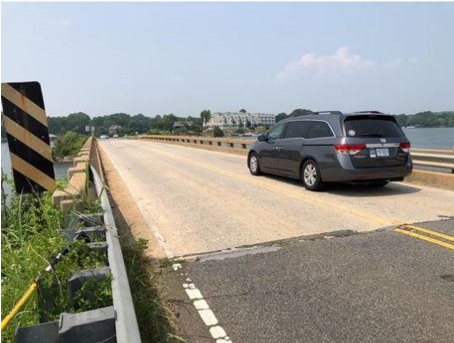
Photo Caption: Looking west
