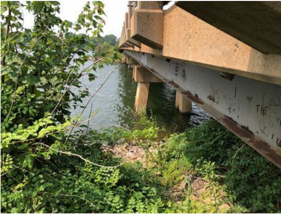
Photo Caption: Looking west
