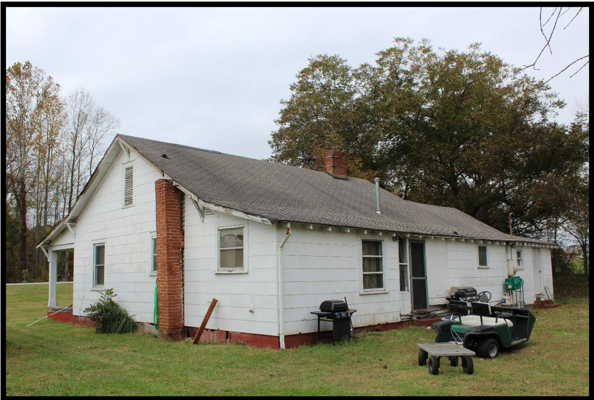
Figure 8: Chester Farmstead, Original Dwelling, Looking Northwest.
