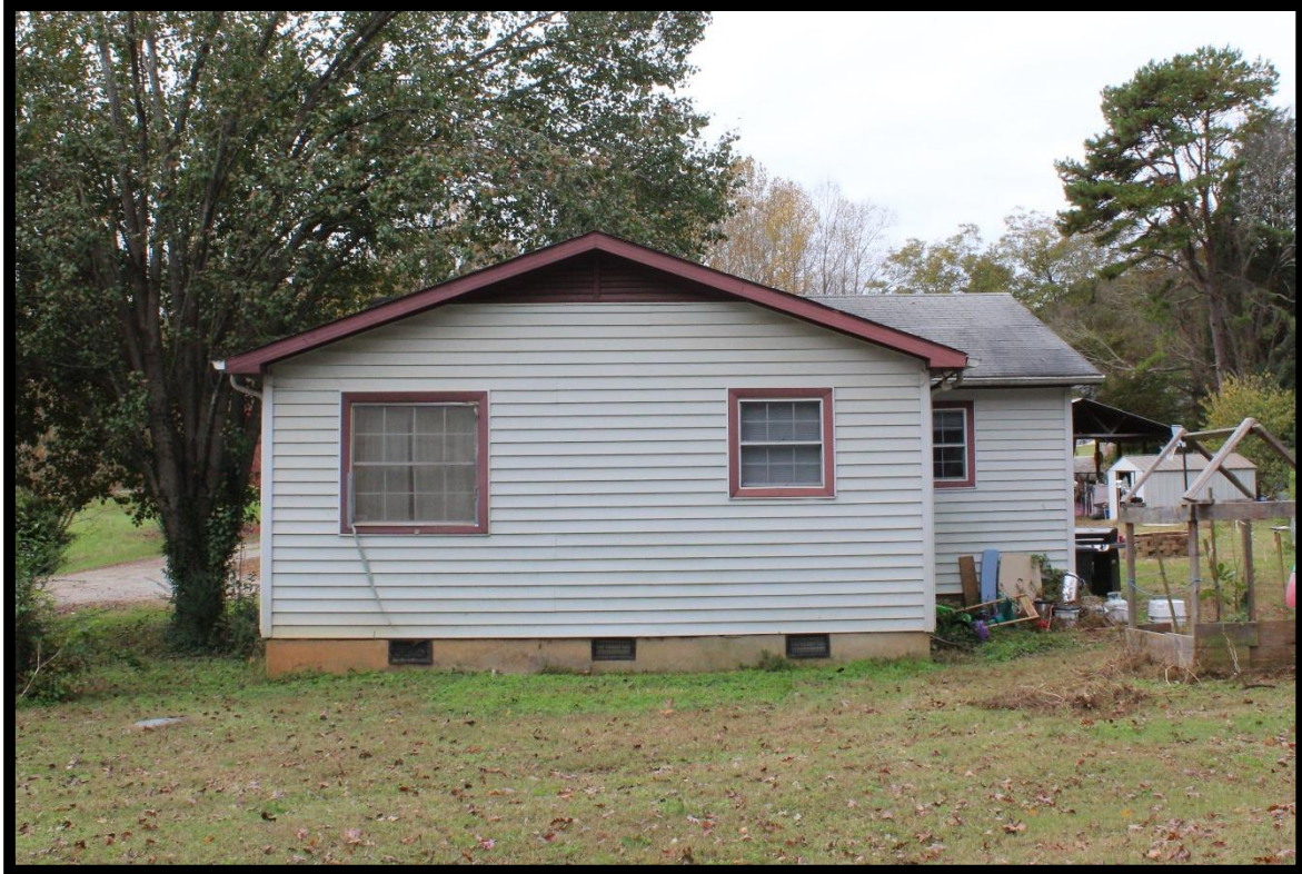
Figure 12: Chester Farmstead, Second Dwelling, Looking West.
