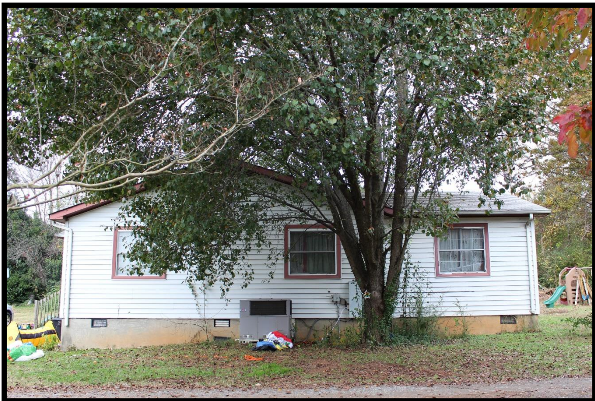
Figure 13: Chester Farmstead, Second Dwelling, Looking North.
