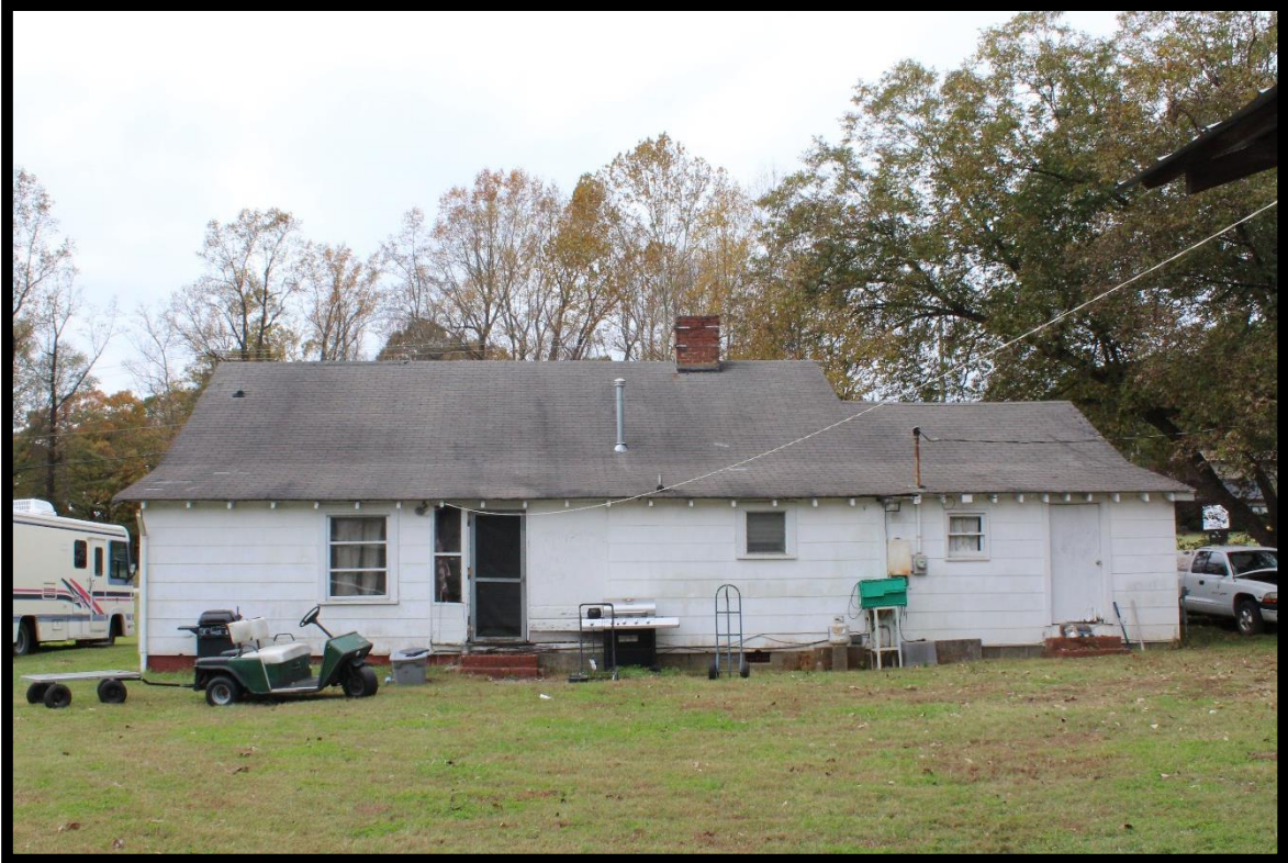
Figure 7: Chester Farmstead, Original Dwelling, Looking West.
