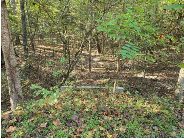
Fig.1: Looking upstream of the existing 60" at SGR and WIP. The 60" Headwall is visible in the picture
