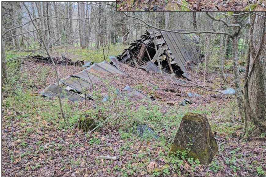
B. Facing East at Feature 101
