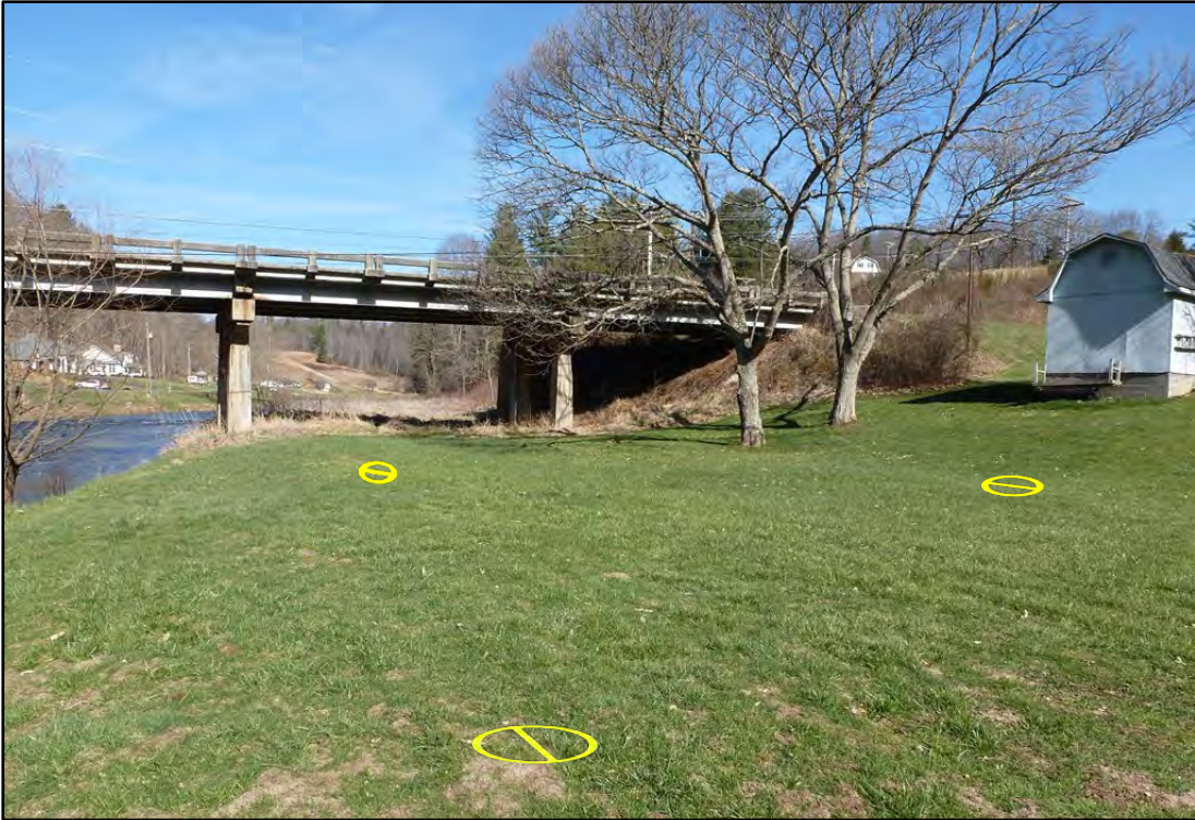
Figure 6: Northwest view of the northeast quadrant.
