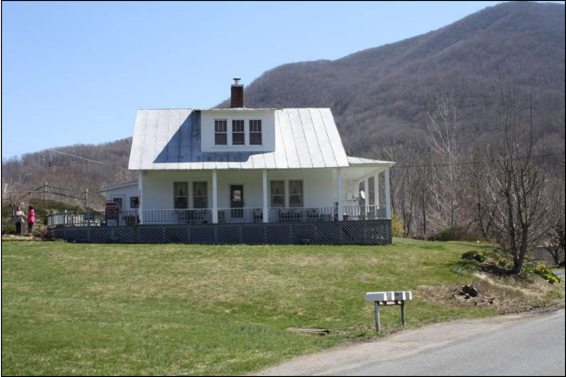
Figure 3: South (front) elevation
