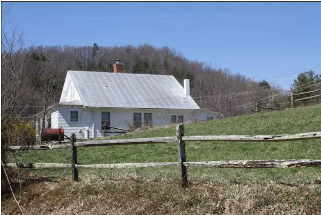
Figure 6: North (rear) elevation
