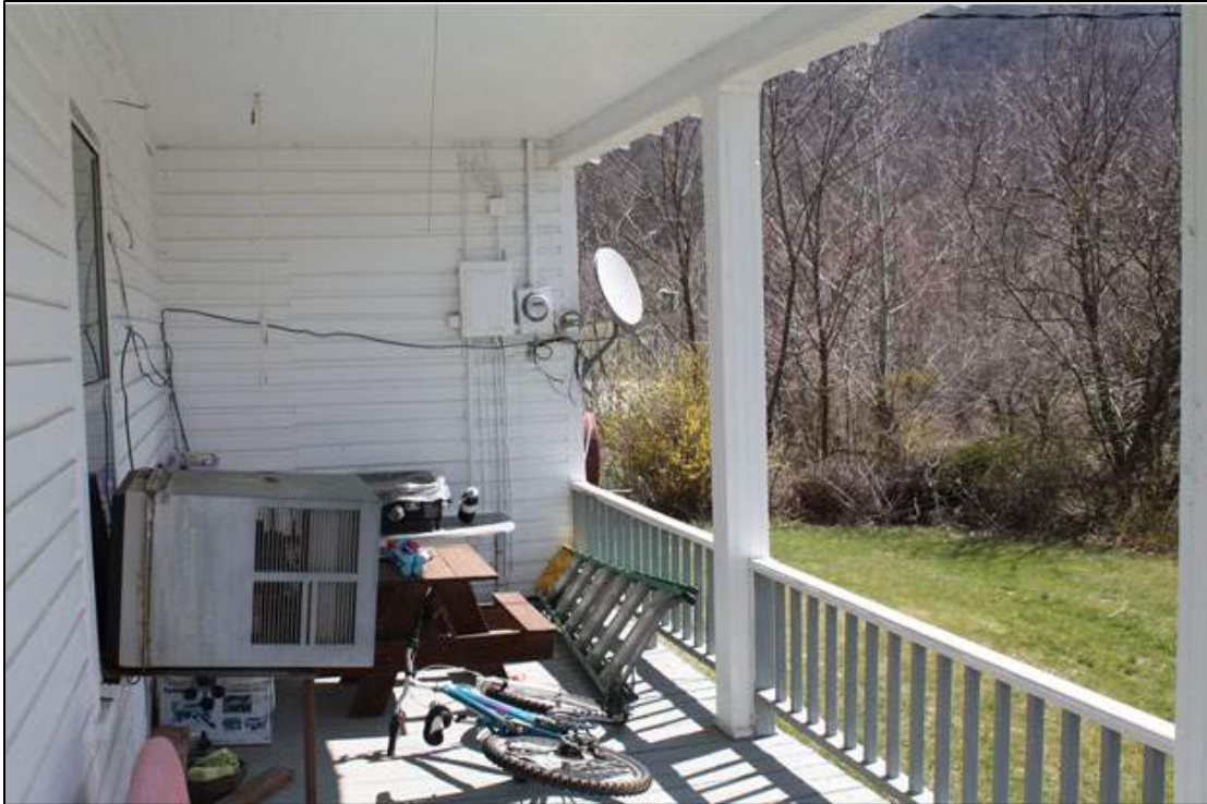
Figure 5: Looking north on the front porch. An area of patched siding can be seen on the far wall where a door was once present.
