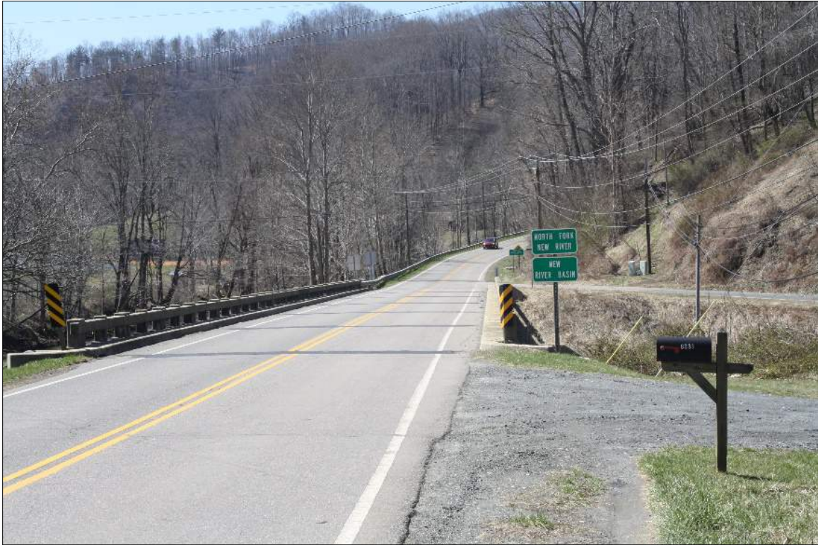
Figure 13: Looking south along NC HWY 194 across North Fork New River Bridge. The Thompson-Barr House is due east of the photographer's location.
