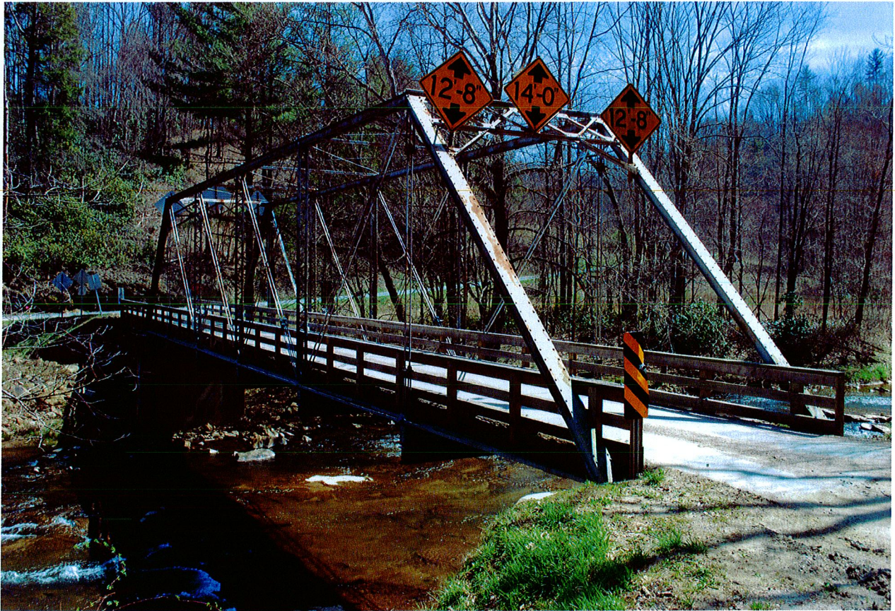
Avery County Bridge No. 125 (AV0125)
