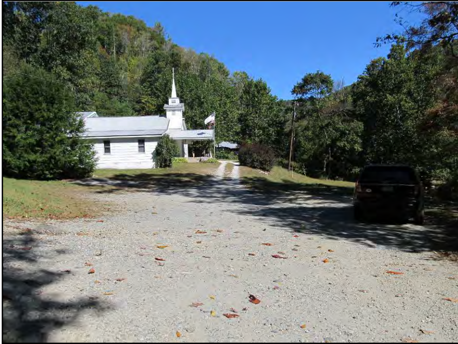
Figure 11. View of church, gravel parking area, and driveway in the northwest quadrant, looking north.
