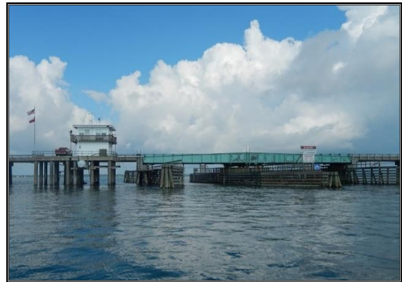
Facing west toward the existing Harkers Island Bridge
