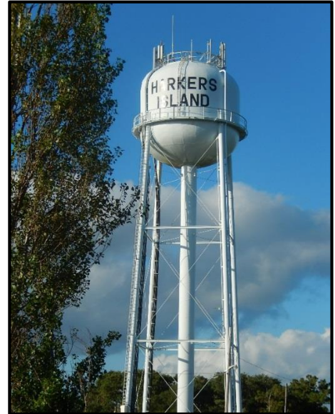
Harkers Island Water Tower
