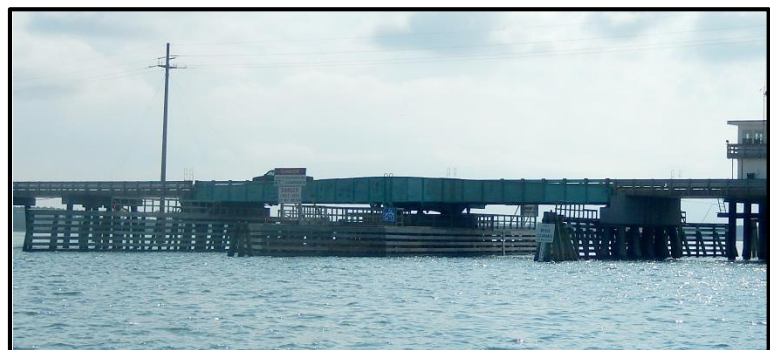
Bridge fender structures
