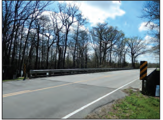
Bridge 139 approach facing SE direction toward Biddle Rd
