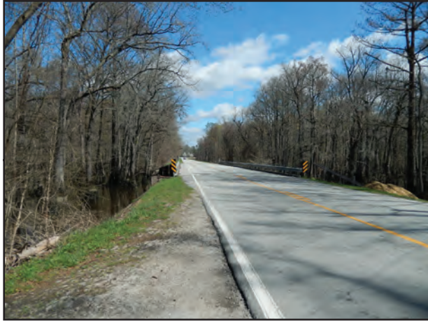
Bridge 138 approach facing NE direction toward SR 1450 (Nelson Rd)
