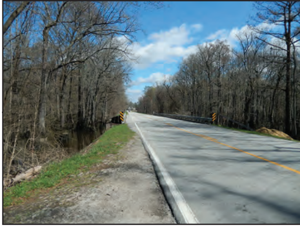
Bridge 139 approach facing NW direction toward SR 1450 (Nelson Rd)
