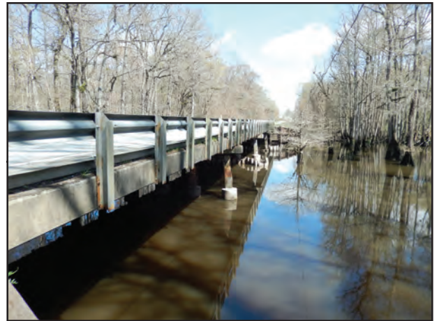
West side of Bridge
