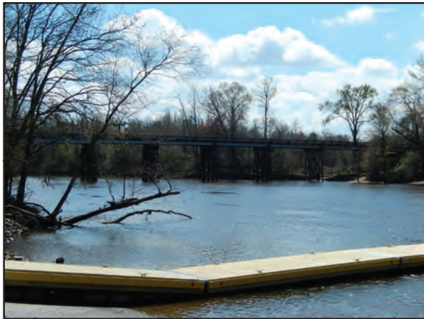
West side of Bridge 138 from Boat Launch site
