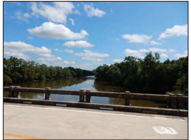
East side of Bridge 138
