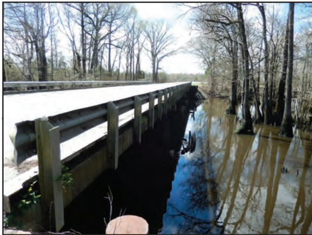
East side of Bridge
