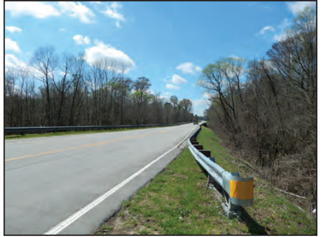
Bridge 138 approach facing SW direction toward Biddle Rd
