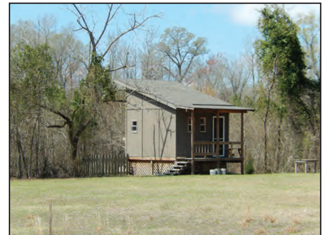
Abandoned Shack northeast of Bridge 138 (south of abandoned house)
