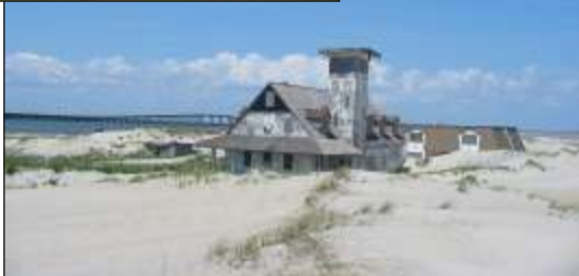
Former Coast Guard Station at Oregon Inlet
