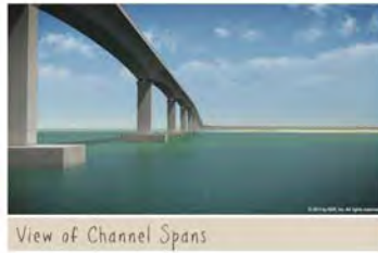
View of Channel Spans
