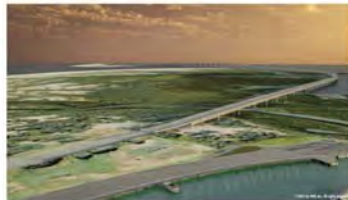
New Bridge (looking south)
