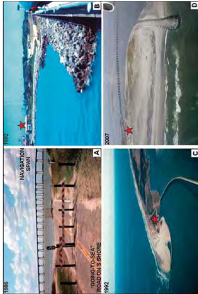
Figure 19. (A) 1986 photograph shows the Oregon Inlet bridge and the rapidly "going-to-the-sea" road on the south shore resulting from the southward migration of Oregon Inlet. (B) 1992 photograph shows the rock revetment built in 1989–1991 around the south end of the bridge to secure it to Pea Island. (C) 1992 oblique aerial photograph shows the north end of Pea Island secured by the rock jetty and rock revetment. (D) Oblique aerial photograph shows of the seaward end of the terminal jetty and the sand-filled inlet. The red stars in B–D indicate the location of the old U.S. Coast Guard Station and the approximate Oregon Inlet shoreline prior to construction of the jetty and revetment. Photographs are by S.R. Riggs.
