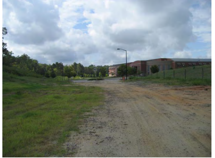
Figure 2: Village Point Access Road Facing South Terminus at Village Point Drive Traffic Circle
