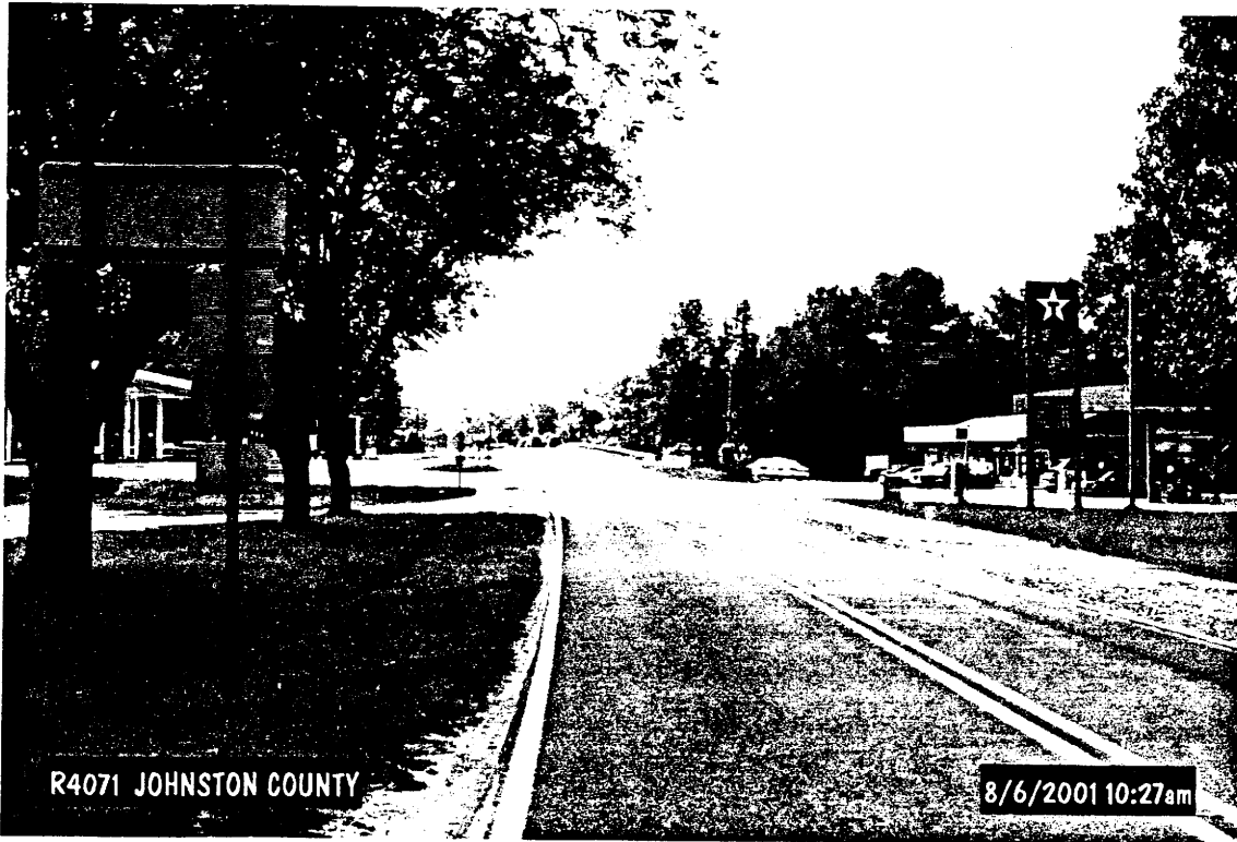
SR 1178 (Keen Road) Looking east towards existing bridge over I-95
