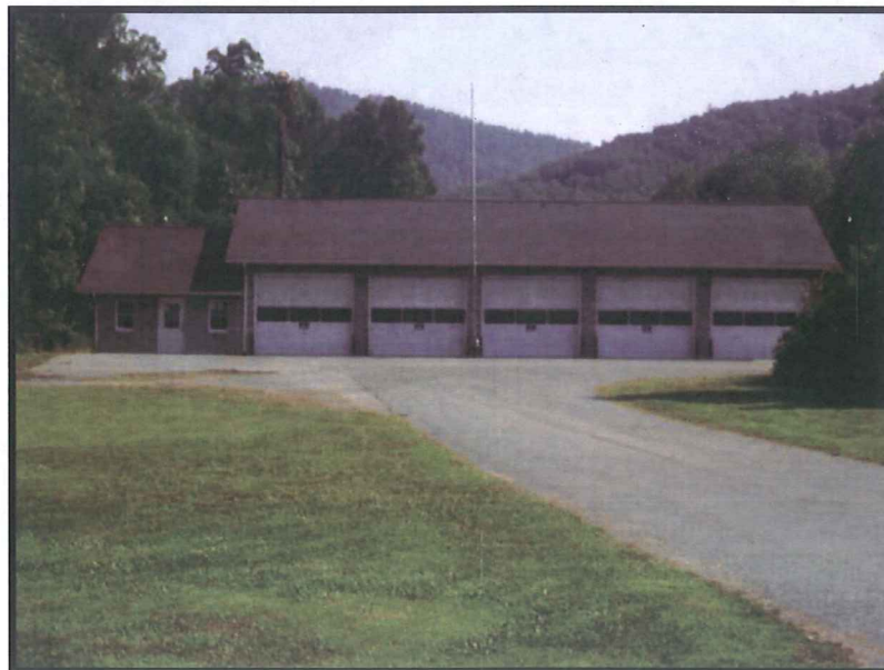
Garren Creek Volunteer Firestation
