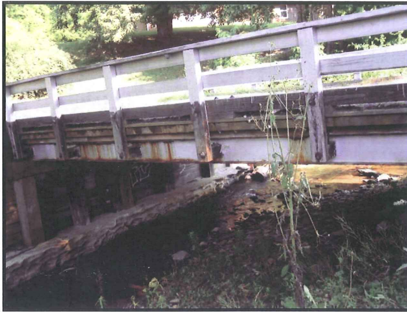
Downstream Side of Bridge No. 108
