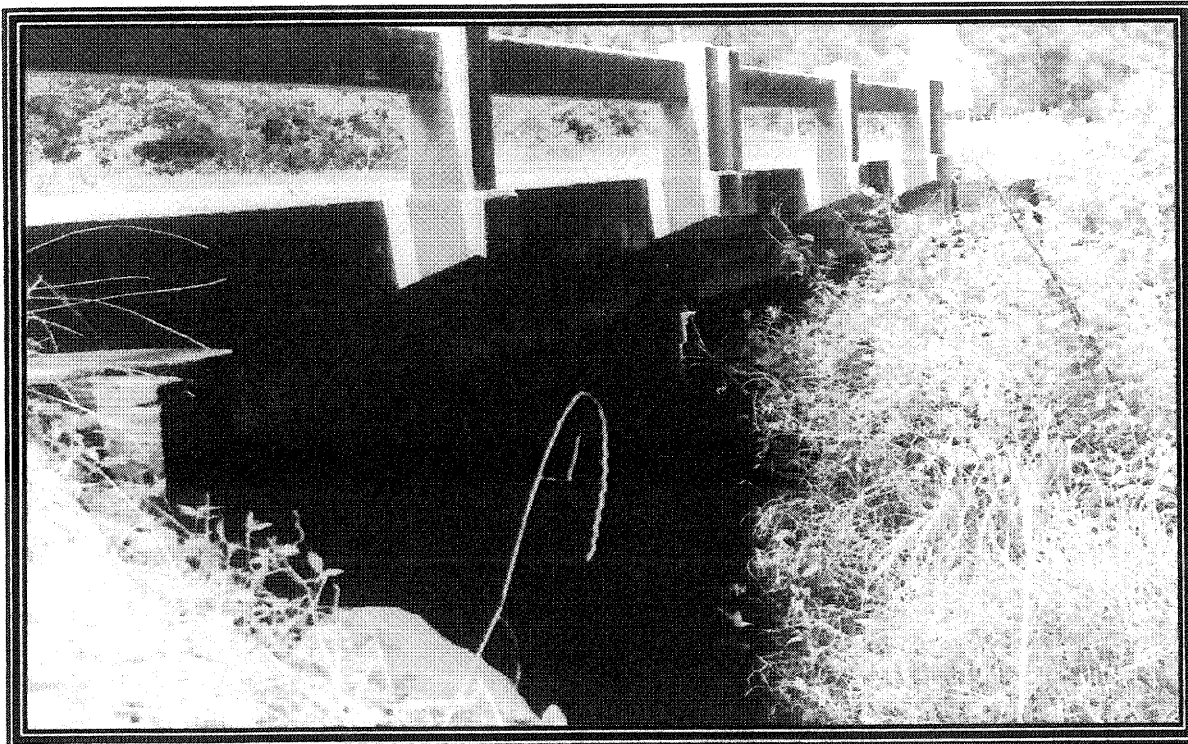
Looking at the North Side of Bridge No. 14
