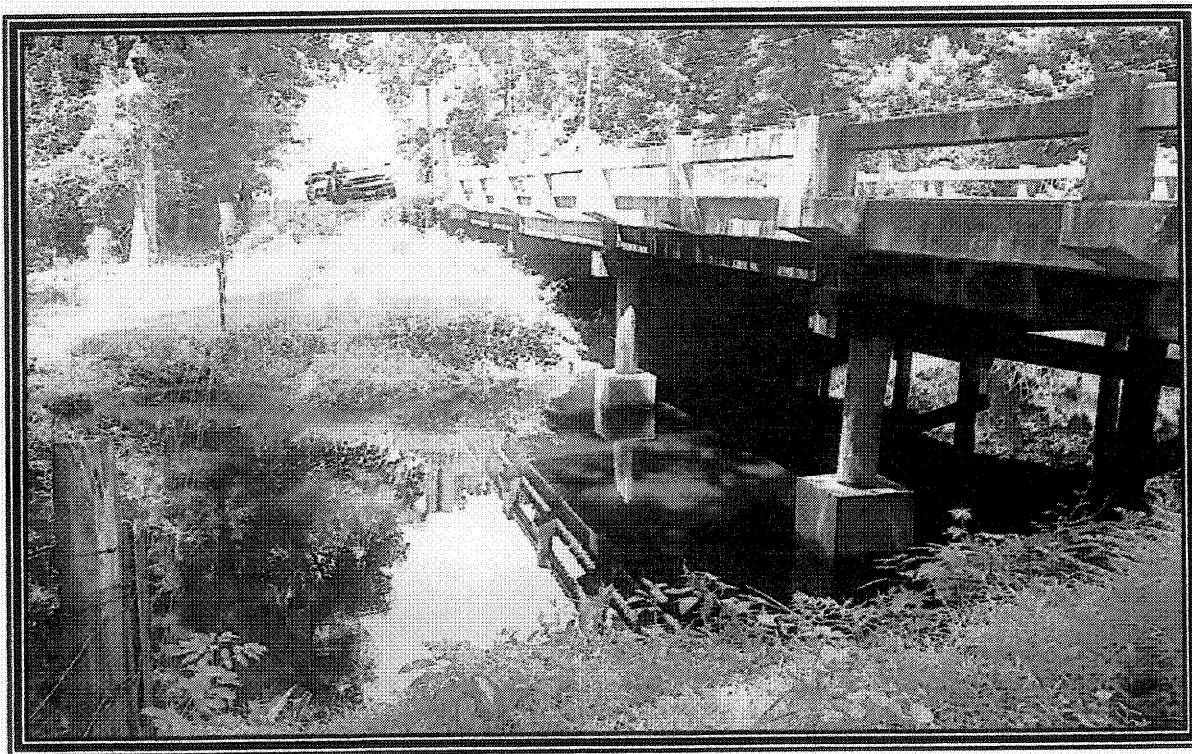
Looking at the South Side of Bridge No. 89
