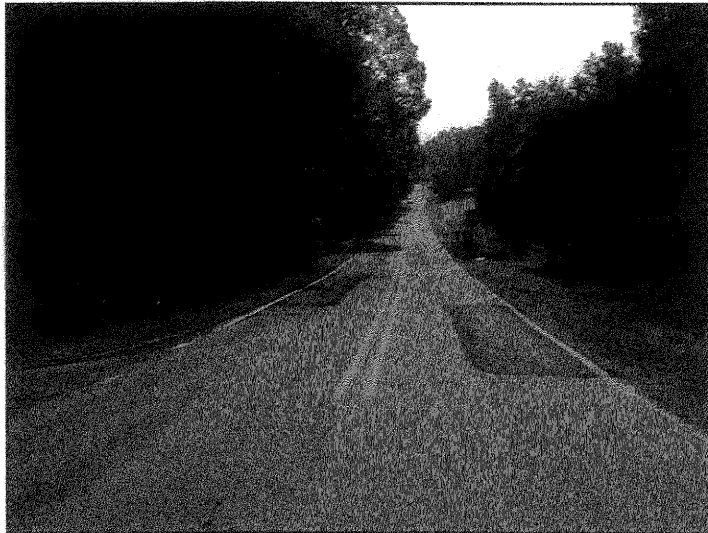
View of east approach from Bridge No. 120.
