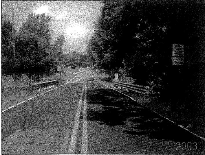
View of west approach from Bridge No. 120.
