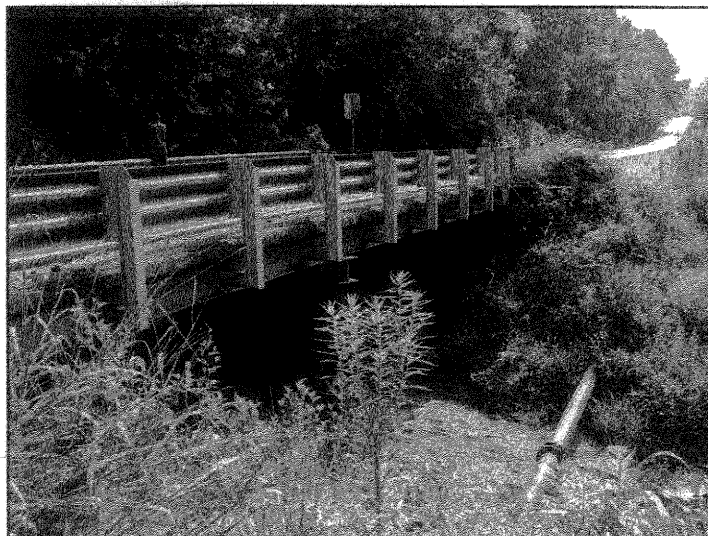
Bridge No. 120 side view from south.
