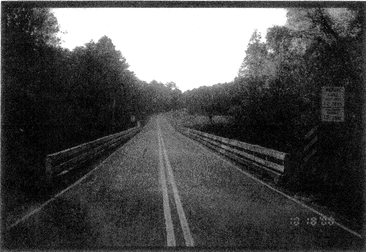
Looking west across Bridge No. 39
