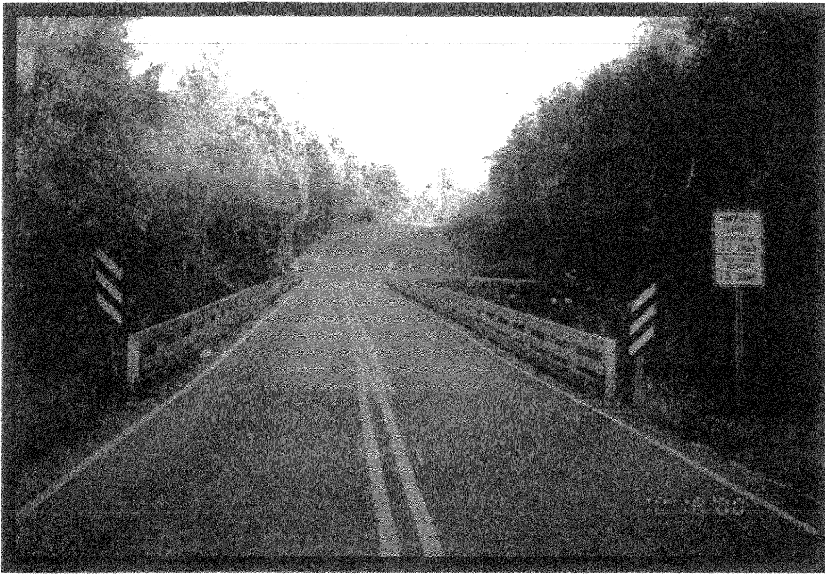
Looking east across Bridge No. 39
