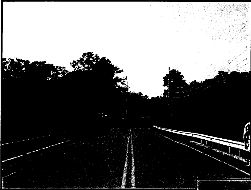
View of south approach.
