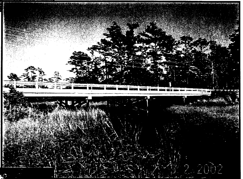
Side view of Bridge No. 72.
