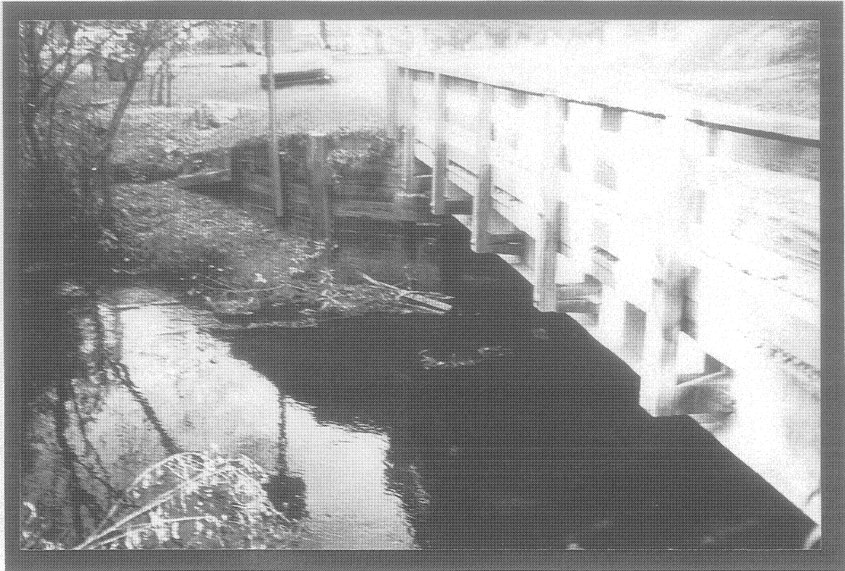
West Face of Bridge
