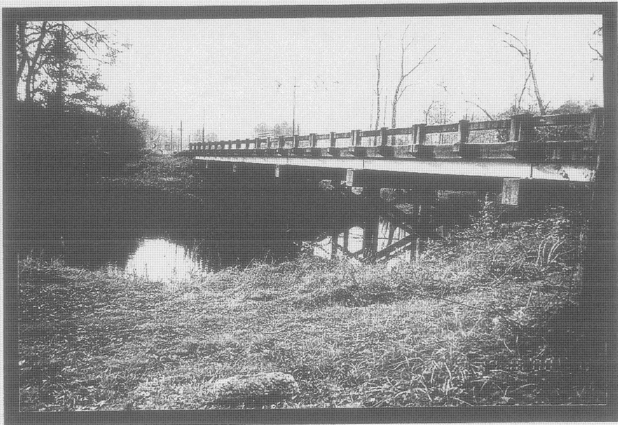
Looking at Downstream side of the Bridge
