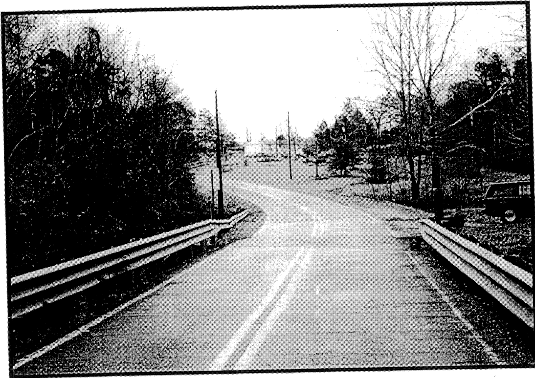
Center of Bridge Facing South
