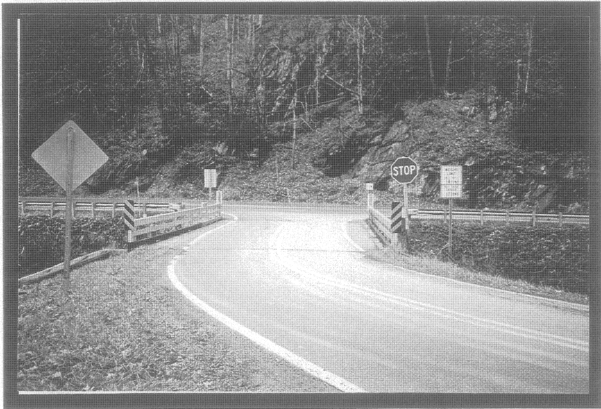
Looking West to the Intersection with NC 88
