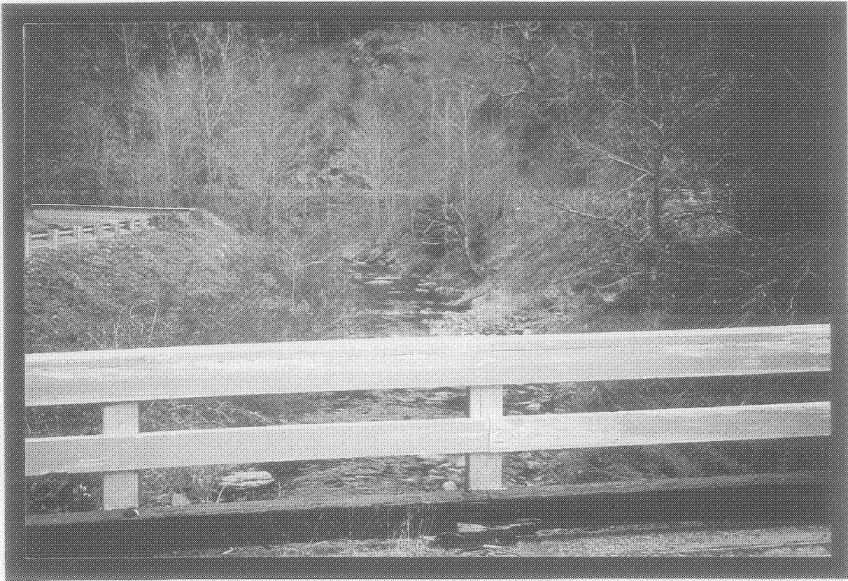
Looking North from the Bridge
