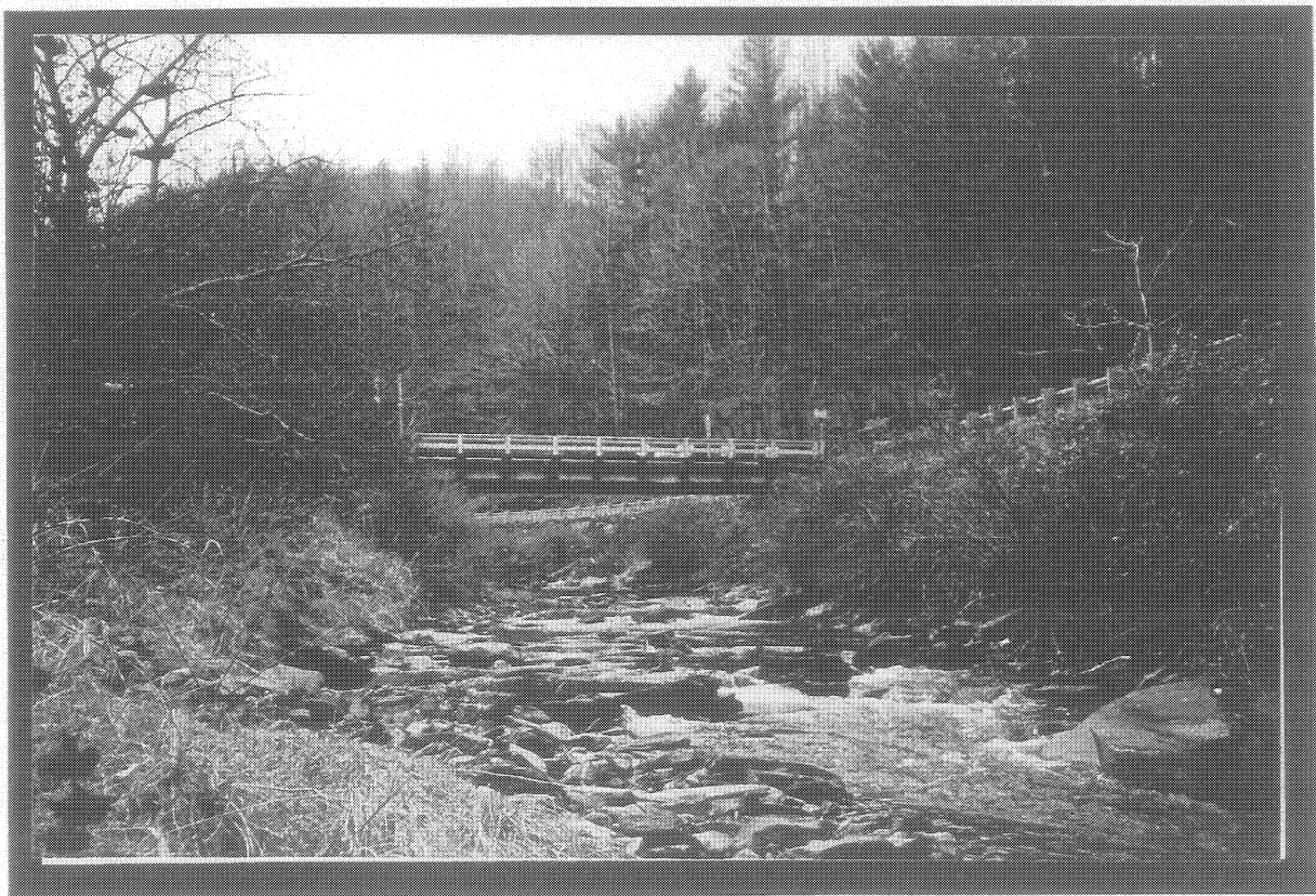
North Face of Bridge
