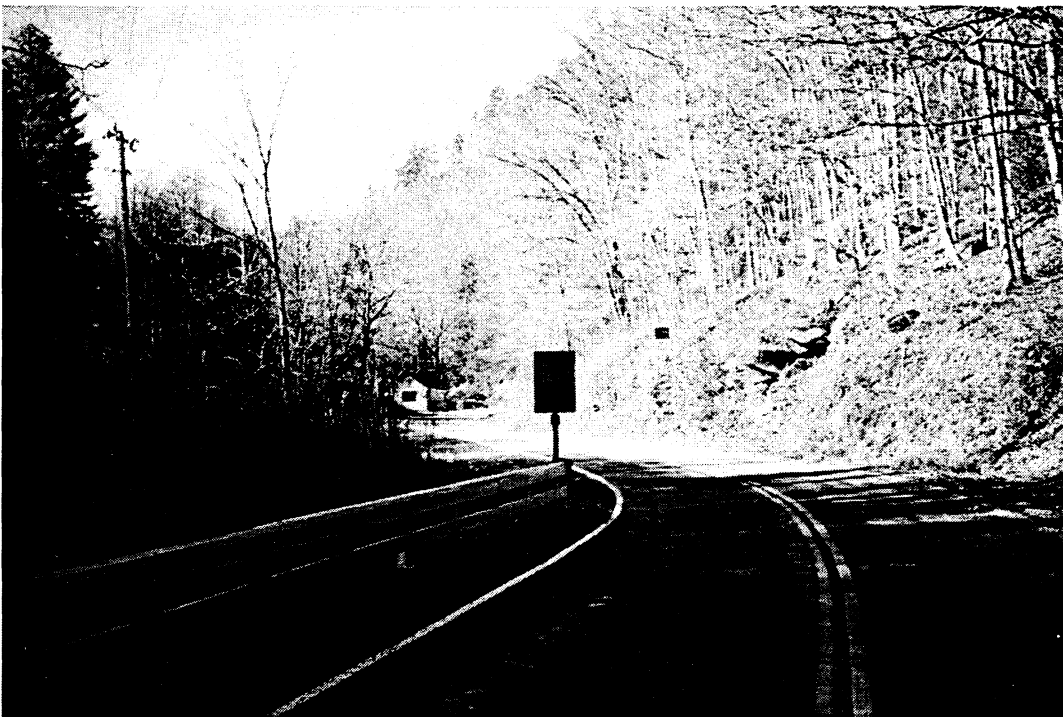
View From Center of Bridge Facing West
