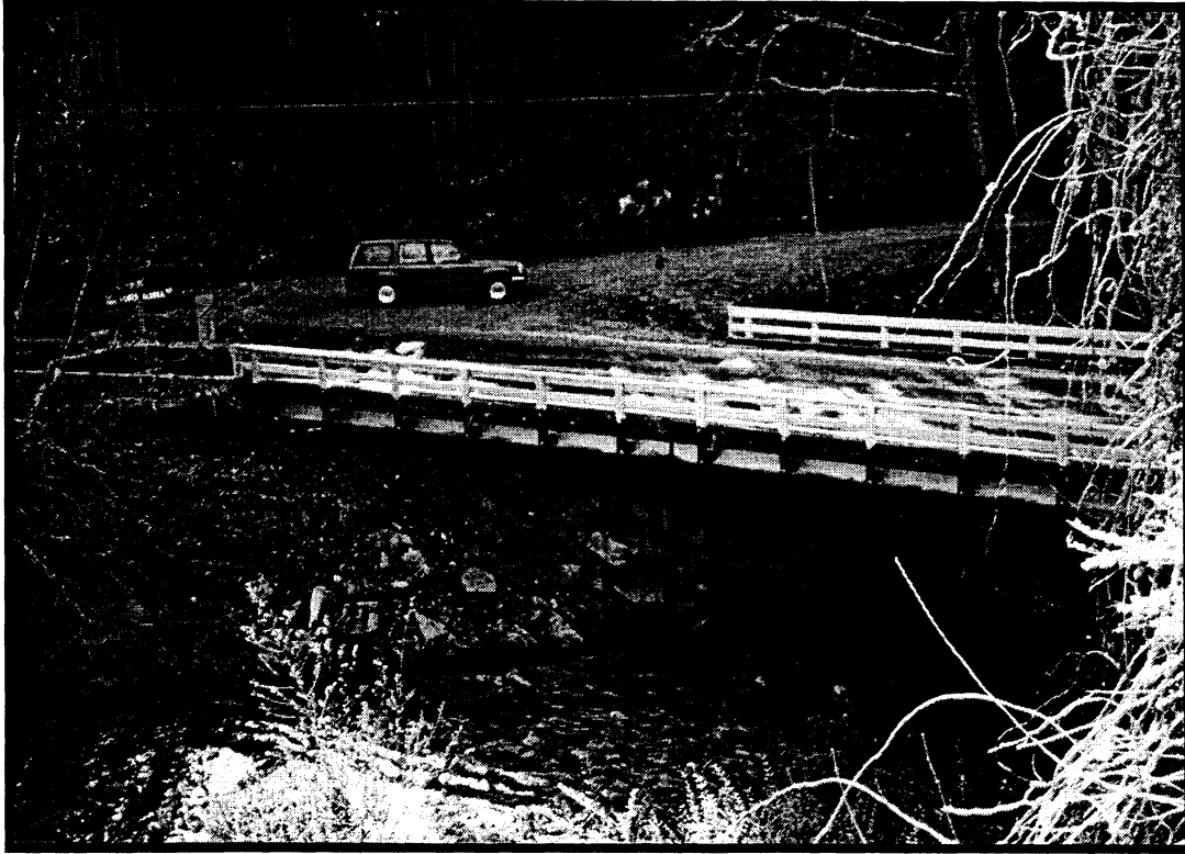
North Face of Bridge No. 106
