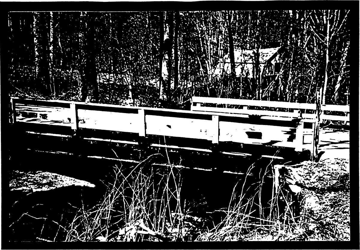
Bridge No. 175 West Face of Bridge
