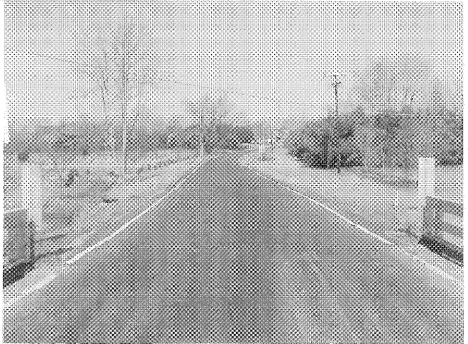
NORTH APPROACH LOOKING NORTH
