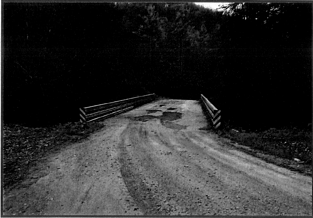
Looking South Across Bridge No. 53.
