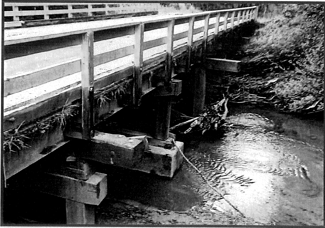
Upstream Side of Bridge No. 53.
