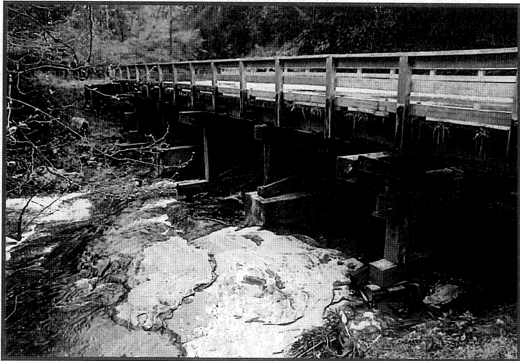
Downstream Side of Bridge No. 53.
