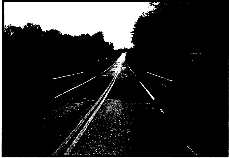
Looking south along SR 1791 across Bridge No. 265.
