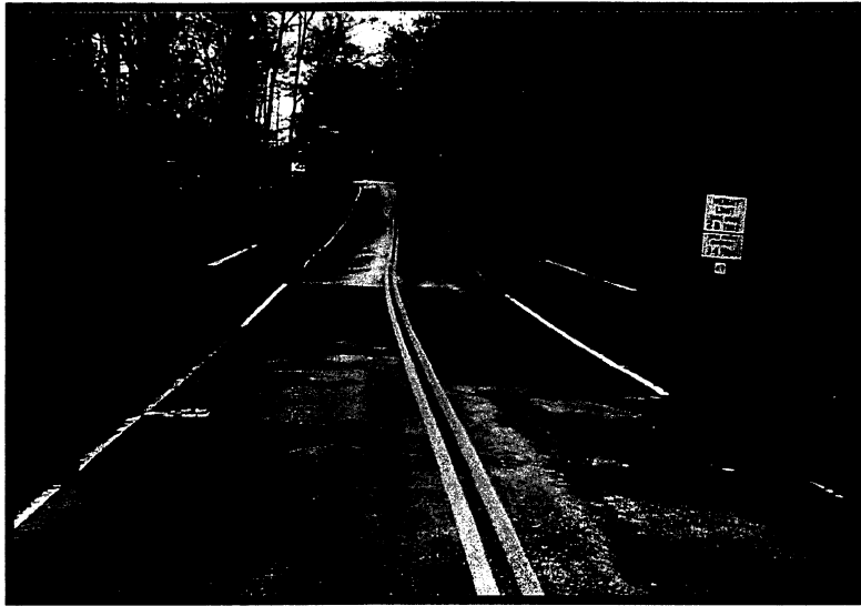
Looking north along SR 1791 across Bridge No. 265.
