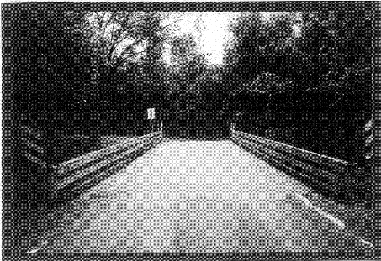
Roadway "Dip" - Looking East
