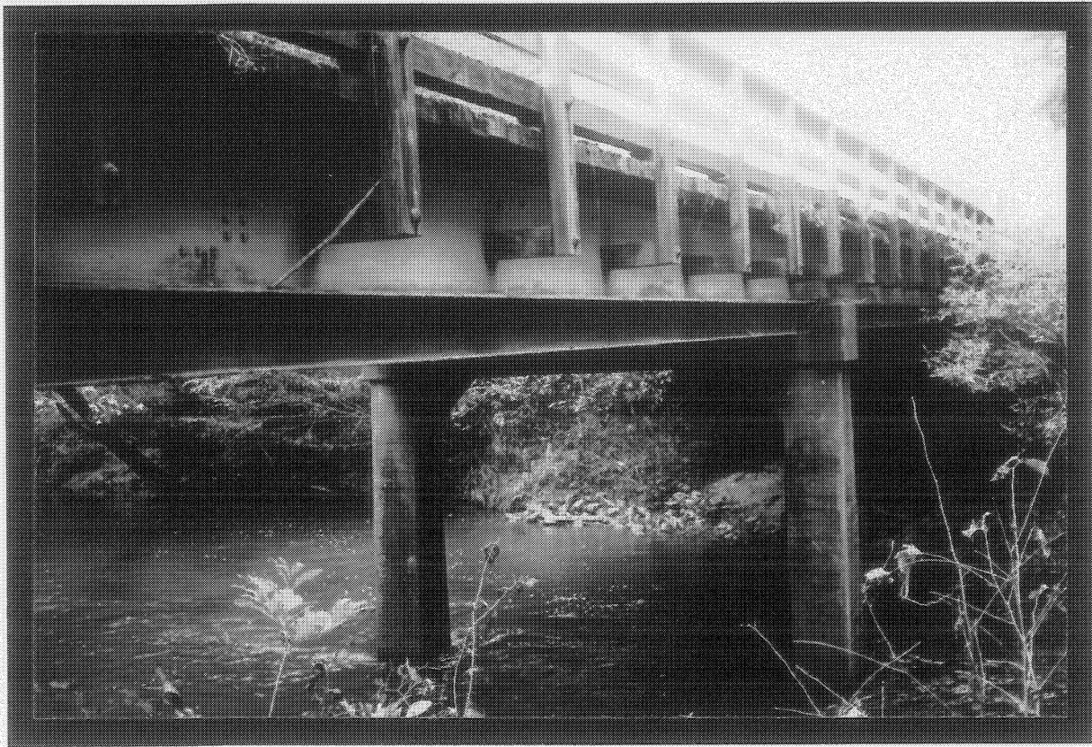
North Face of Bridge
