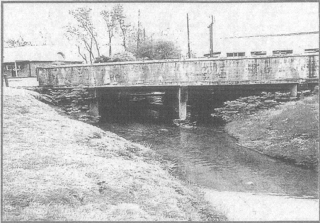
Side view of Bridge No. 356.
