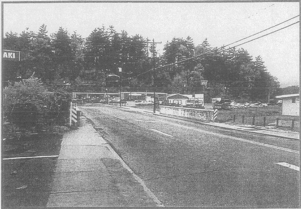
Looking west along SR 1127 across Bridge No. 356.
