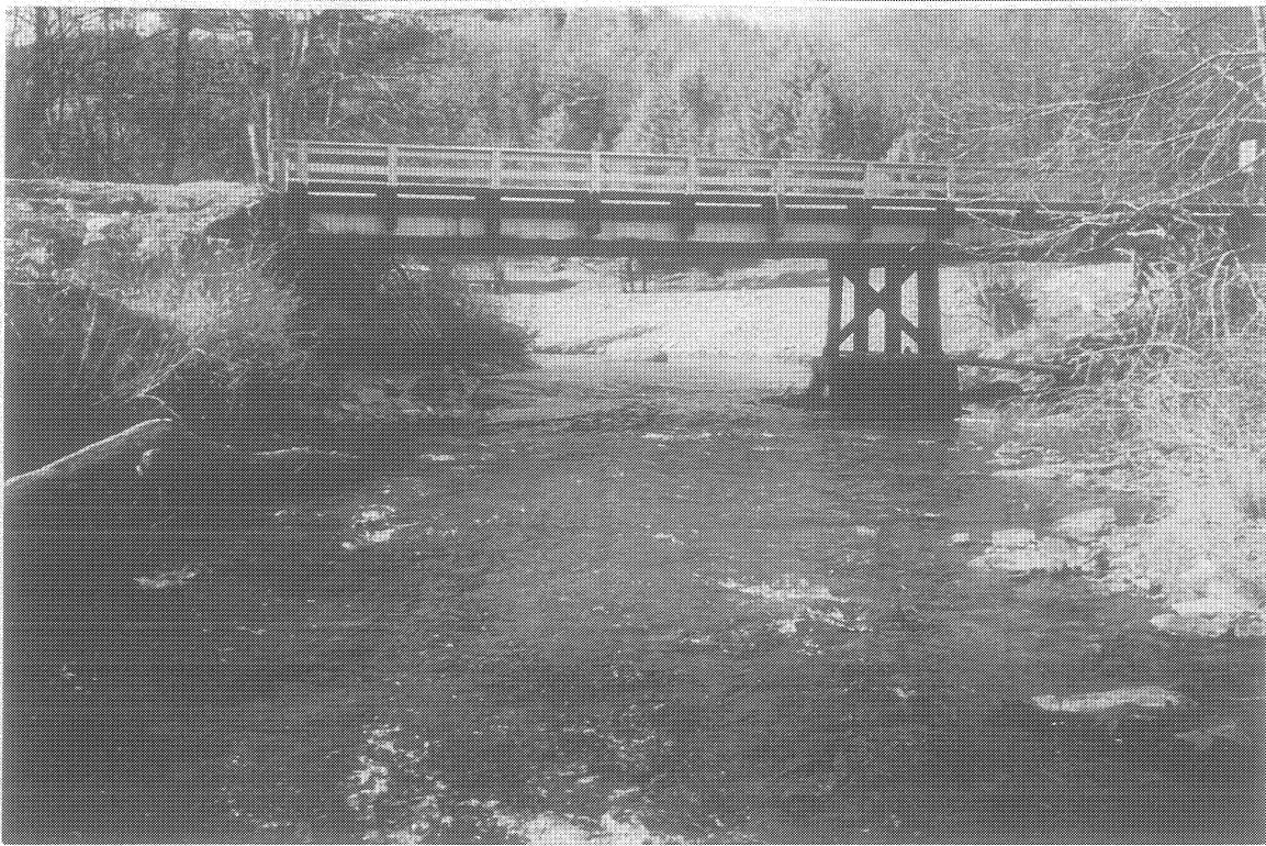
PHOTO #3: Southeast face of Bridge No. 53
