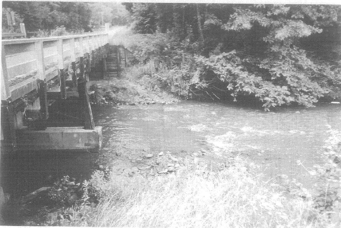
PHOTO #4: Northwest face of Bridge No. 53
