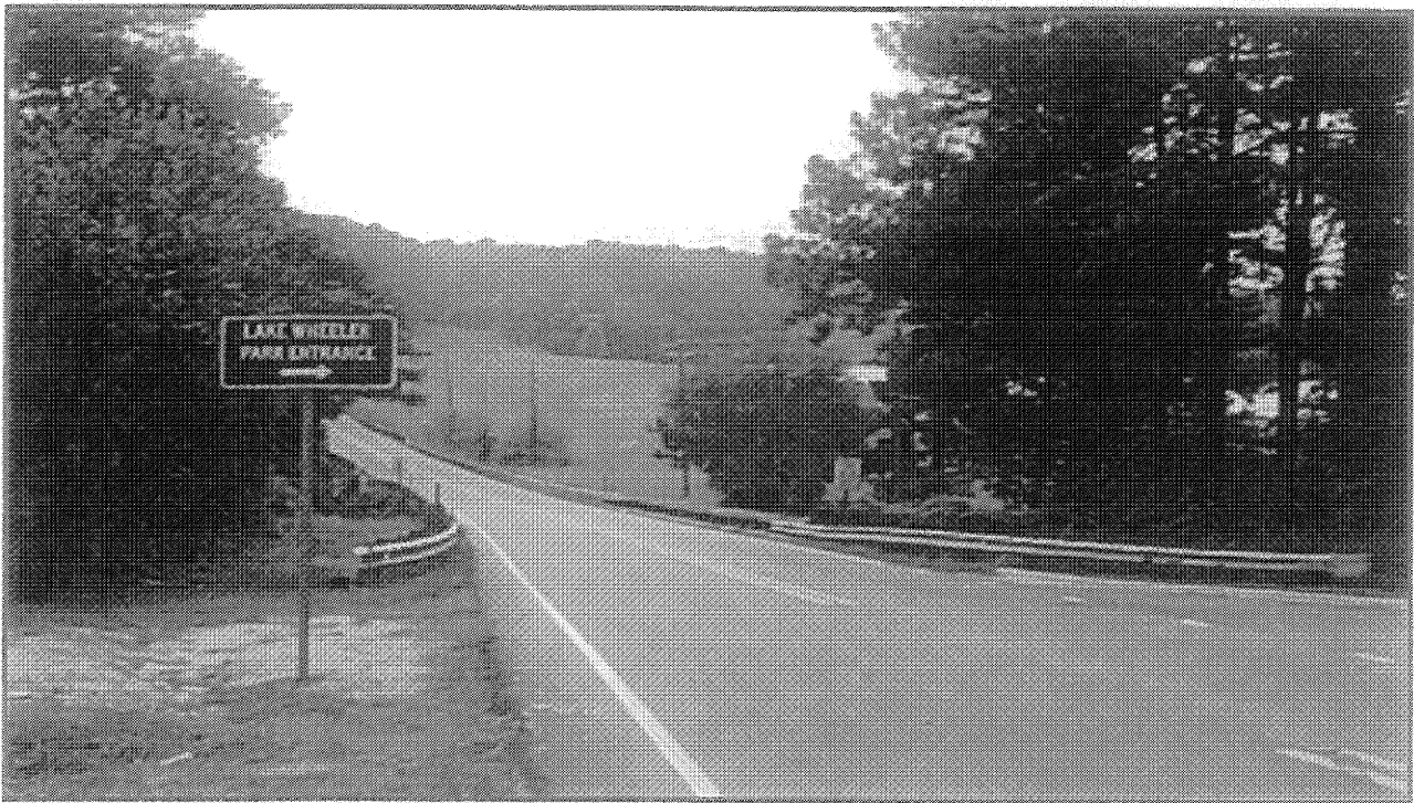
Looking south along SR 1375 across Bridge No. 471. Park entrance to the right.
