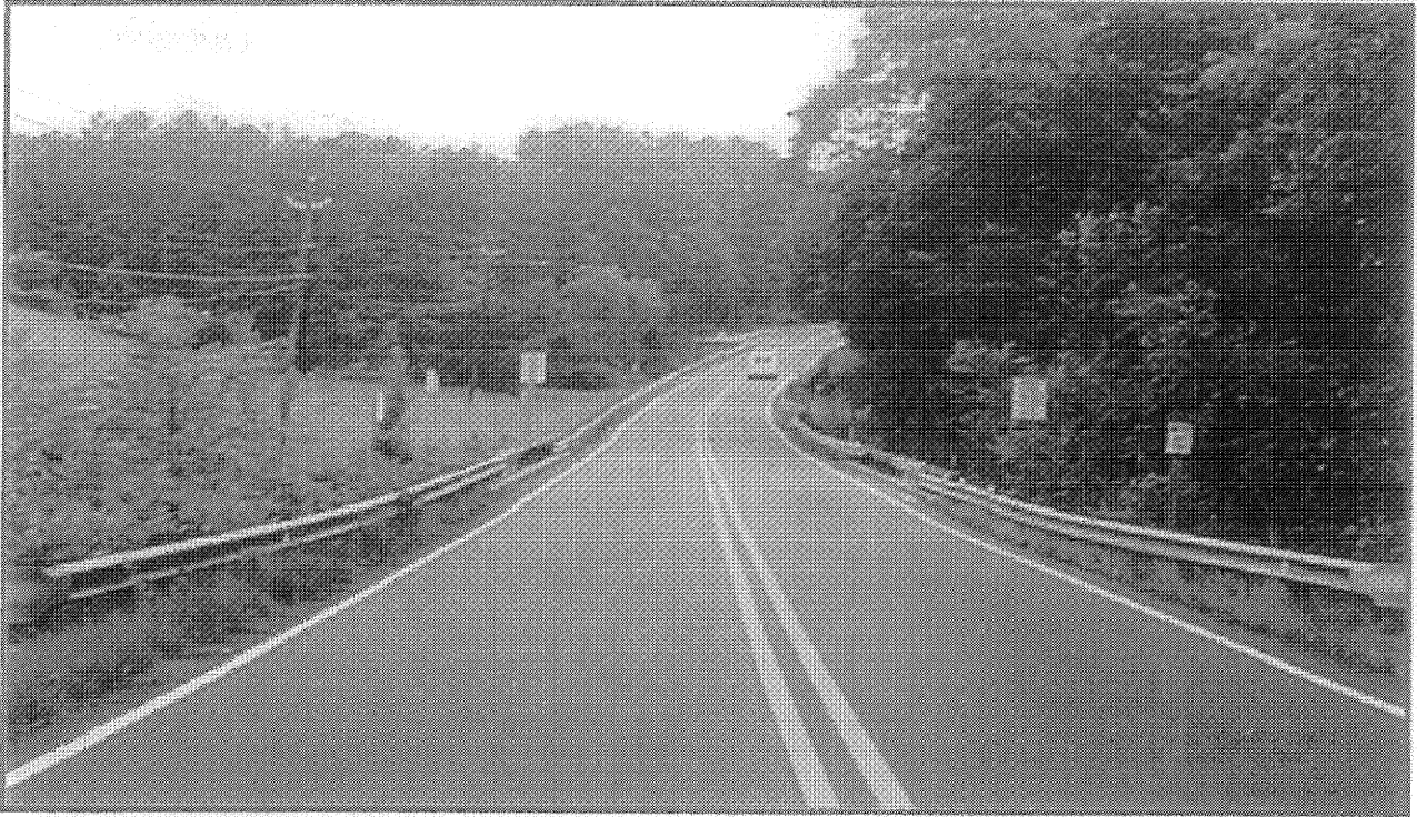
Looking north along SR 1375 across Bridge No. 301.
