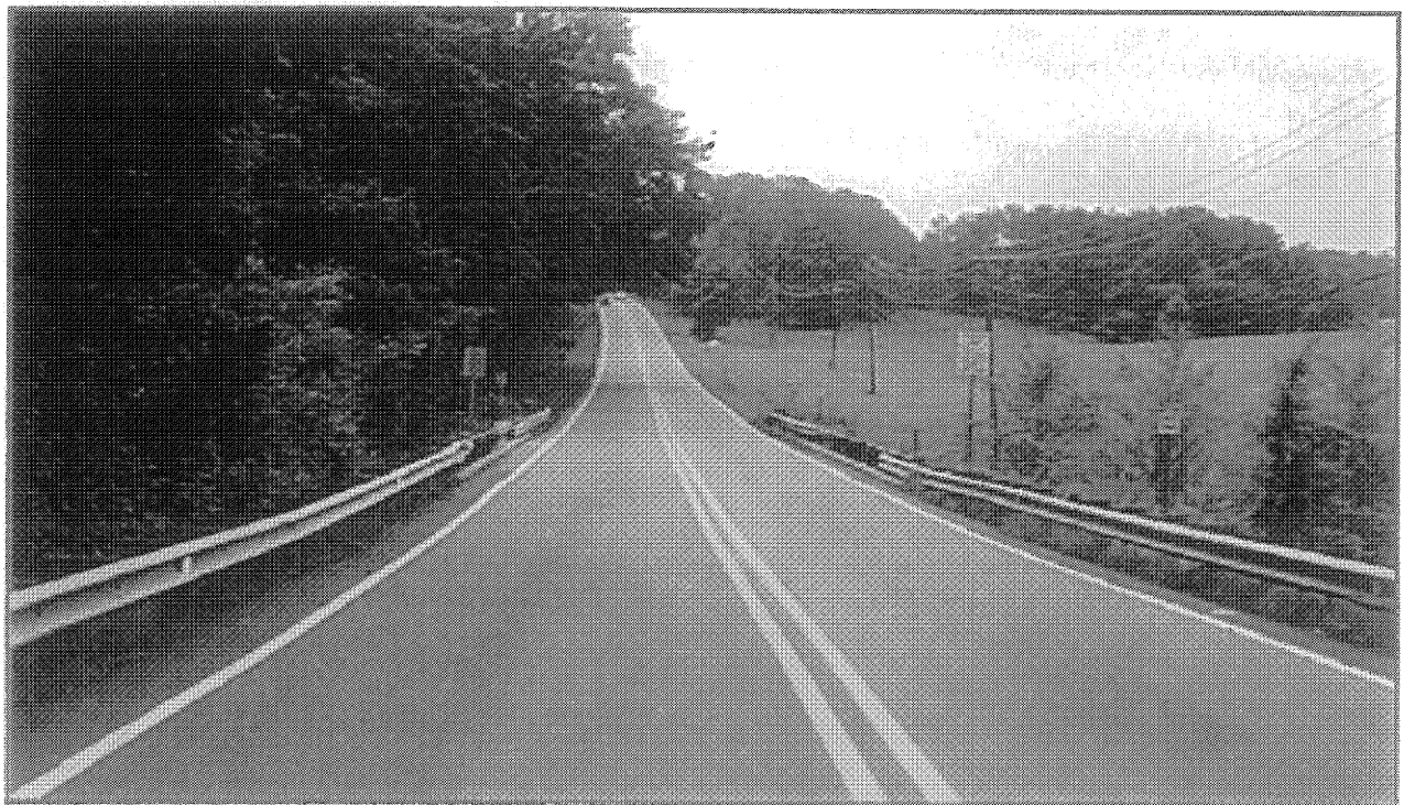
Looking south along SR 1375 across Bridge No. 301.
