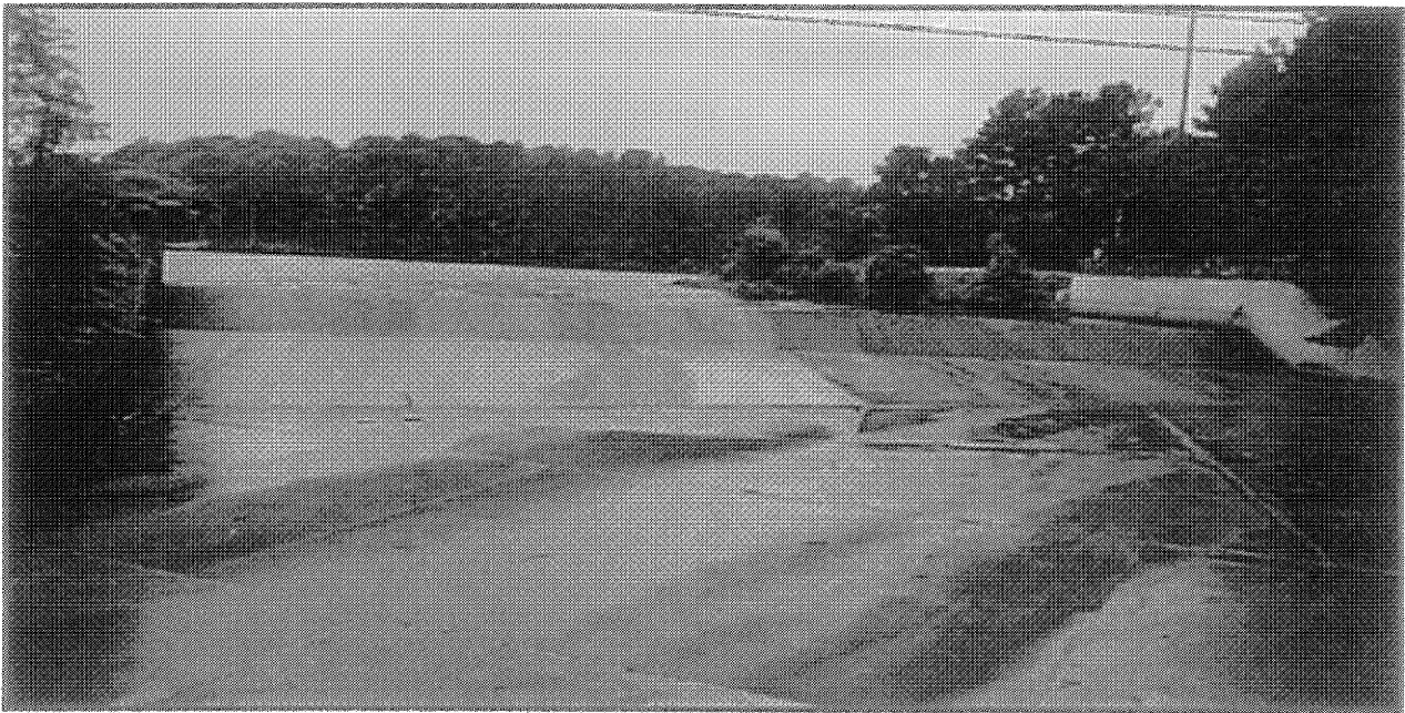
Spillway viewed from Bridge No. 471.
