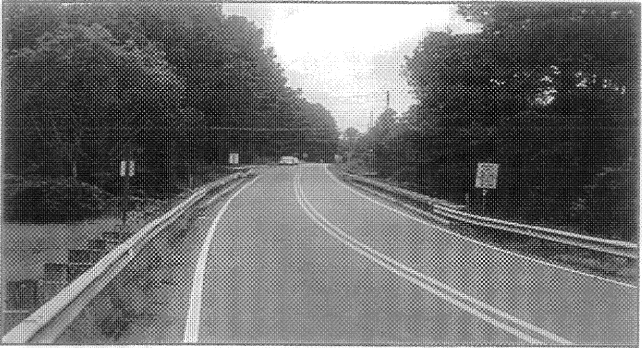
Looking north along SR 1375 across Bridge No. 471.
