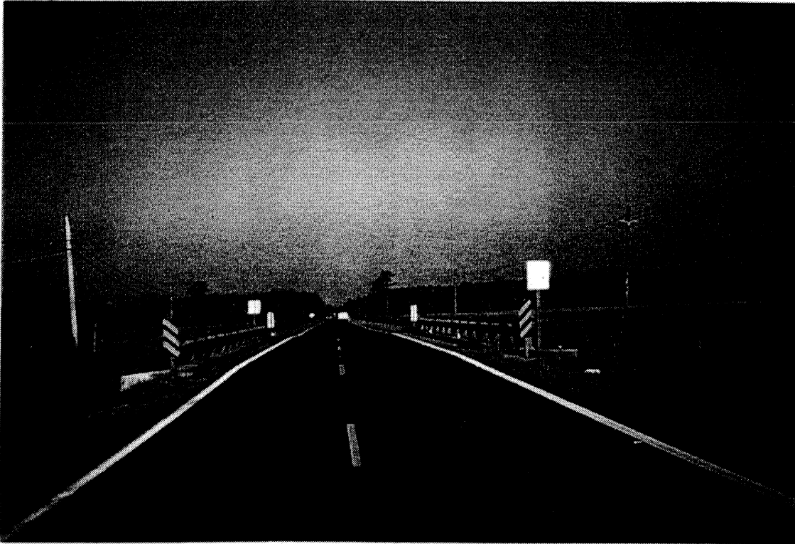
LOOKING WEST AT EAST APPROACH
