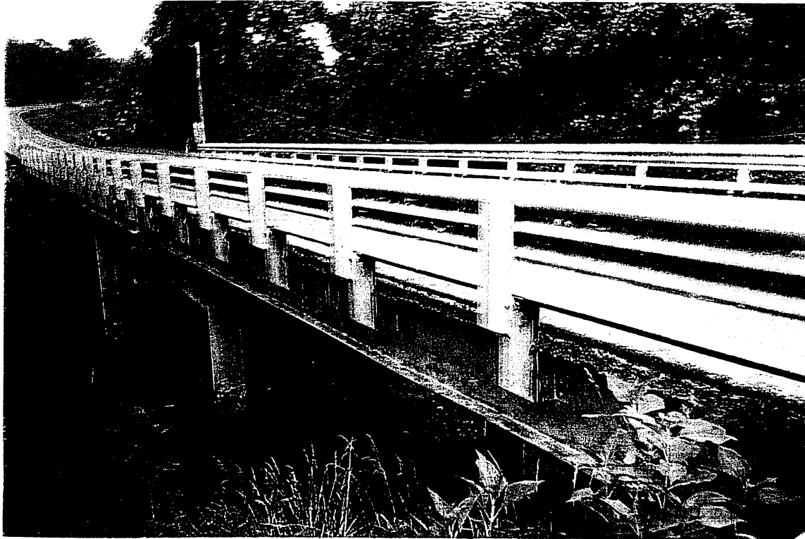
PHOTO #4: North Face of Bridge No. 27
