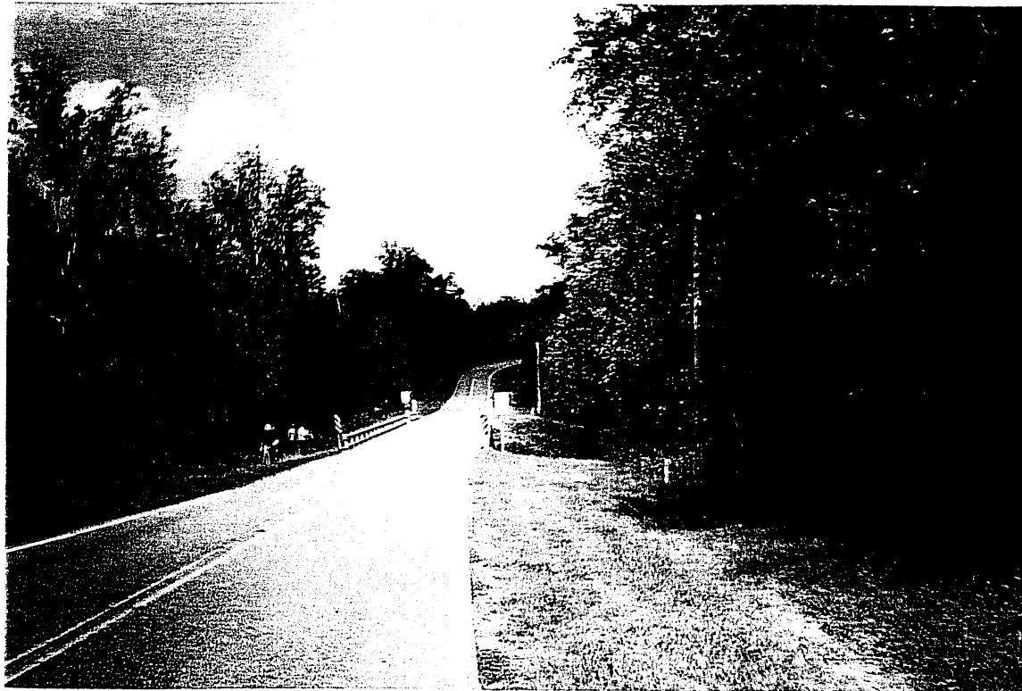
PHOTO #1: Looking to the northeast, along SR 1001
