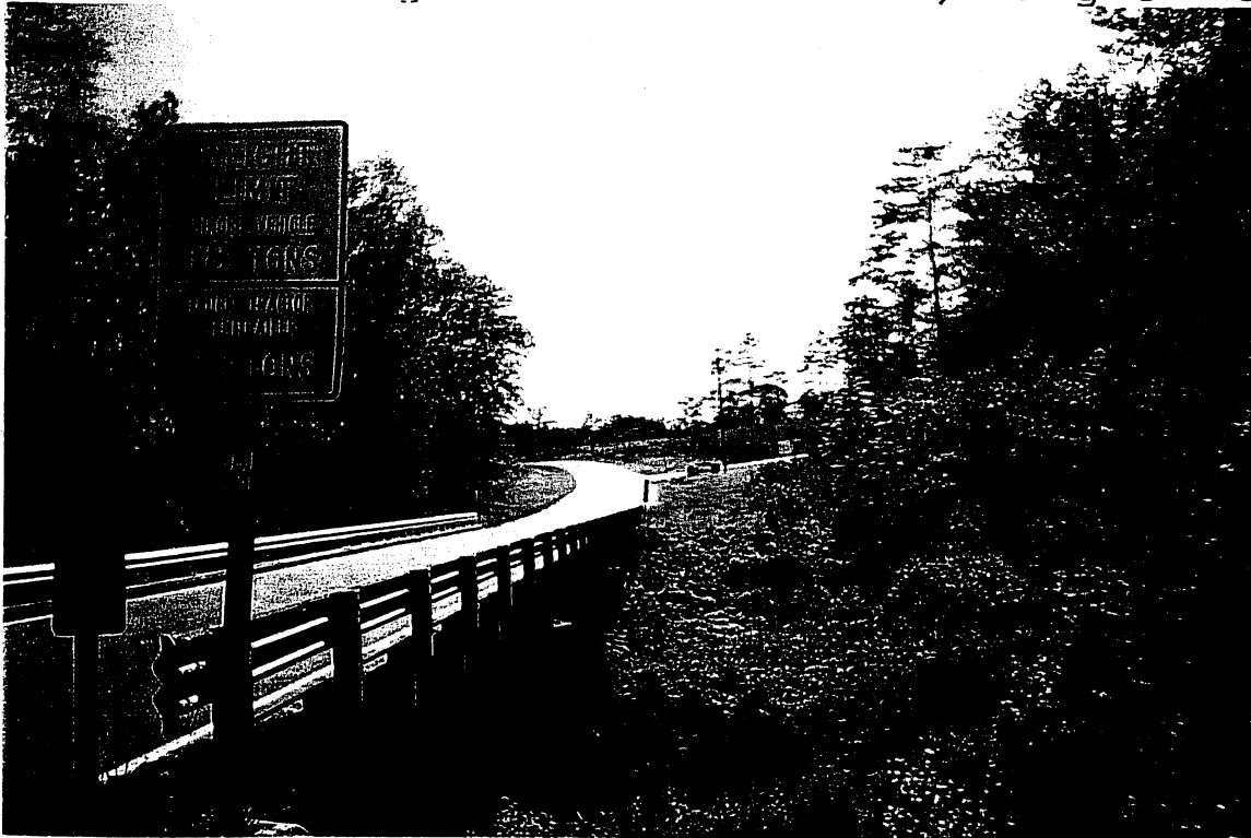
PHOTO #2: Looking to the southwest, along SR 1001
