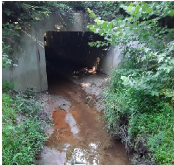
Image 6. Site 2 - 10' X 9' RCBC outlet looking upstream
