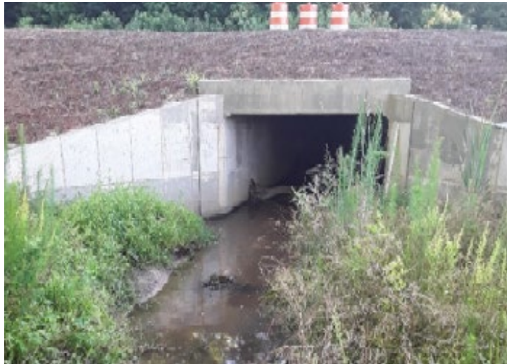
Image 5. Site 2 - 10' X 9' RCBC inlet looking downstream
