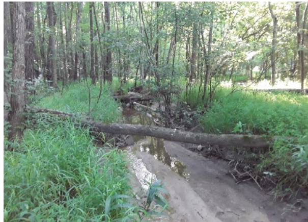
Image 11. Site 3 - At culvert centerline looking downstream across floodplain
