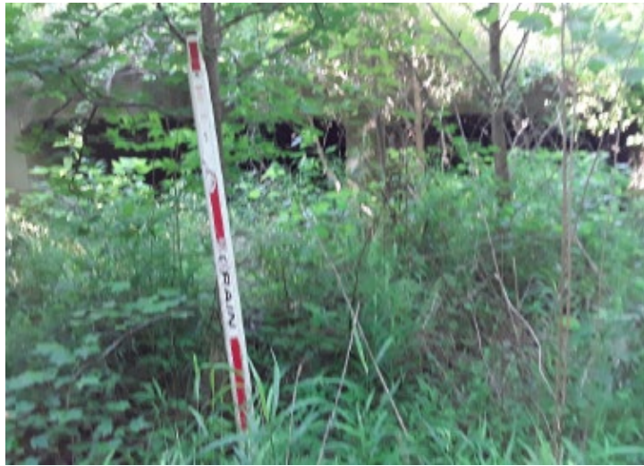
Image 2. Site 1 – Outlet looking upstream
