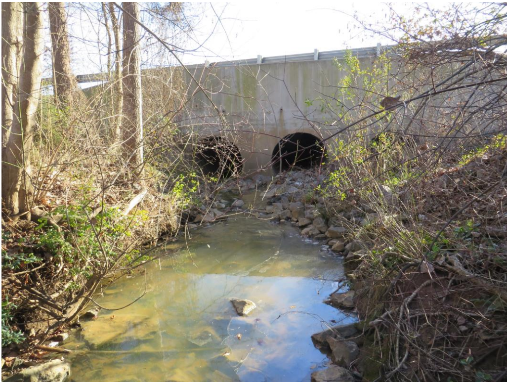
Looking Downstream from RCPs' Outlets
