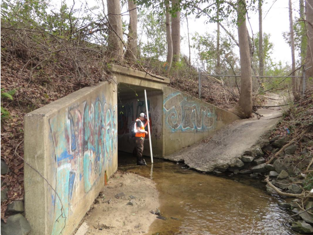
Looking at Upstream Face of 1 @ 8' x 9' RCBC
