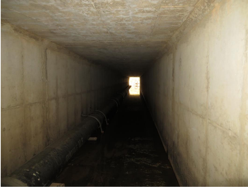
Looking Downstream Inside RCBC
