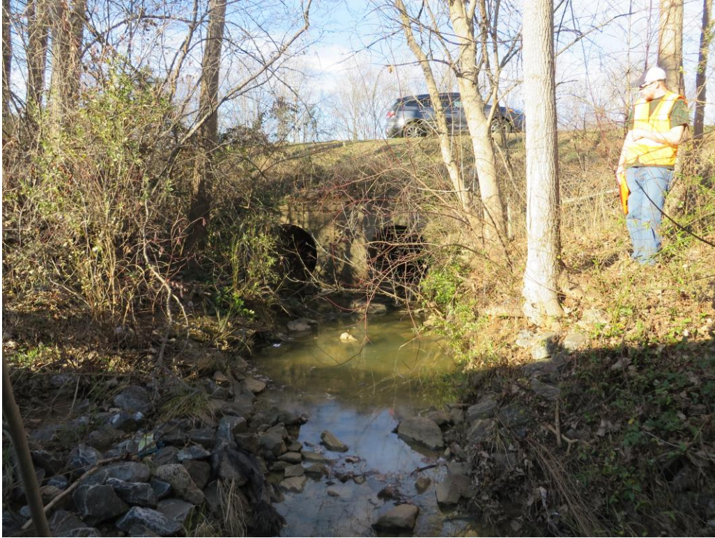
Looking at Downstream Face of 2 @ 54" RCP
