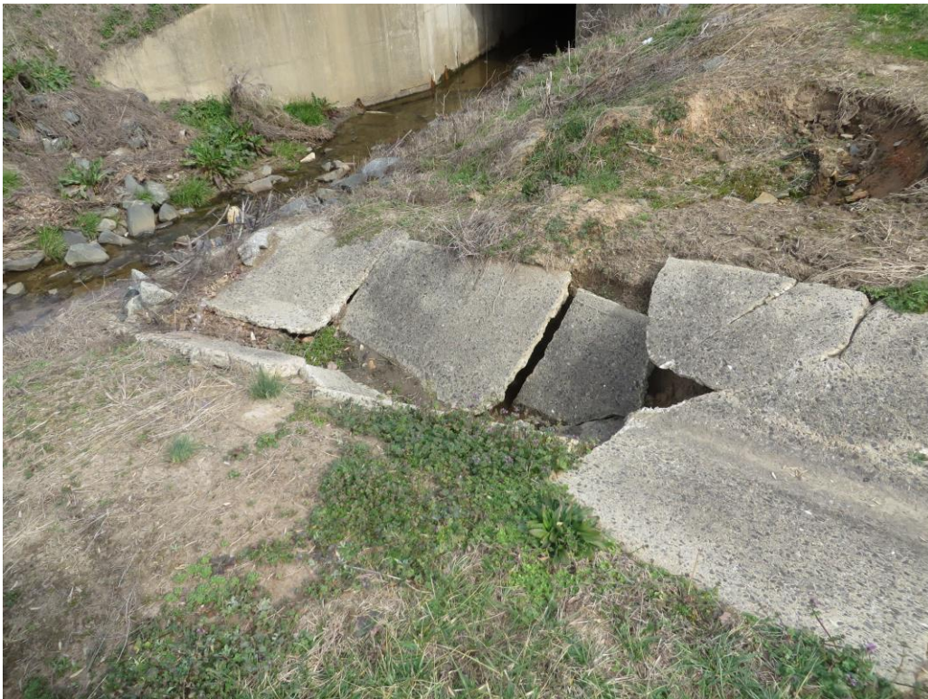
Paved Ditch at Upstream Right
