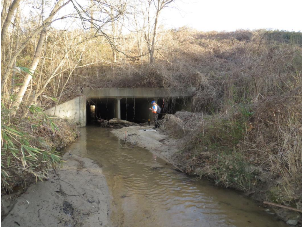
Looking at Upstream Face of 1 @ 7' x 9', 2 @ 8' x 9' RCBC
