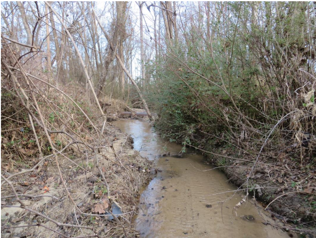
Looking Downstream from RCBC Outlet
