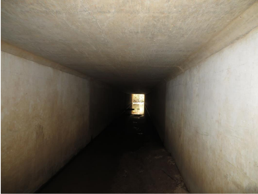
Looking Inside RCBC
