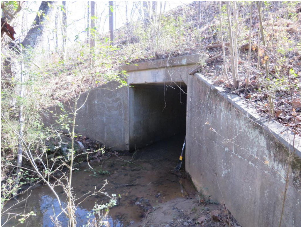
Looking at Upstream Face of 1 @ 8' x 8' RCBC
