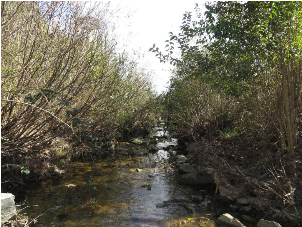
Looking Downstream from RCBC Outlet
