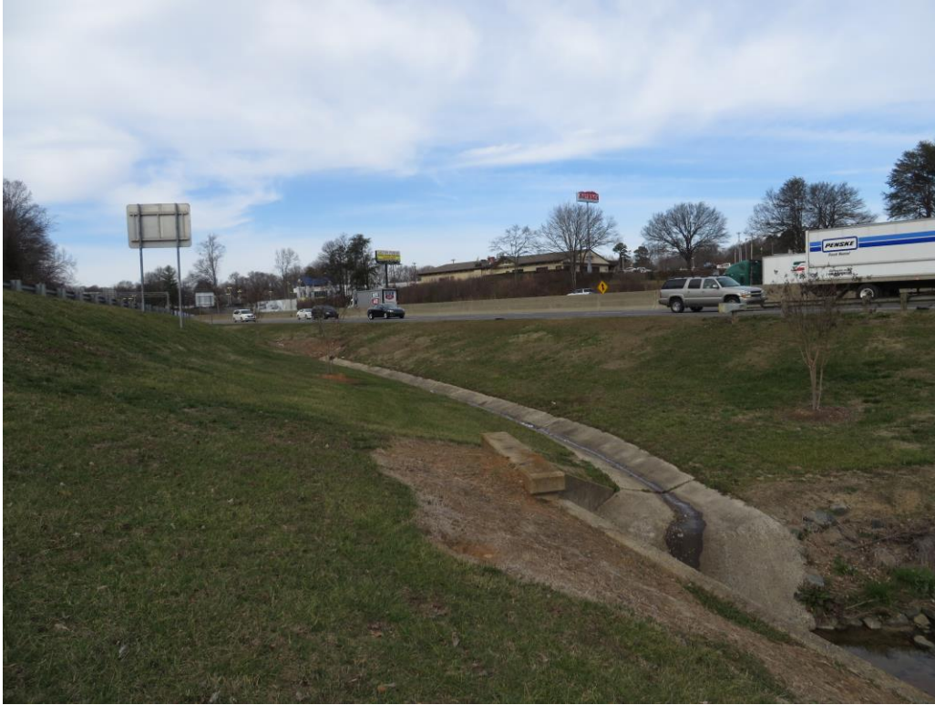
Paved Ditch at Downstream Left
