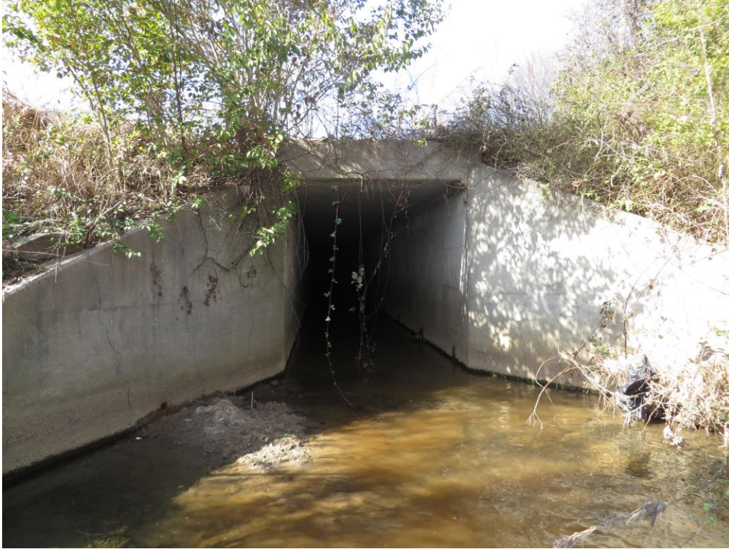
Downstream Face of 1 @ 8' x 9' RCBC
