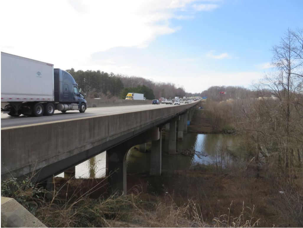
Looking at Downstream Face
