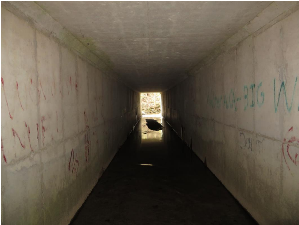
Looking Upstream Inside Culvert from Downstream End
