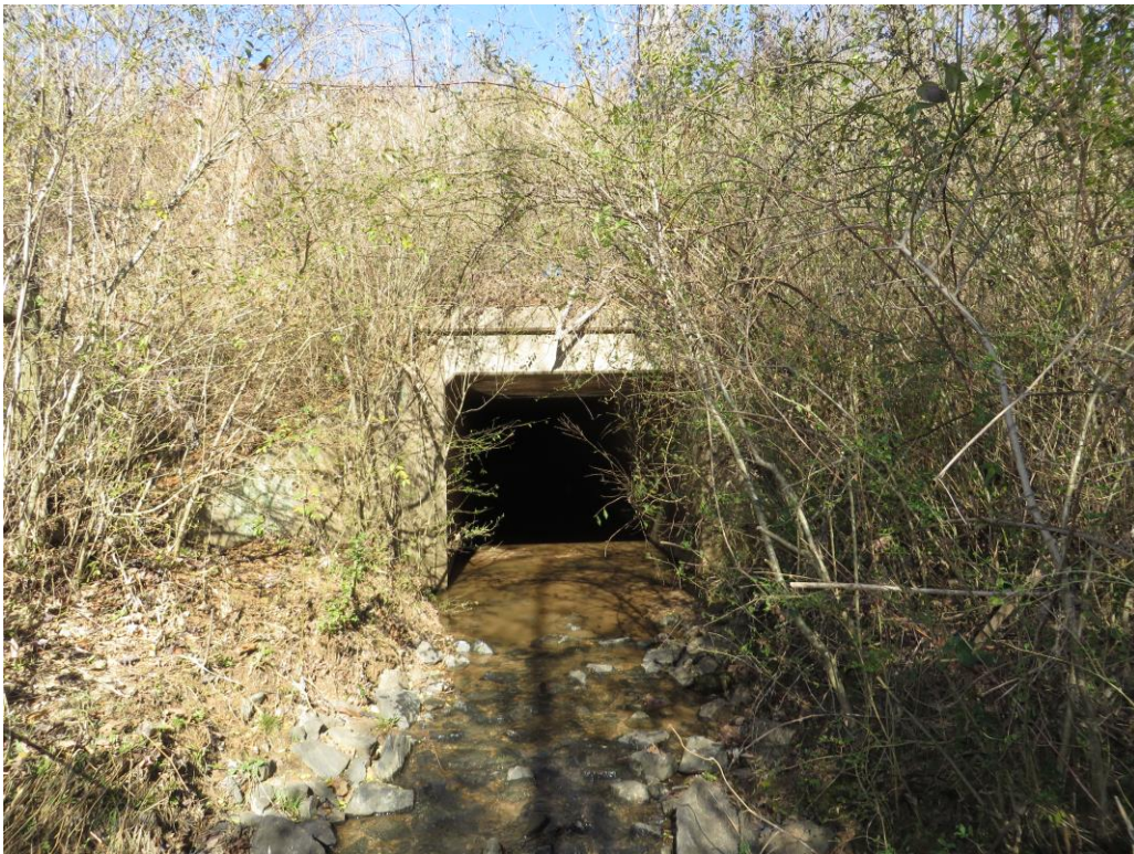
Looking at Downstream Face of 1 @ 8' x 8' RCBC
