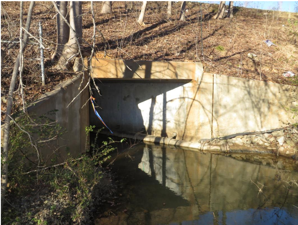
Looking at Downstream Face of 1 @ 8' x 8' RCBC
