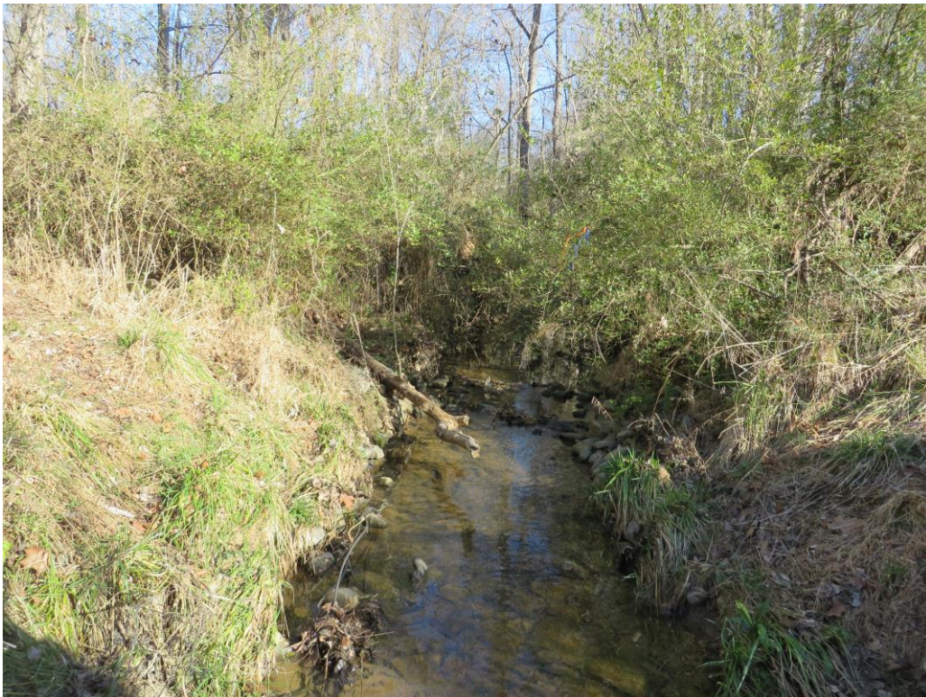
Looking Upstream from RCBC Inlet
