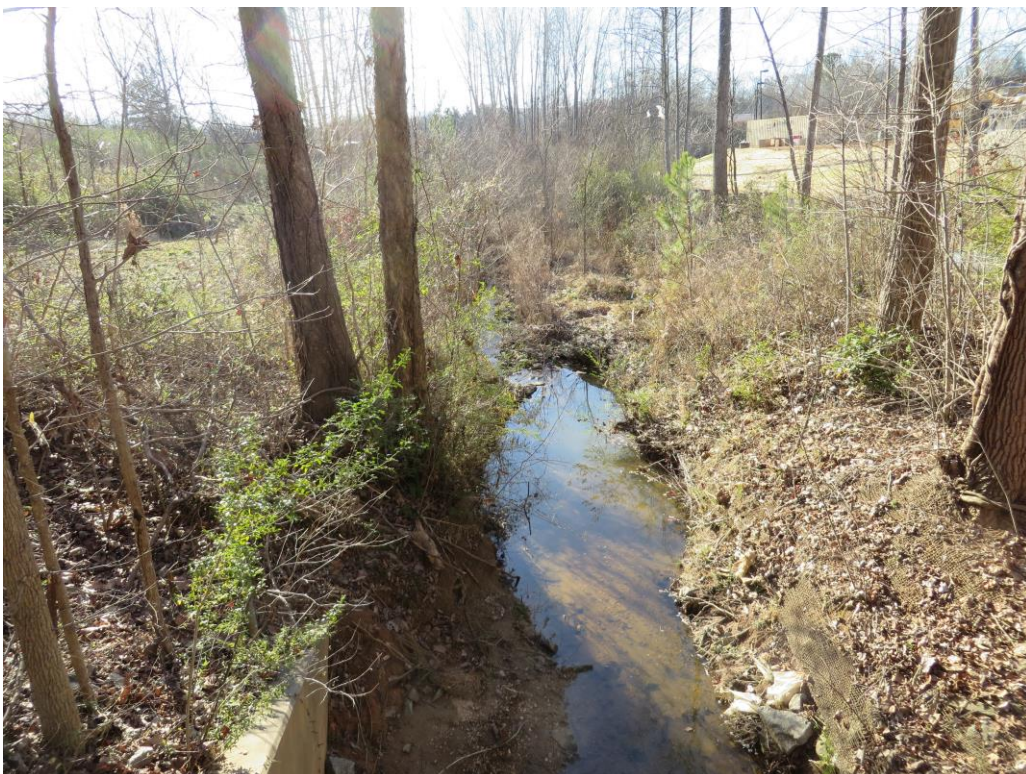
Looking Downstream from Outlet
