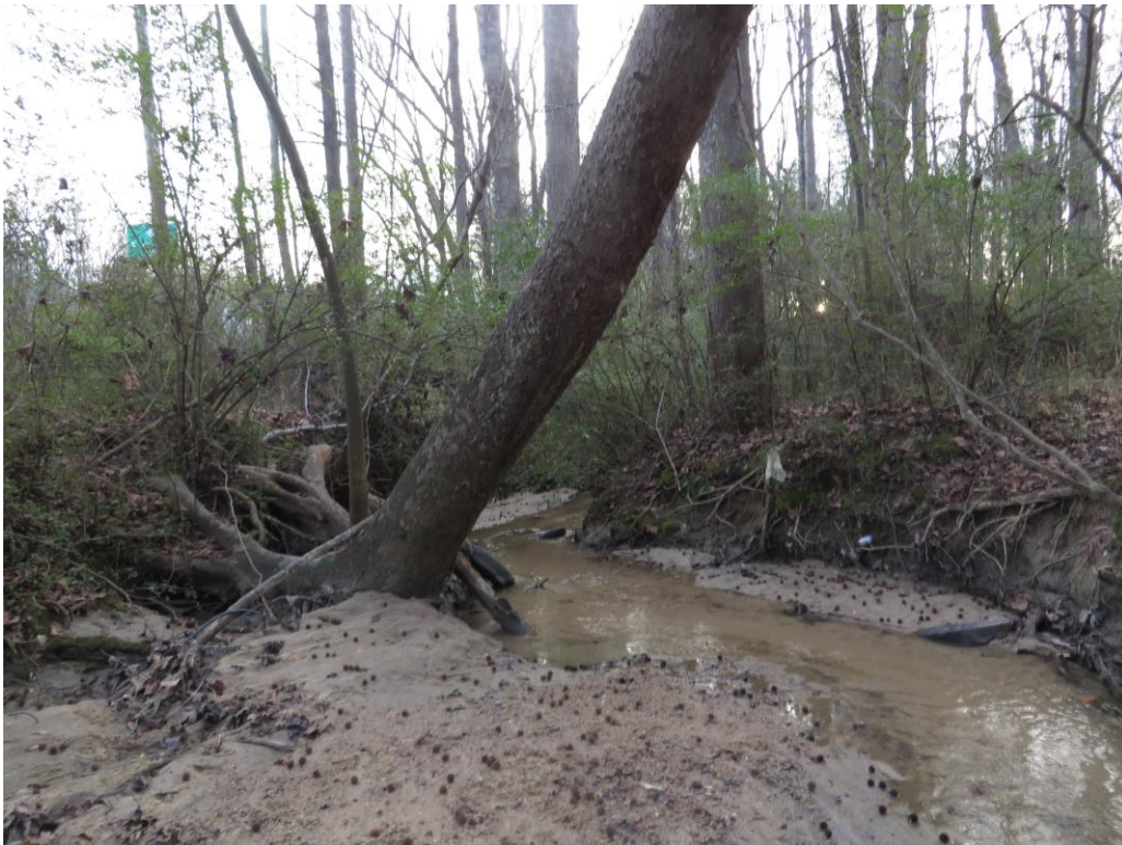
Looking Upstream from RCBC Inlet
