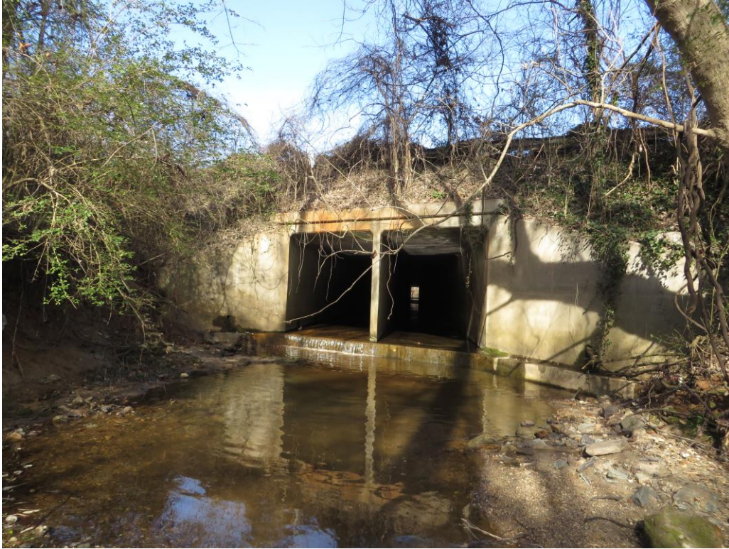
Looking at Downstream Face of 2 @ 8' x 9' RCBC
