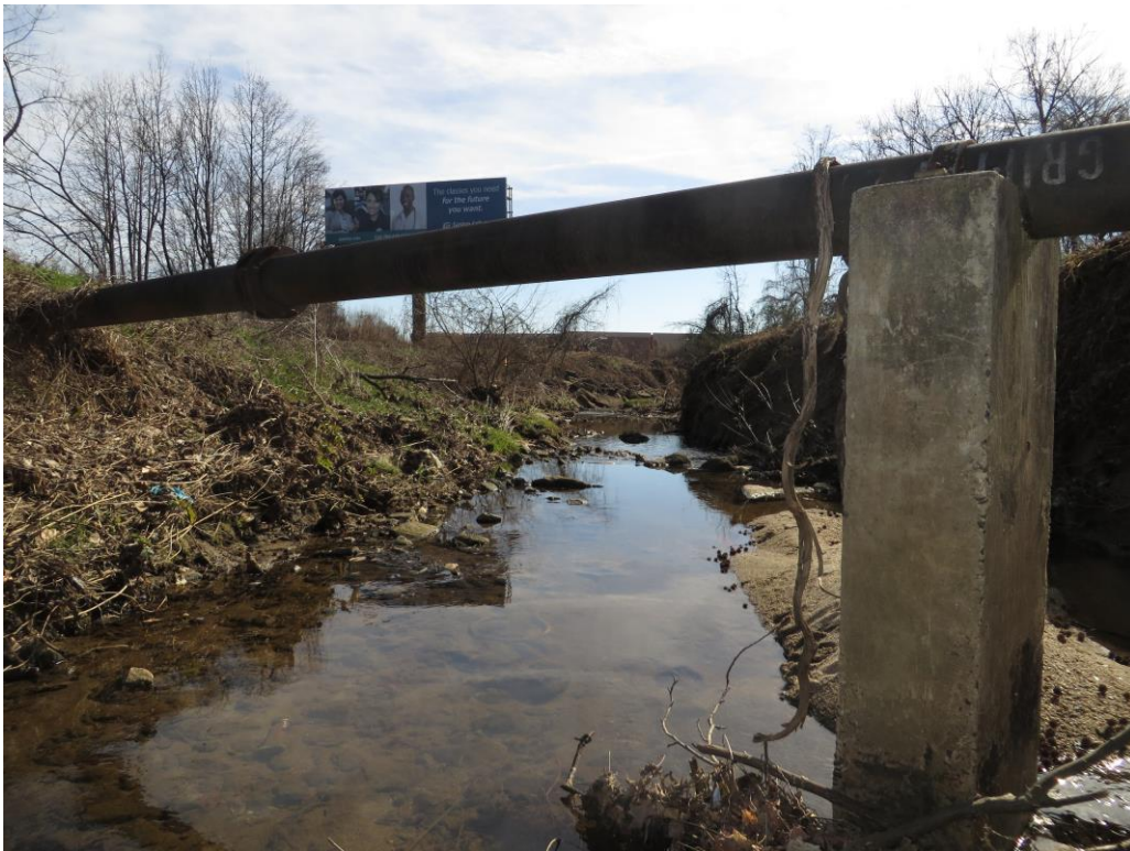
Looking Downstream from RCBC Outlet
