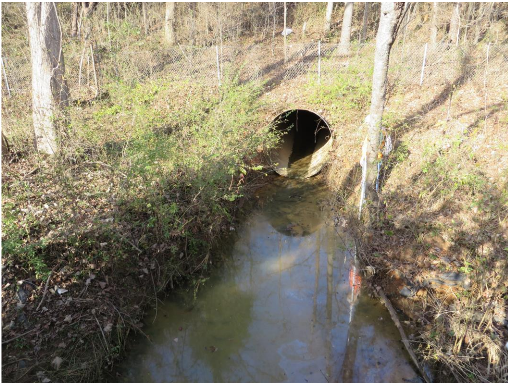
Looking Upstream from RCP Inlet
