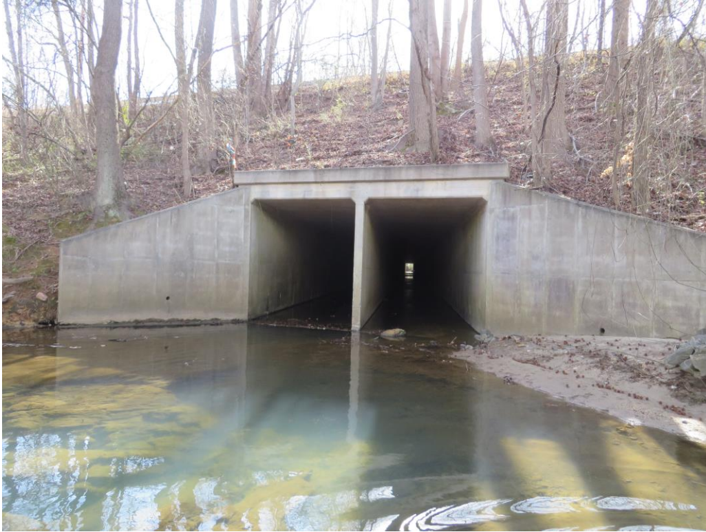
Looking at Upstream Face of 2 @ 8' x 9' RCBC
