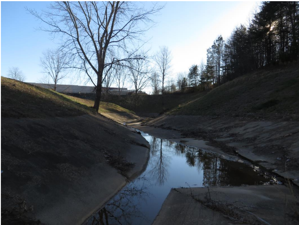
Paved Ditch Downstream of RCBC
