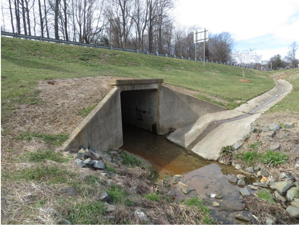
Looking at Downstream Face of 1 @ 8' x 9' RCBC
