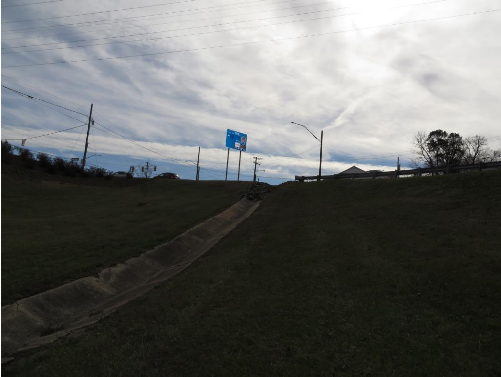
Paved Ditch at Upstream Right
