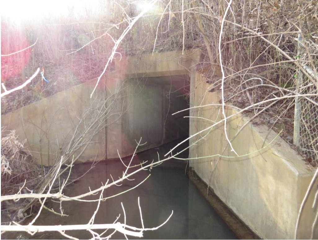
Looking at Upstream Face of 1 @ 7' x 8' RCBC
