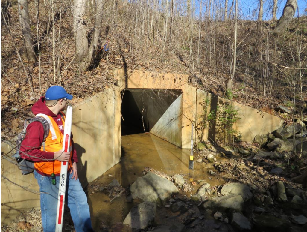
Looking at Downstream Face of 1 @ 8' x 8' RCBC
