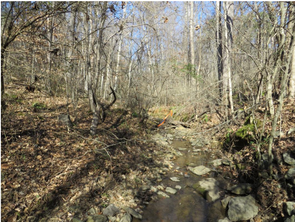
Looking Upstream from RCBC Inlet
