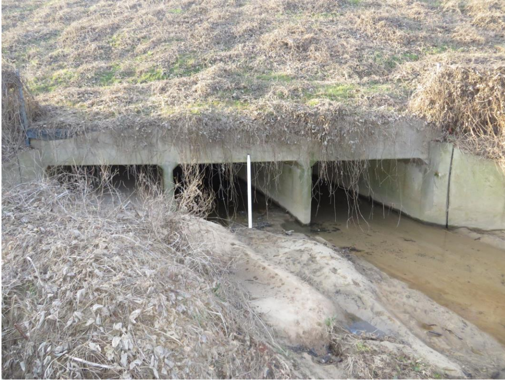
Looking at Downstream Face of 1 @ 7' x 9', 2 @ 8' x 9' RCBC
