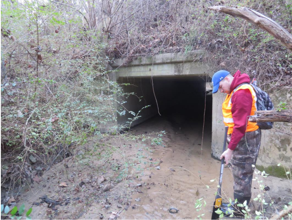
Looking at Downstream Face of 1 @ 9' x 9' RCBC
