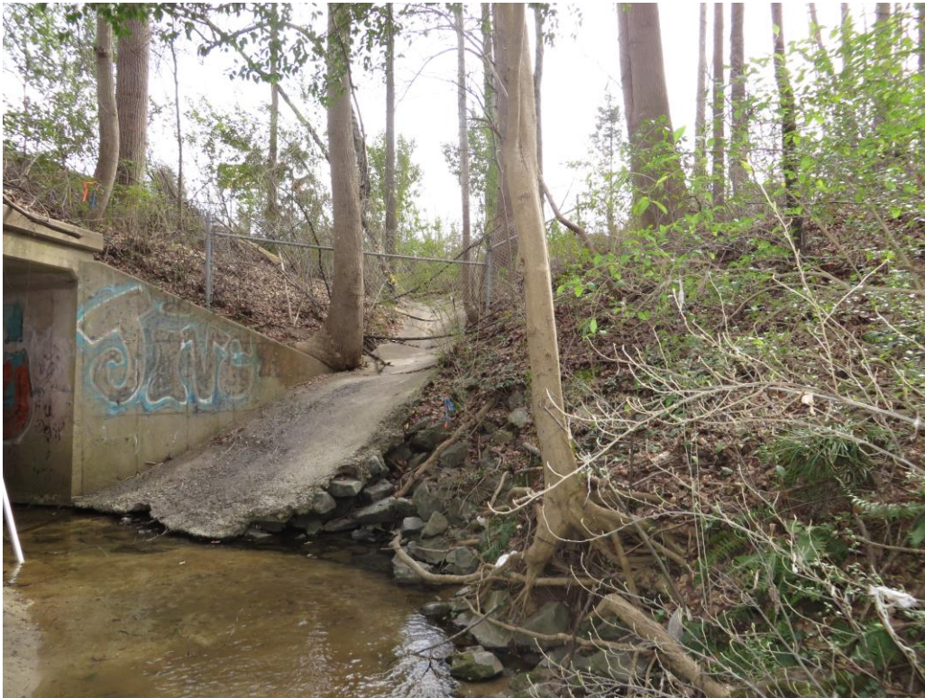
Paved Ditch at Upstream Right
