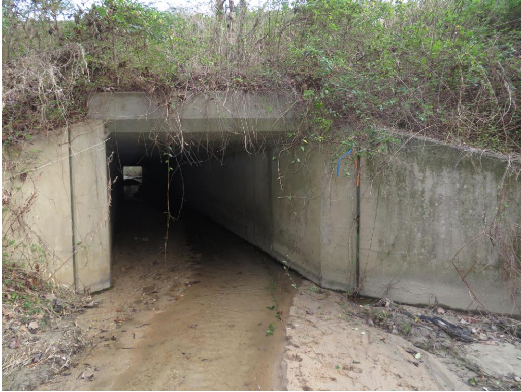
Looking at Upstream Face of 1 @ 9' x 9' RCBC
