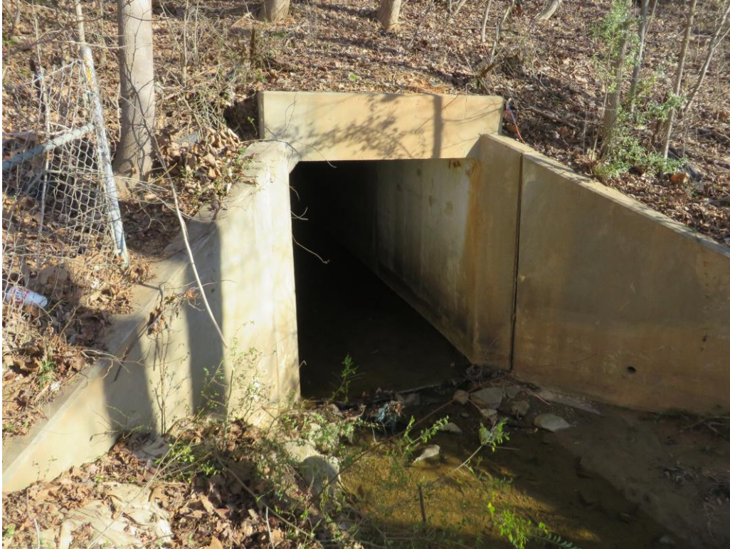
Looking at Downstream Face of 1 @ 7' x 8' RCBC
