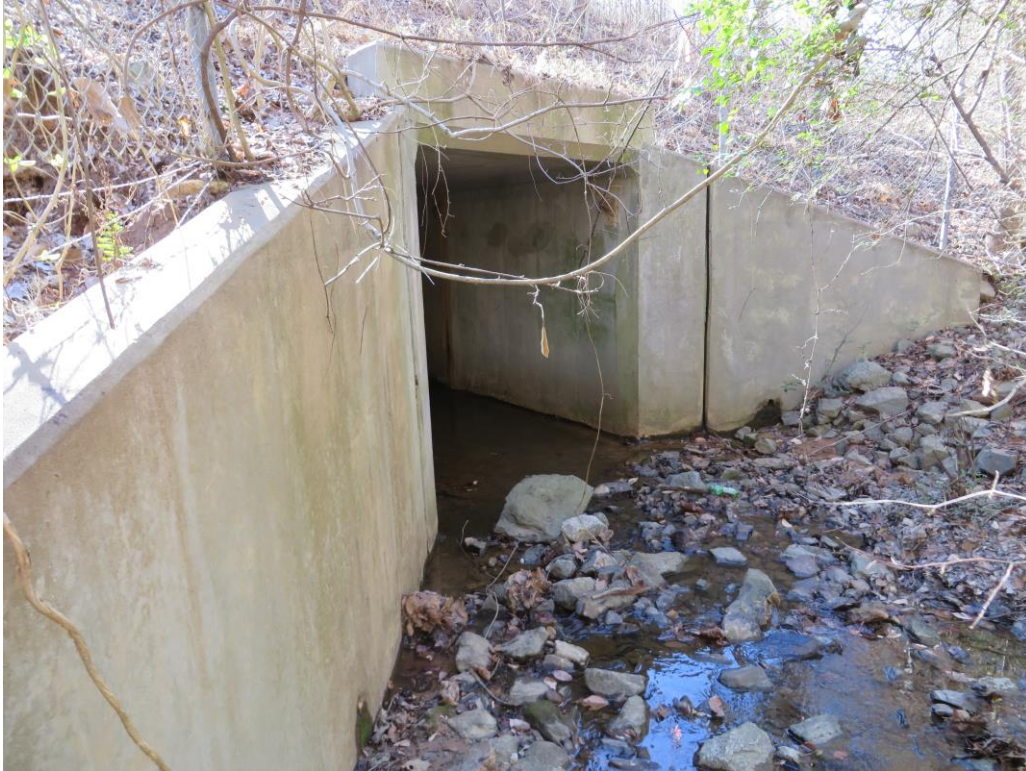
Looking at Upstream Face of 1 @ 8' x 8' RCBC
