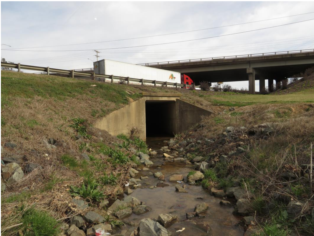
Looking Downstream from RCBC Outlet
