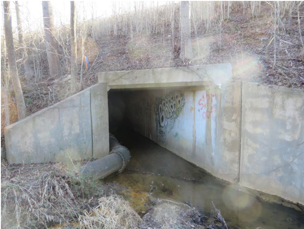
Looking at Upstream Face of 1 @ 8' x 8' RCBC
