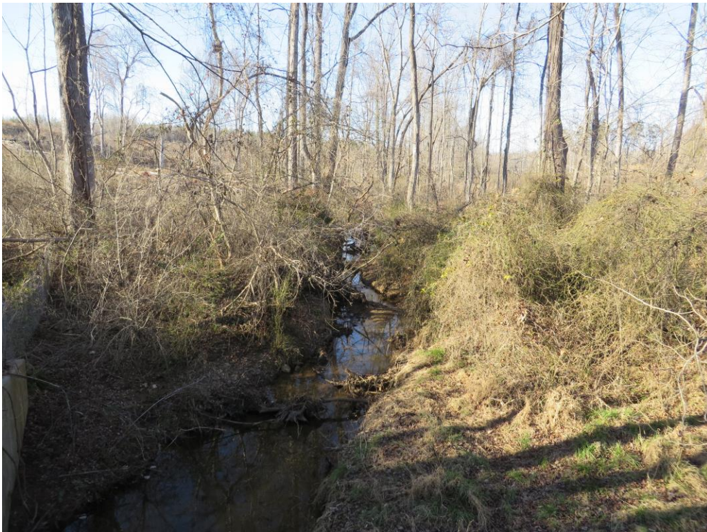
Looking Upstream from RCBC Inlet
