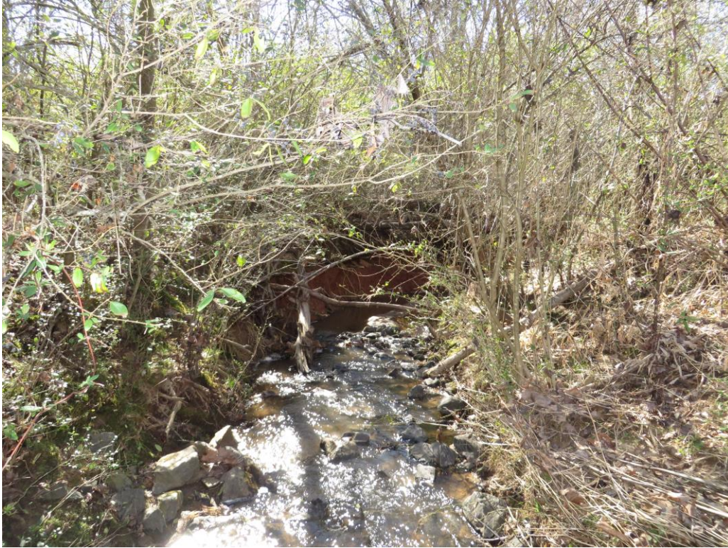
Looking Downstream from RCBC Outlet
