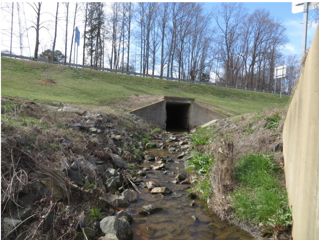
Looking Upstream from RCBC Inlet
