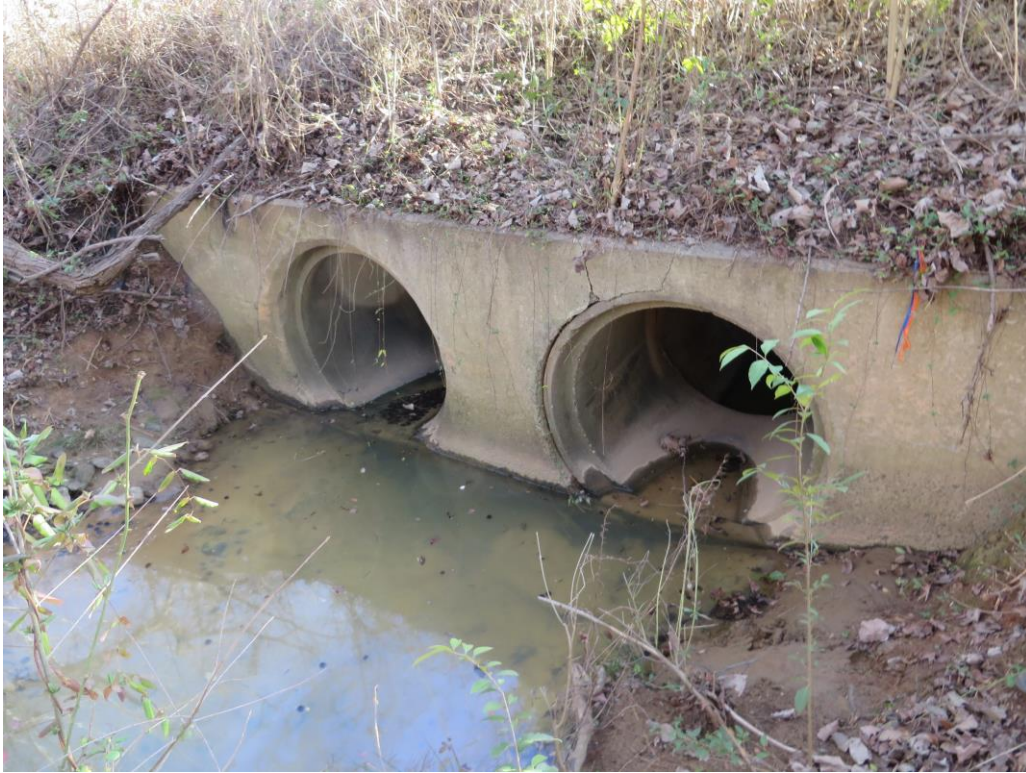
Looking at Upstream Face of 2 @ 54" RCP
