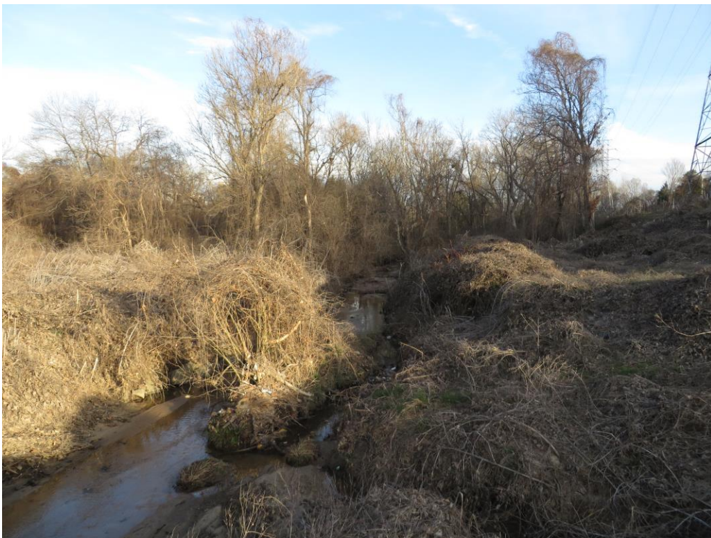
Looking Downstream from RCBC Outlet
