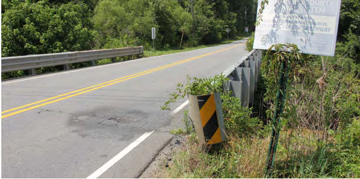
Existing Bridge on Back Creek Church Road
