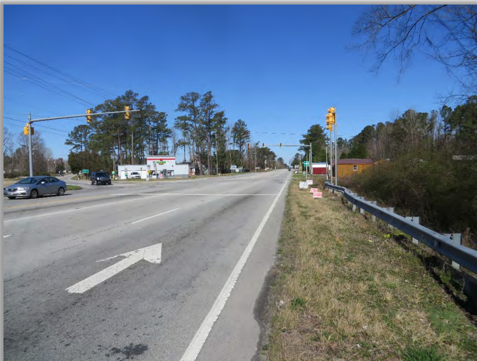
Looking Northwest along US 258 (Richlands Hwy.) Downstream - Left / Upstream - Right
