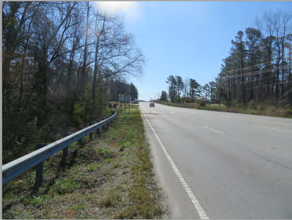
Looking Southeast along US 258 (Richlands Hwy.) Upstream - Left / Downstream - Right
